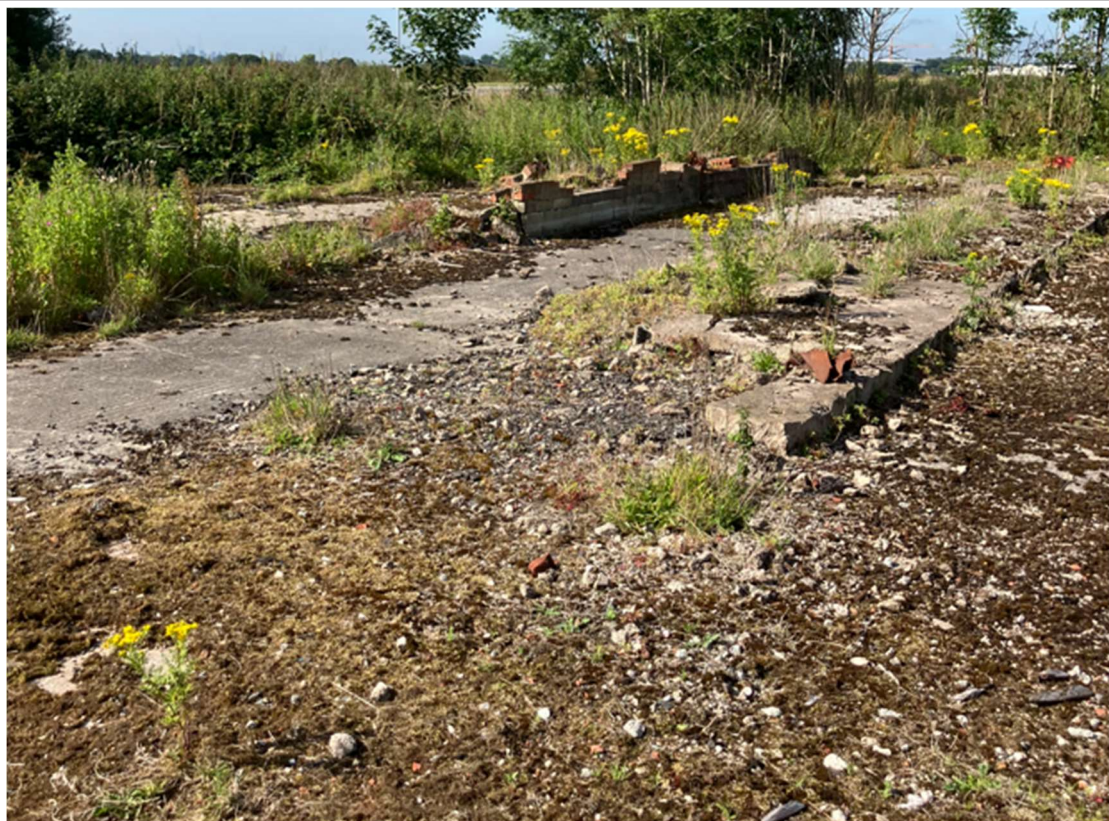
PLATE 4 – REMNANT SLABS AND WALLS AT FORMER HARES HILL FARM
