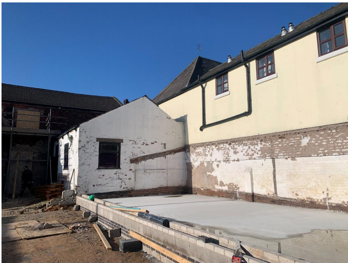
Plate 4: View of buildings on site.
