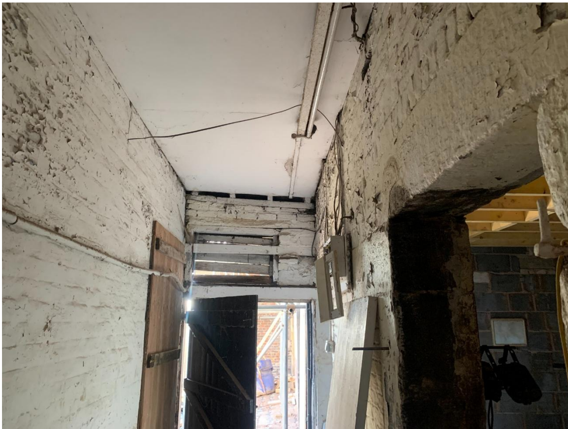
Plate 20: Internal view of structure.
