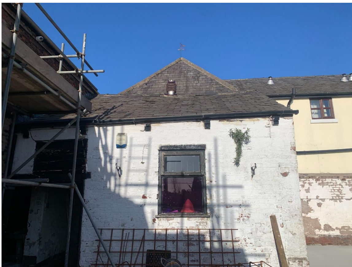
Plate 6: View of buildings on site.
