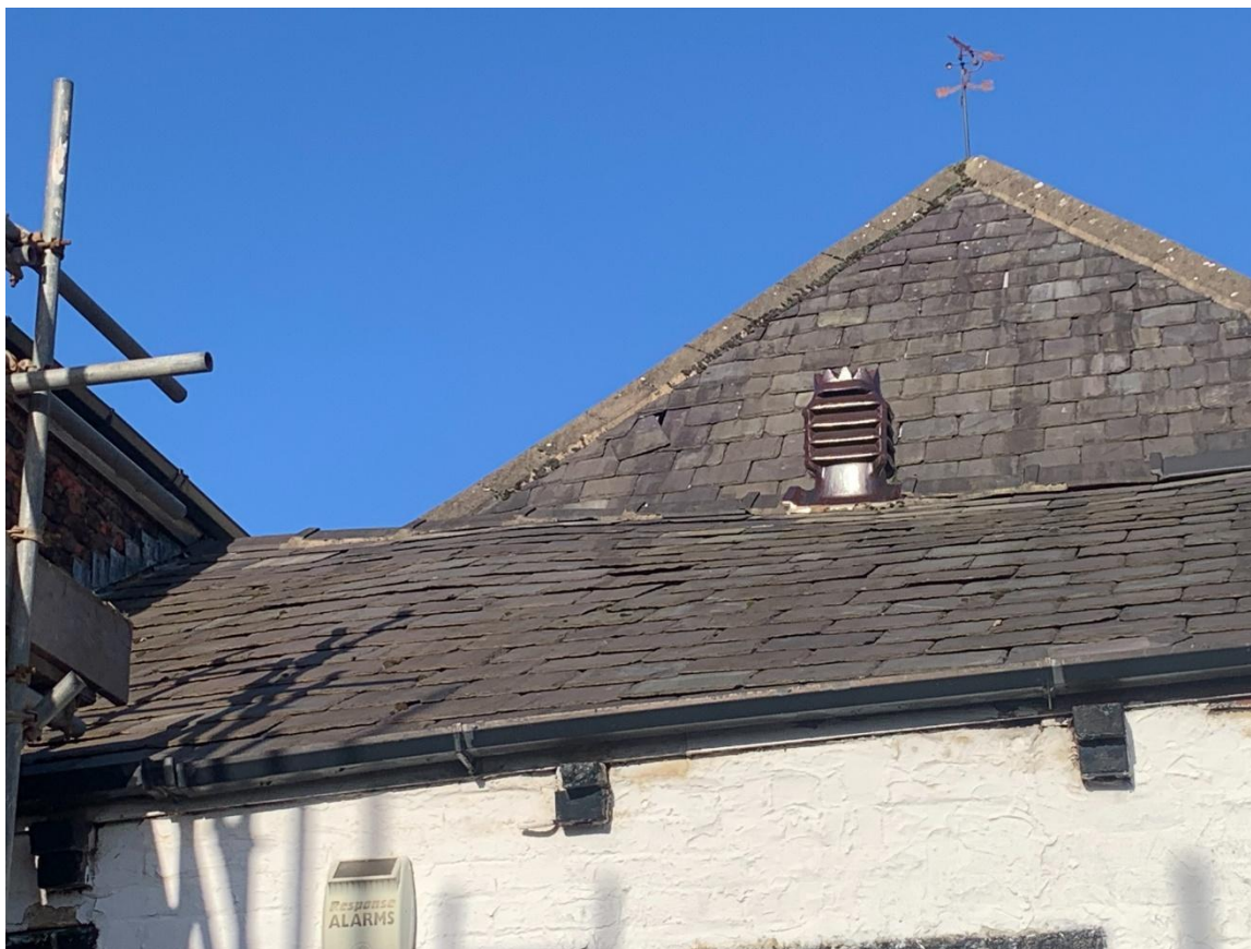
Plate 7: Close-up of roof tiles.
