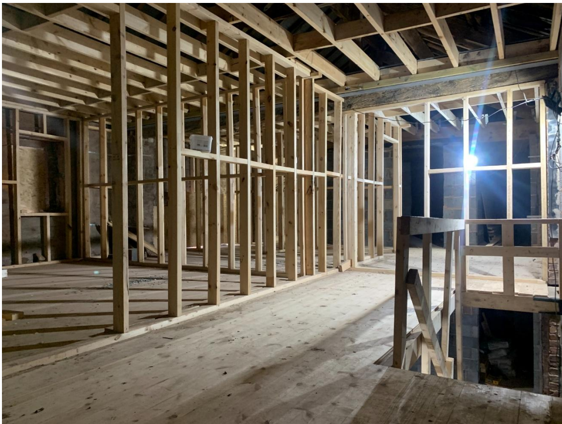
Plate 12: Internal view of structure.
