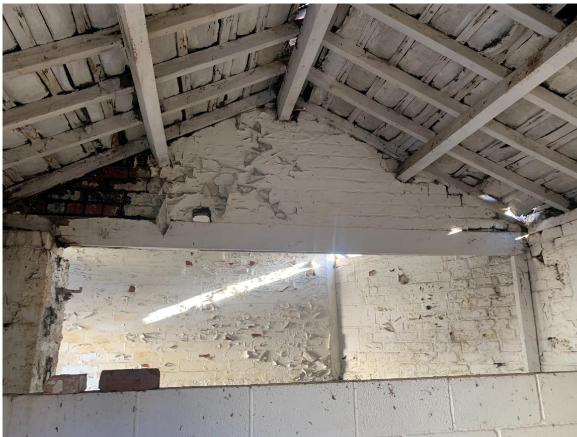
Plate 23: Internal view of structure.
