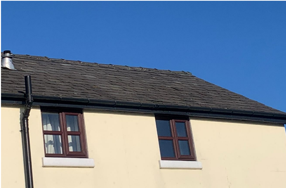
Plate 9: Close-up of roof tiles.
