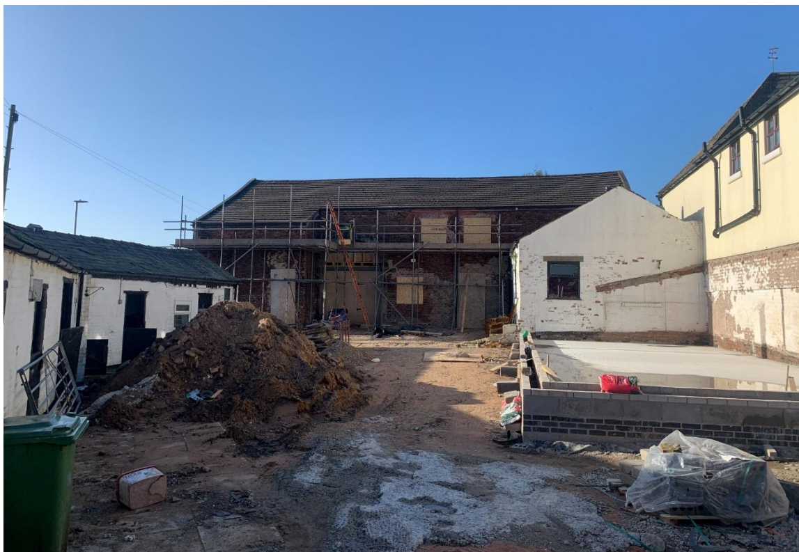
Plate 3: View of hardstanding areas.
