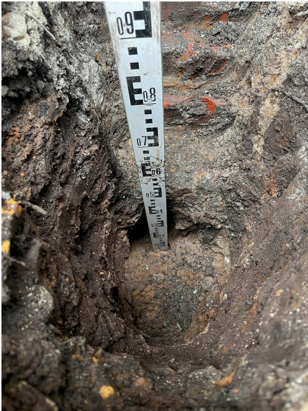
Plate 3 - HP01 possible concrete footing at a depth of 0.85mbgl. Projects 270mm. Underside proven.
