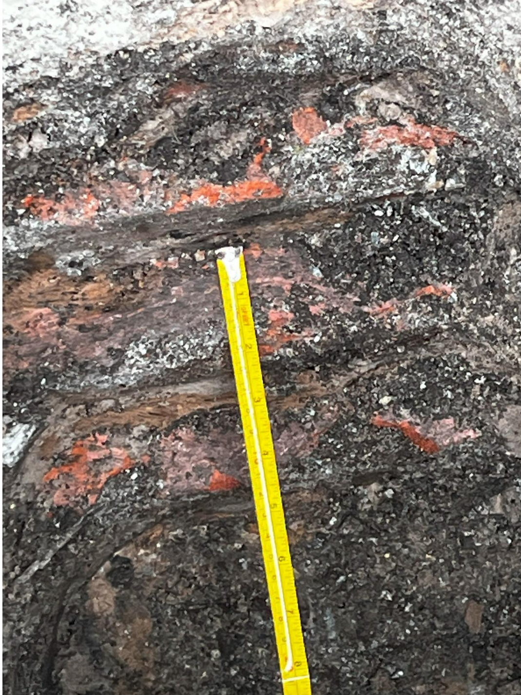
Plate 4 - HP01 brick foundation at a depth of 0.55mbgl, projects 0.120mm away from brick wall.
