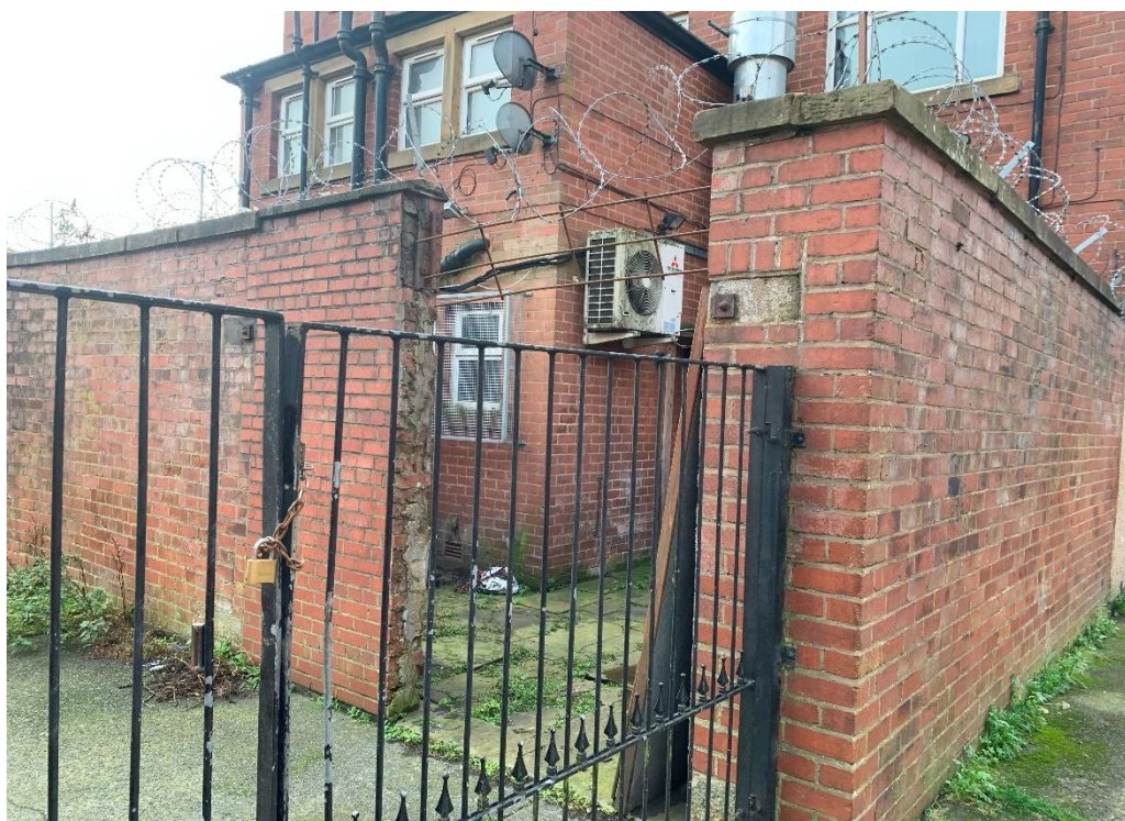
Plate 8 – Gated entrance to courtyard in the north of site, looking southeast.
