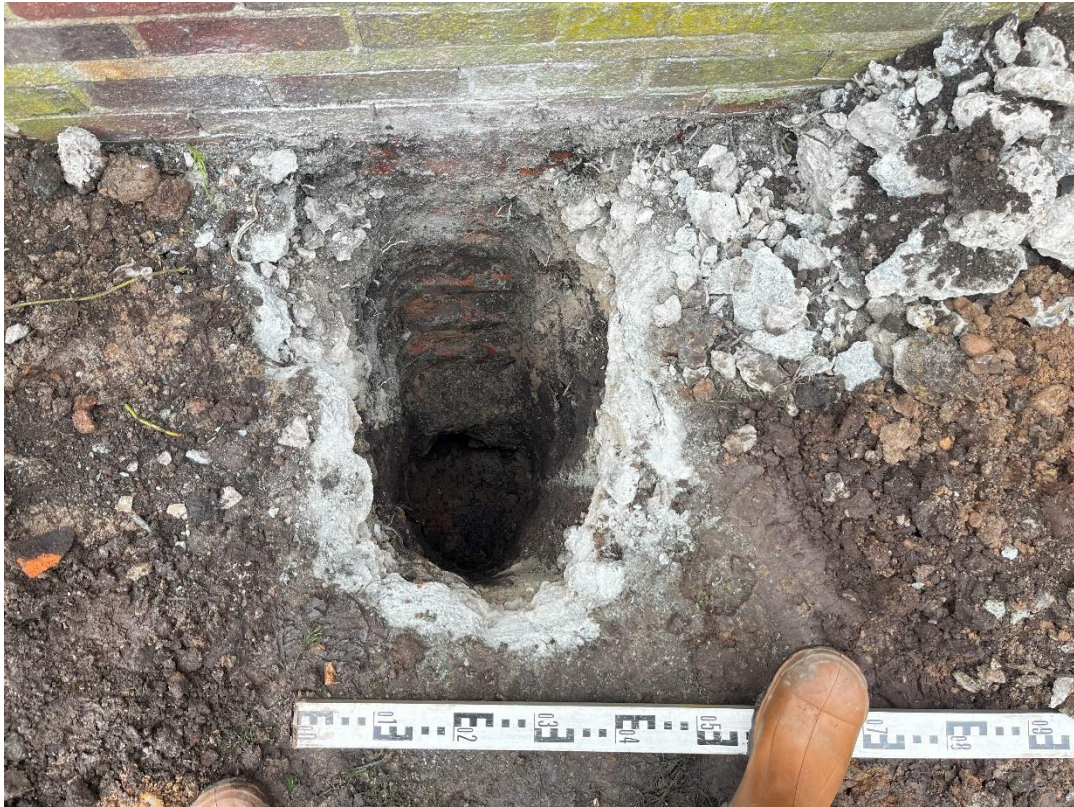
Plate 1 - Hand pit 01 (HP01) arisings ground level to 1.3mbgl.
