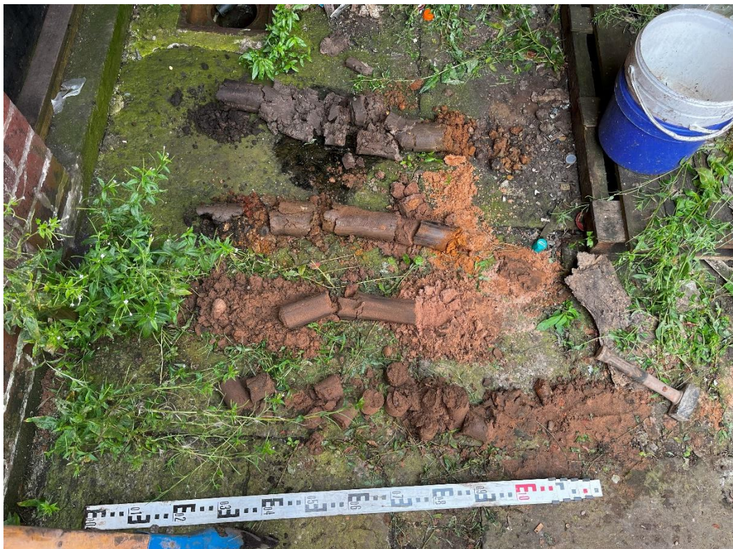
Plate 2 – WS01, 1.20m bgl and 5.00m bgl.
