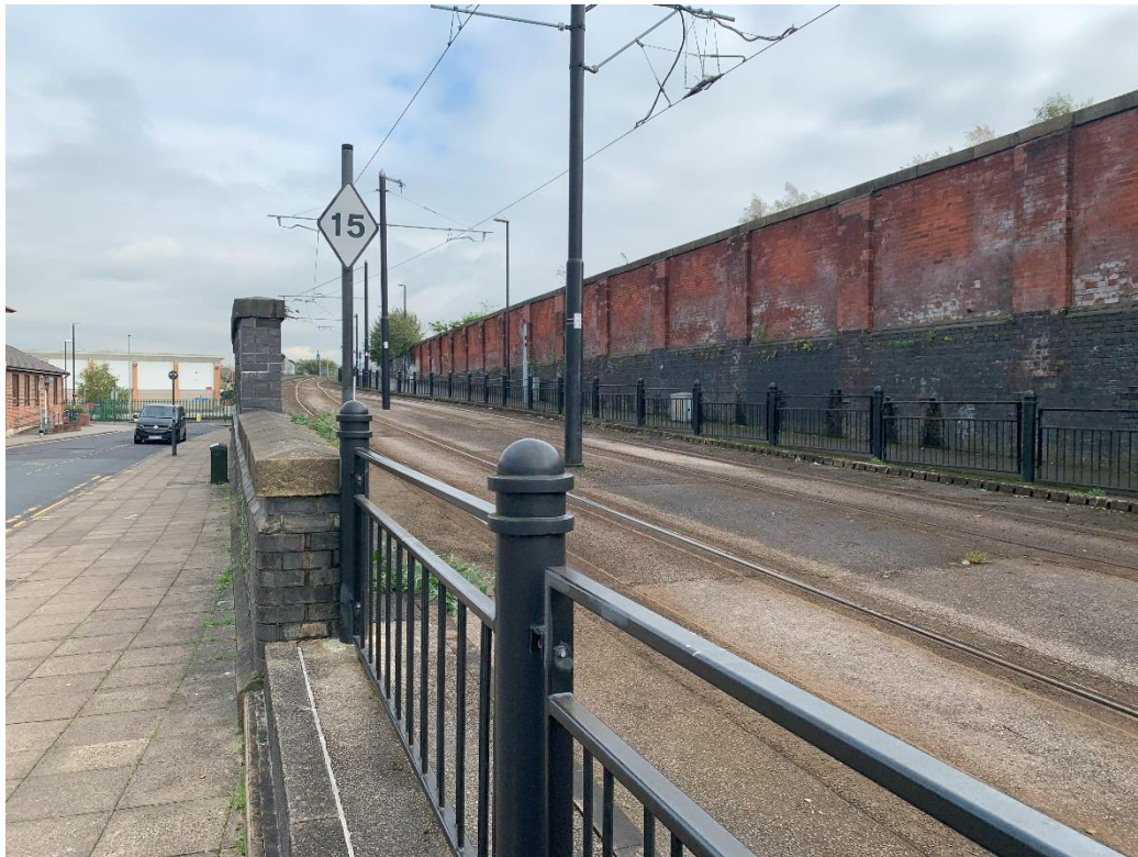
Plate 6 – Station Road (left) and High Level Road (right), the sites southern boundary, looking east.
