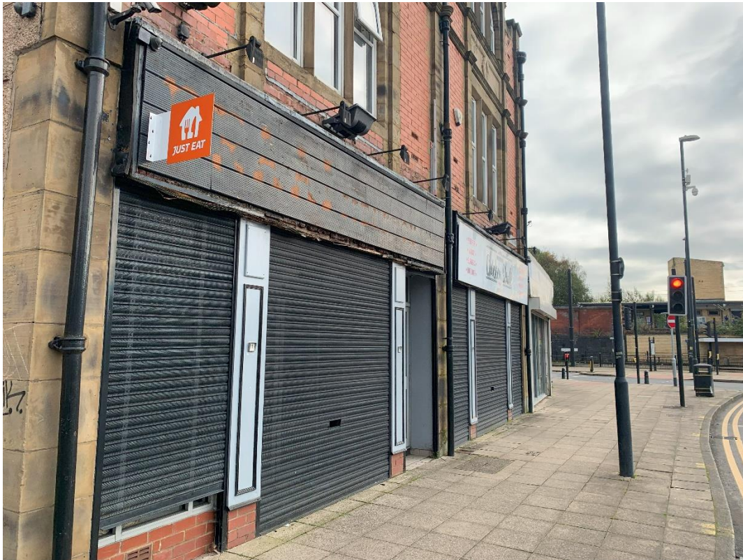
Plate 3 – 3-storey building present on site, looking south.
