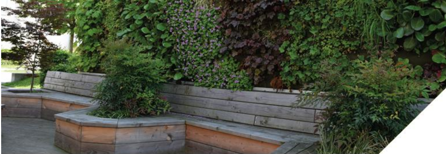
A two-dimensional system is installed on an ETICS rendered façade in Freiburg's Turmcafé.
