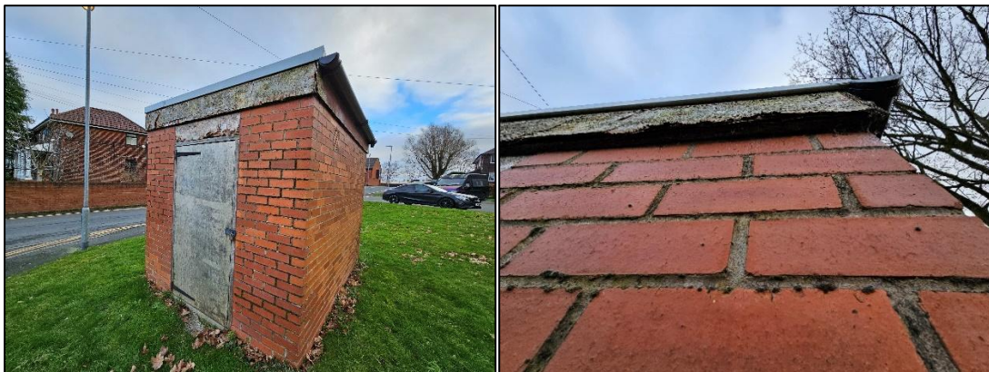
Photographs 5 (left) and 6 (right) showing the substation building and the gap between the wall and the barge board, respectively.
