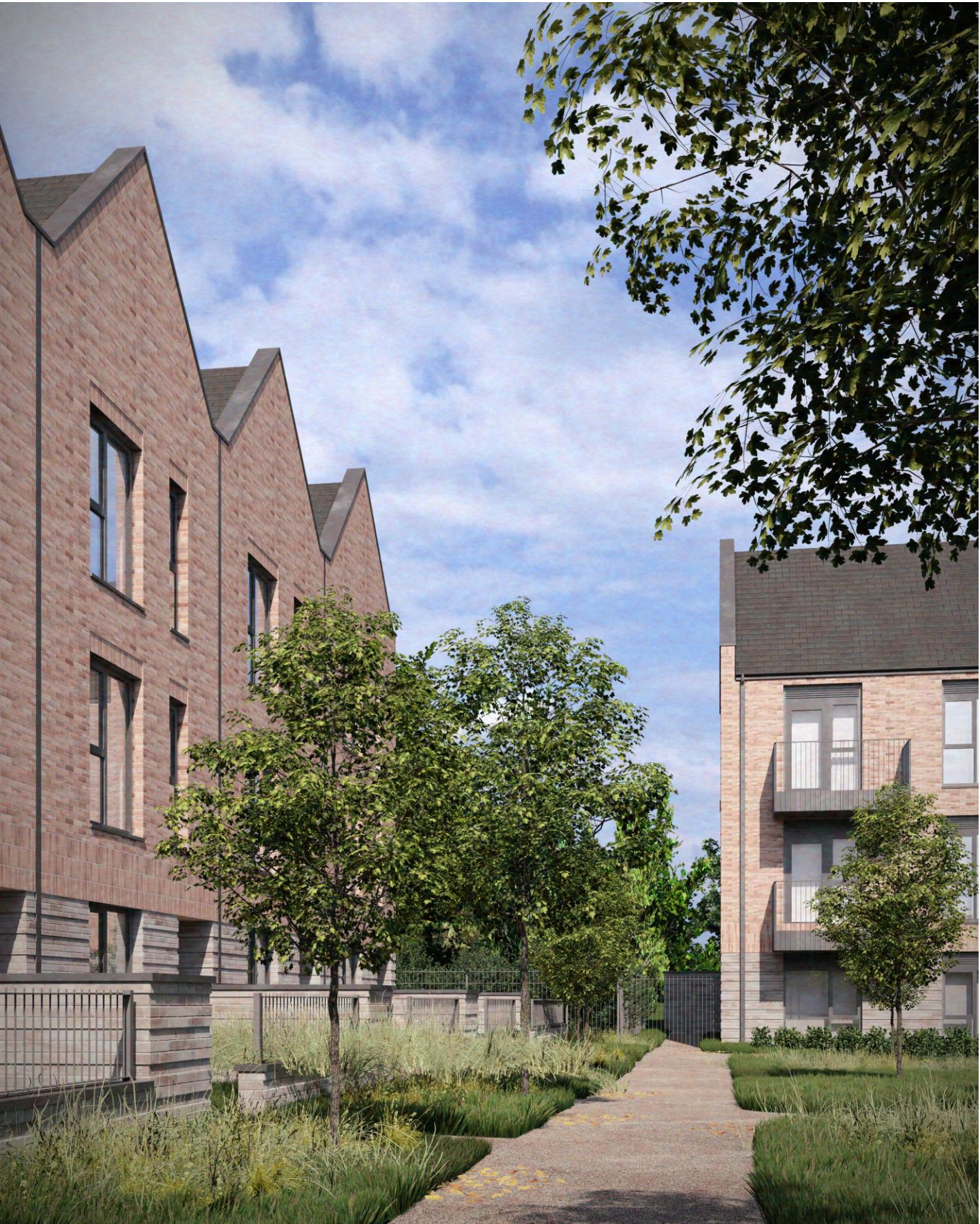
View of the proposed development – looking south-west in front of the dwelling block
