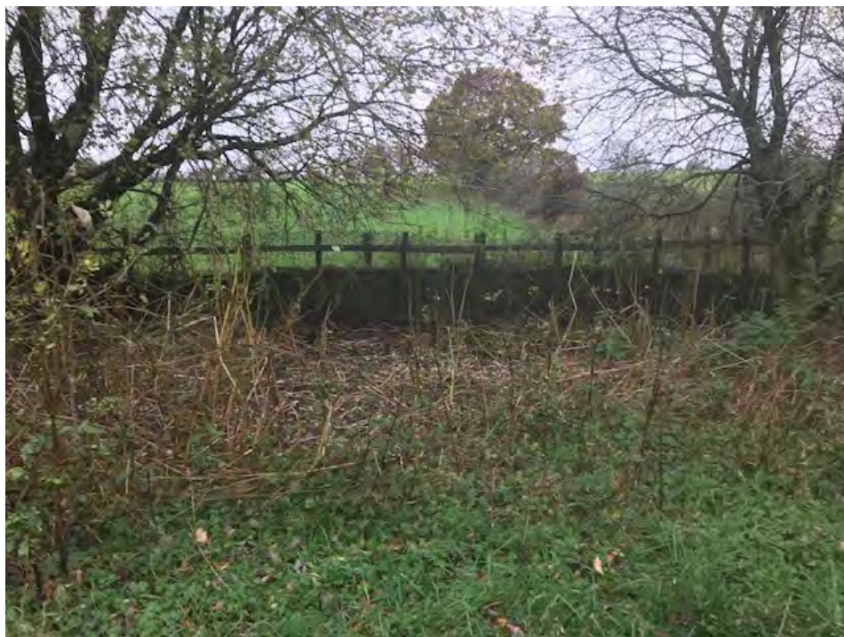
Photograph 10: View of the stone boundary wall along the south-west boundary of the Site, looking SW
