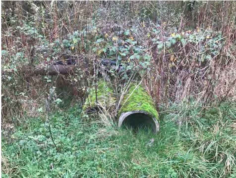
Photograph 12: A dump of disused service pipes in the north-west corner of the Site, indicating that some excavation work has been carried out
