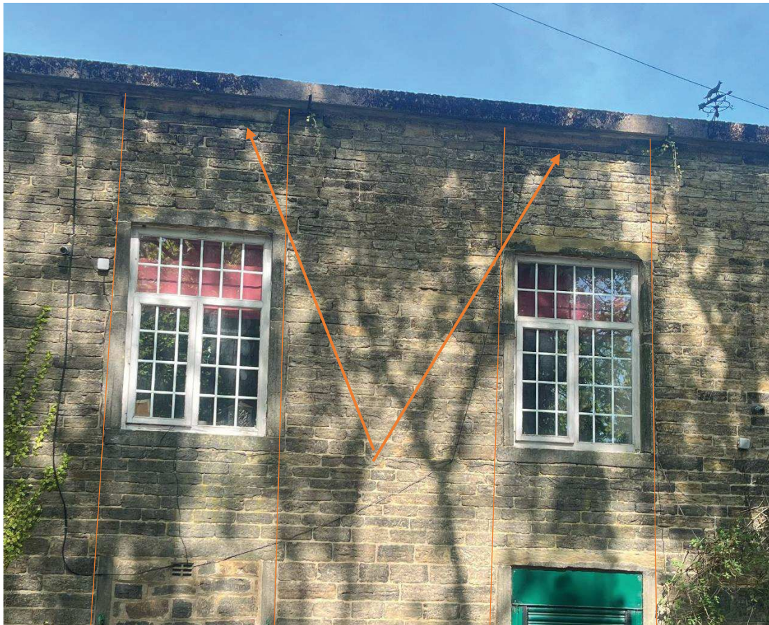
Figure 3.3 The front façade, note the arrangement of the window bays, the concrete copings and the possible window cills at eaves level. The window cills are also visible on the side elevation in similar bays.
