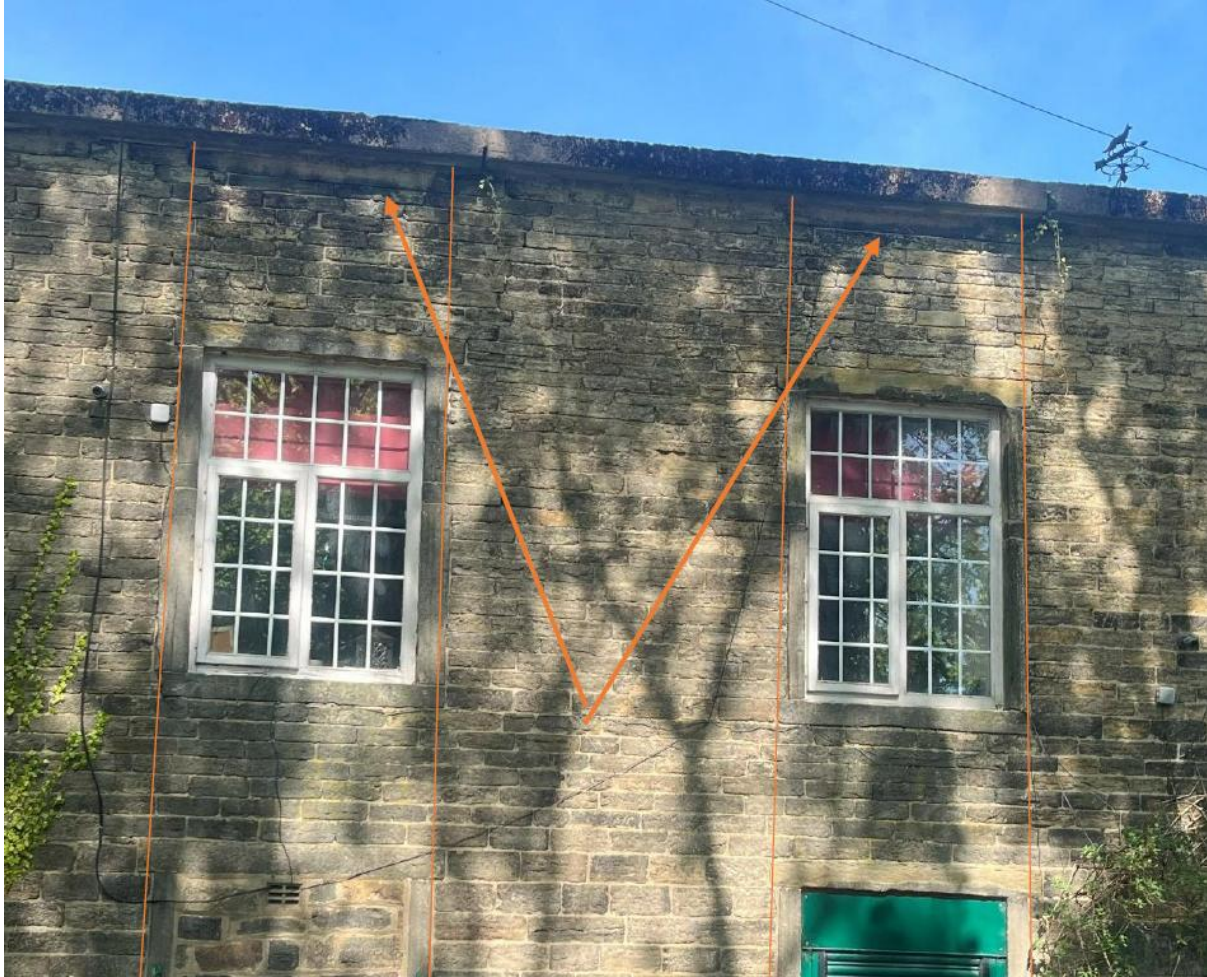
Fig 4: The front façade, note the arrangement of the window bays, the concrete copings and the possible window cills at eaves level. The window cills are also visible on the side elevation in similar bays
