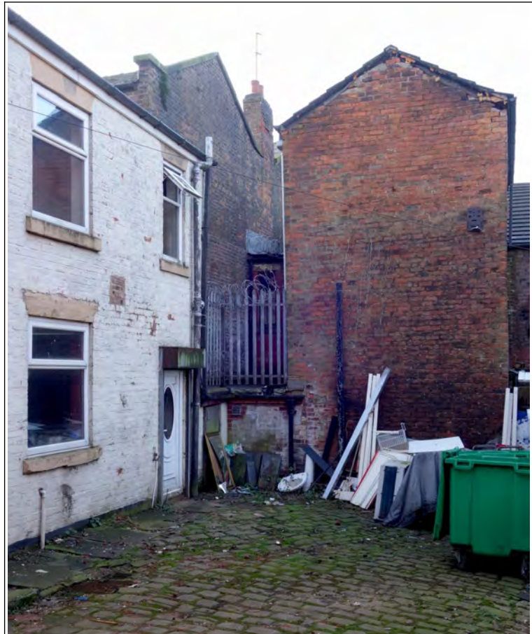
Photo 10: South-west end of courtyard (rear of Oldham Road properties to right)
