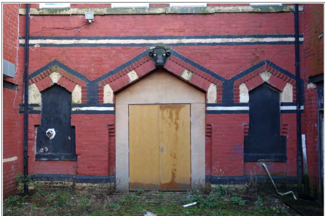
Photo 5: Ground floor openings, courtyard elevation
