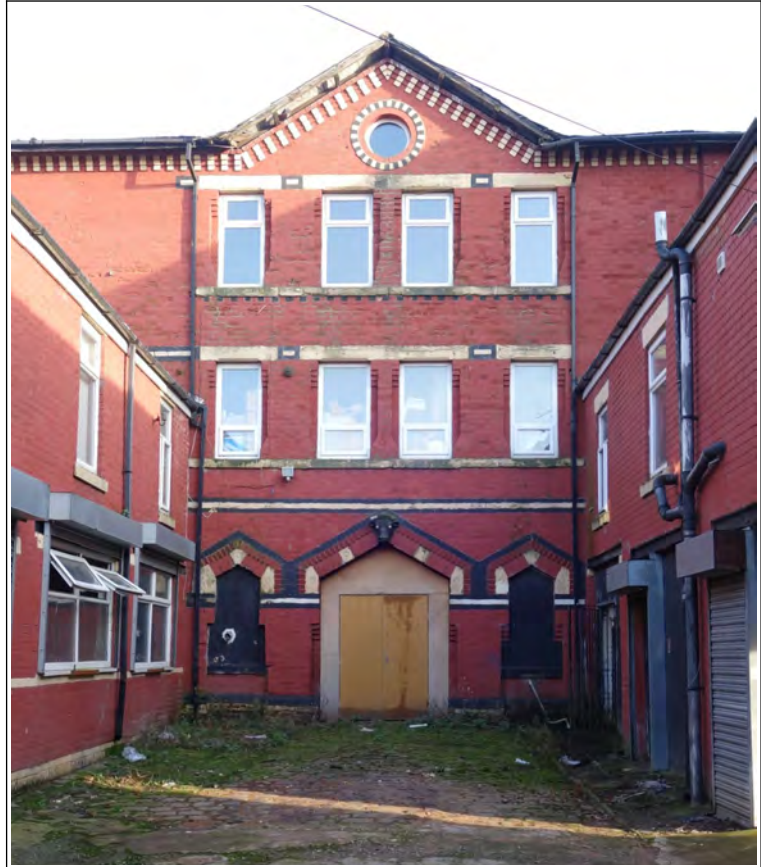
Photo 4: Courtyard elevation of main block
