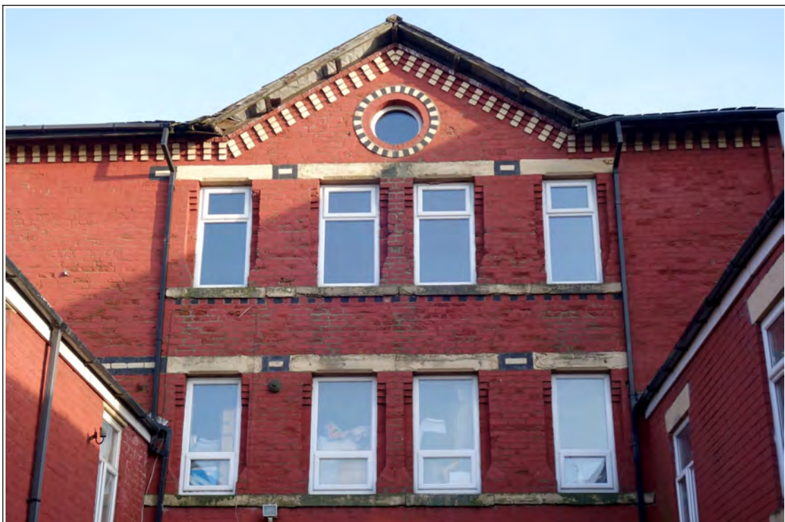
Photo 7: Upper floor details, courtyard elevation
