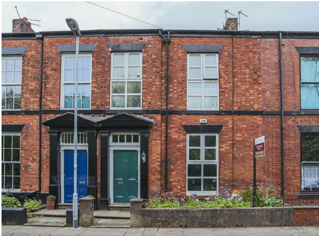
Figure 1 – Front elevation, 14 St James Terrace, Heywood
