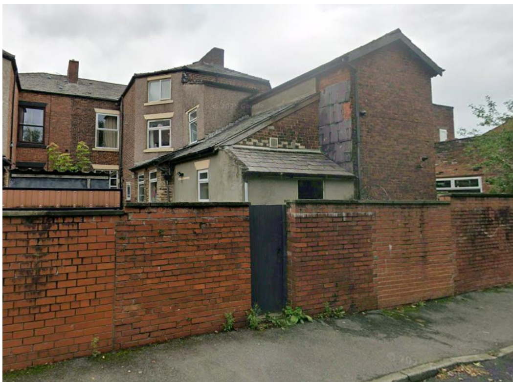
Figure 2 – Rear elevation, view from Cartridge Street
