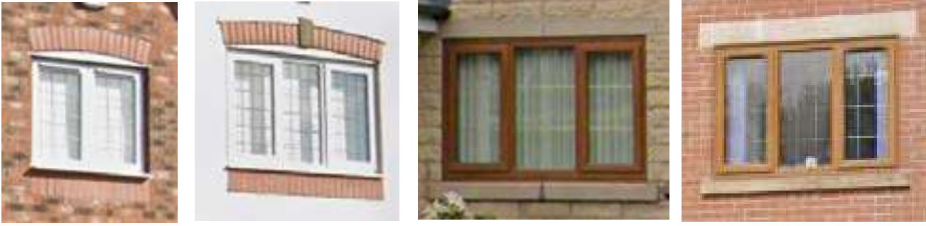
Window heads and cill details vary from red soldier bricks to stone in different heights, widths and styles, whether it be arched or linear.
