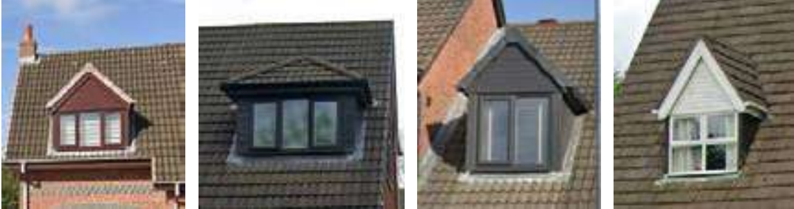
Dormer windows of different widths and height are another common vernacular detail seen within the local surroundings.
