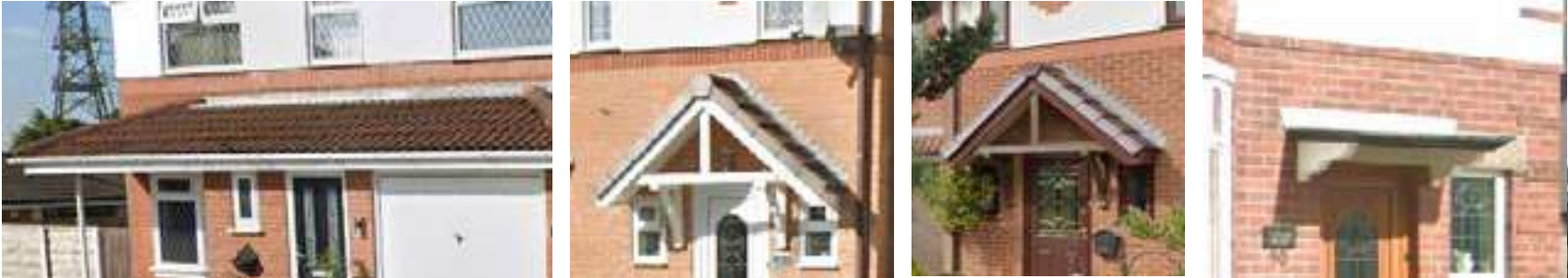
Entrance canopies vary from flat hung to flat canopies or standalone protrusions.
