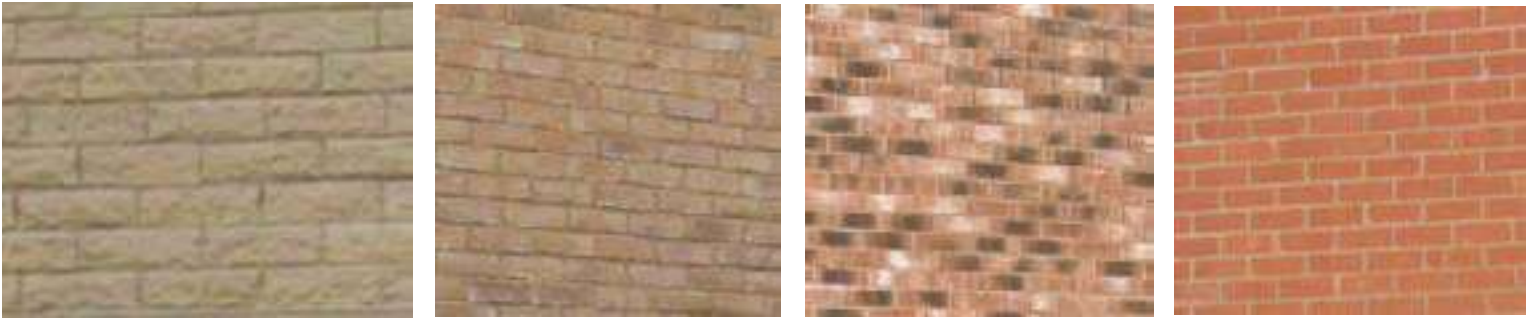
Houses are predominantly constructed from buff or red brick of varied tones with either grey or red roof tiles.
