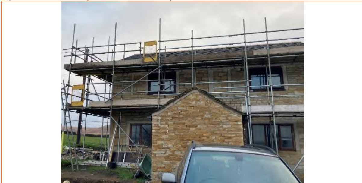
Figure 2 Showing B1's southwestern aspect
