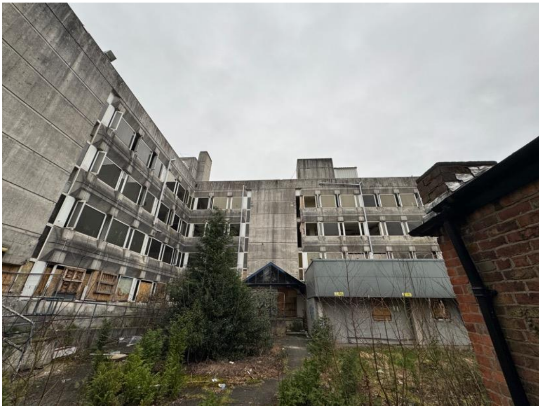
Image 25 – View of inner corner of building, looking at south elevation to left and west elevation to right of image. Restricted viewpoint due to Garden of Remembrance to immediate right.
