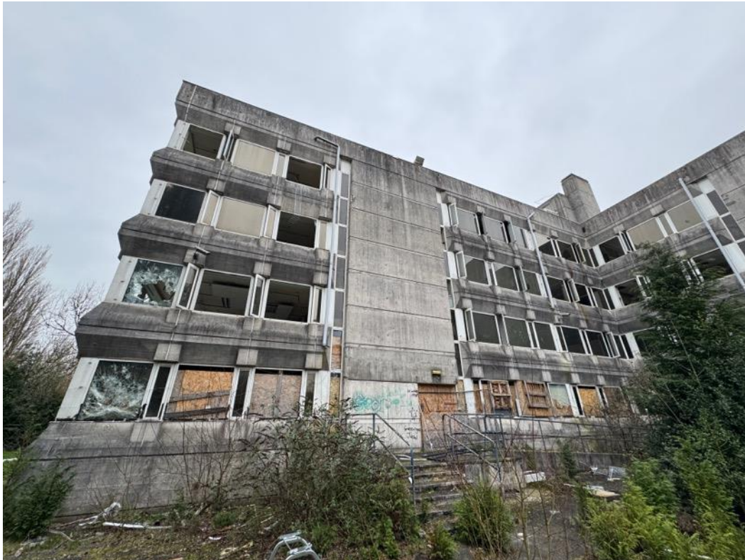
Image 24 – Overall view of south elevation left hand side. Photo taken from inner courtyard, access restricted by vegetation growth.
