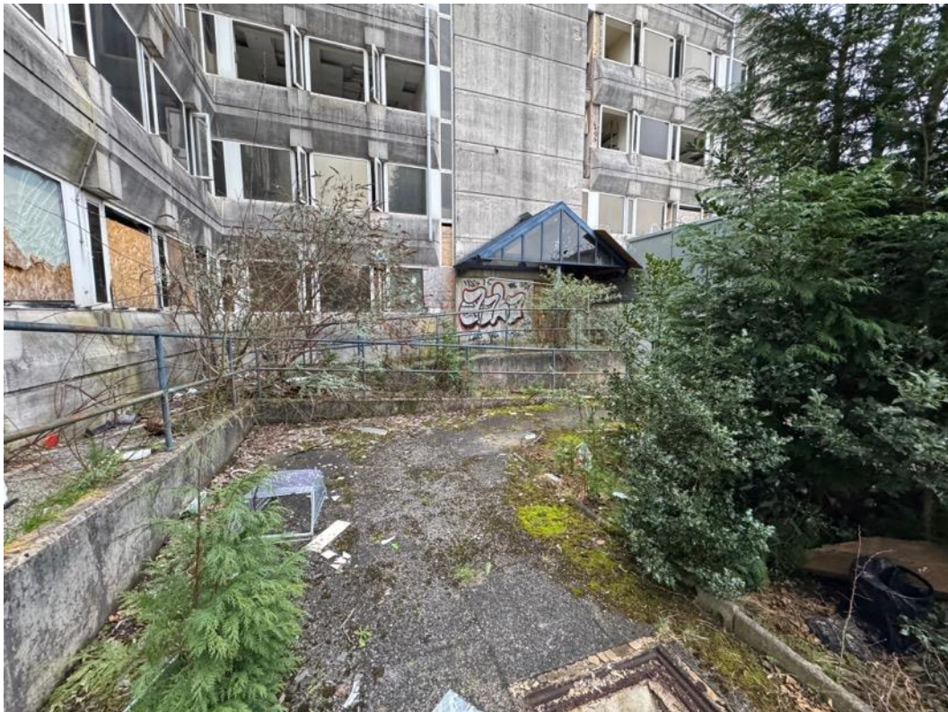
Image 27 – View of access/egress point to west elevation. Original concrete block canopy replaced by metal and glass canopy.
