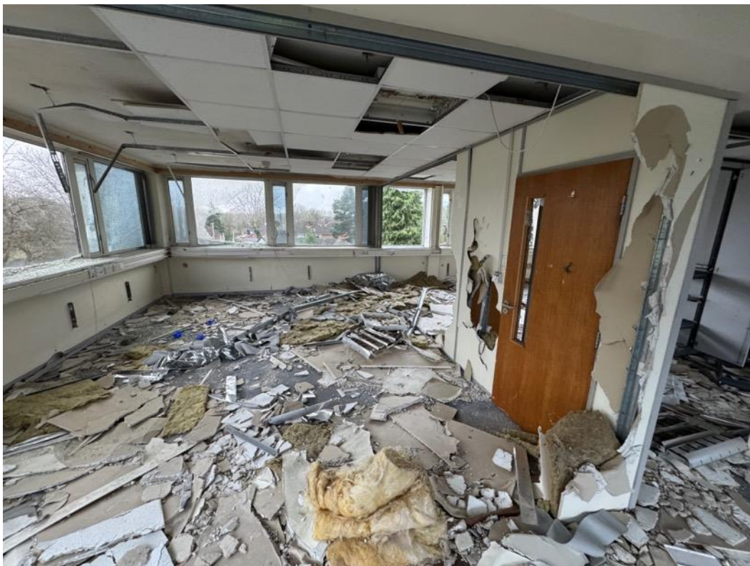
Image 95 – View of former enclosed offices to southern end, looking toward the west.
