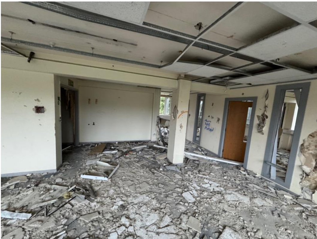
Image 79 – Second floor entrance from northern stairwell looking south.
