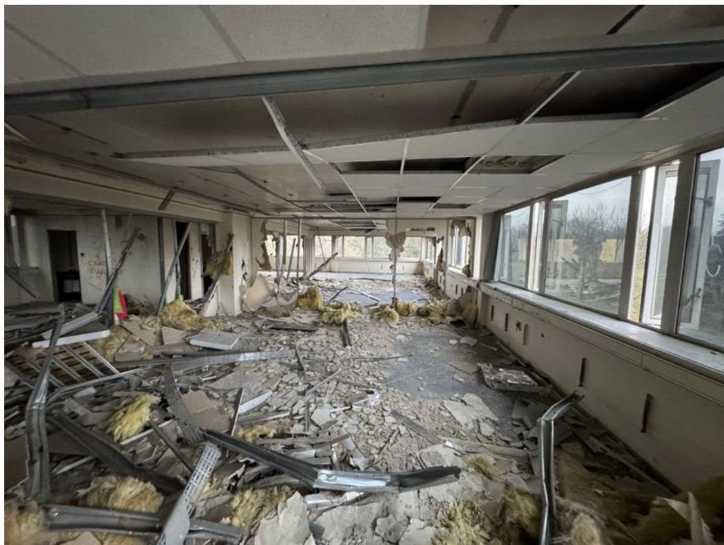
Image 107 – Southern end of third floor looking north.
