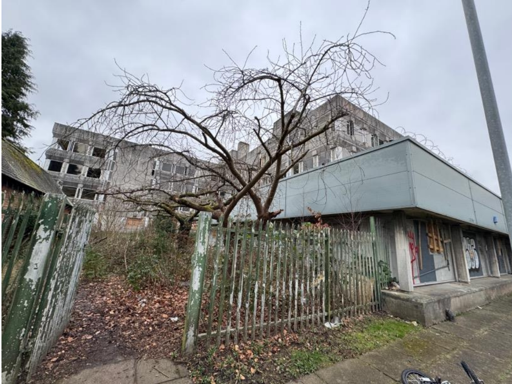
Image 32 – View of southwest corner of ground floor extension, with steel palisade fencing to inner courtyard area.
