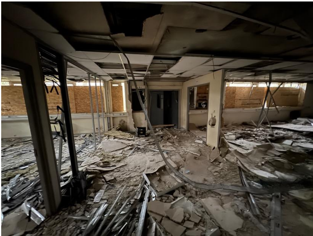
Image 57.- internal view of entrance point to north elevation, into ground floor north extension.
