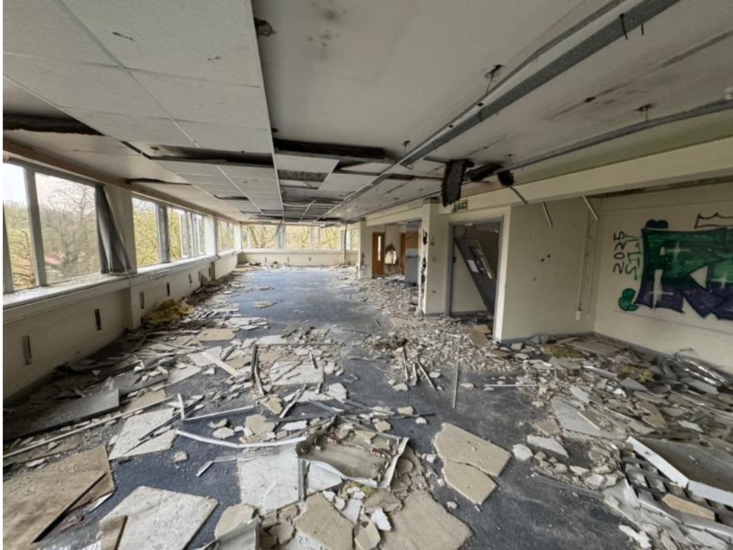
Image 92 – View of south side second floor, looking to southeast corner.
