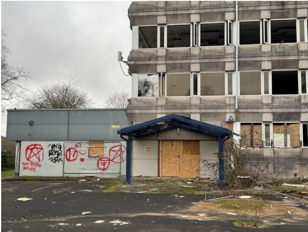
Image 8 – Closer view of main entrance point, with metal and glass canopy.
