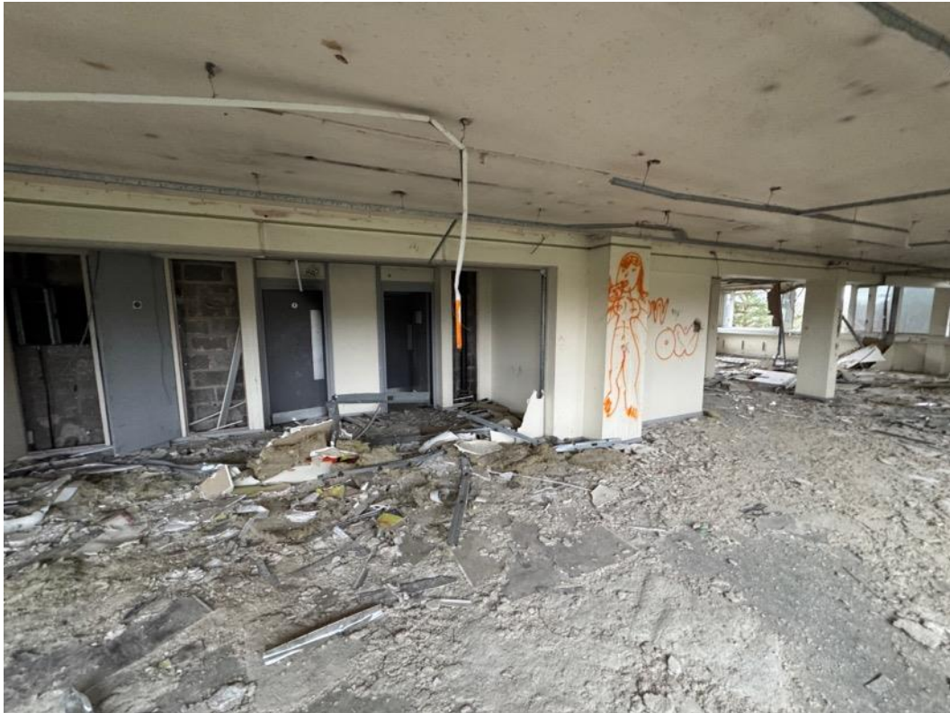
Image 102 – Third floor view toward toilet blocks at western end, looking south.
