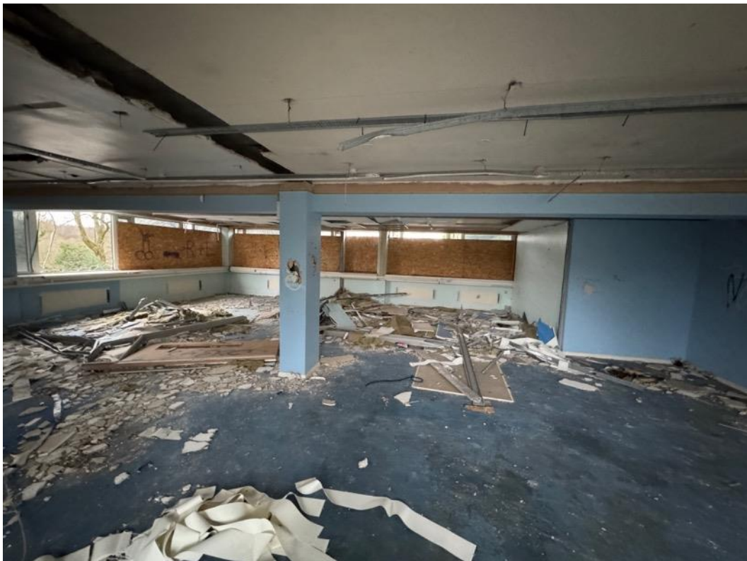
Image 75 – First floor view of southwest corner. Windows boarded above ground floor flat roof.
