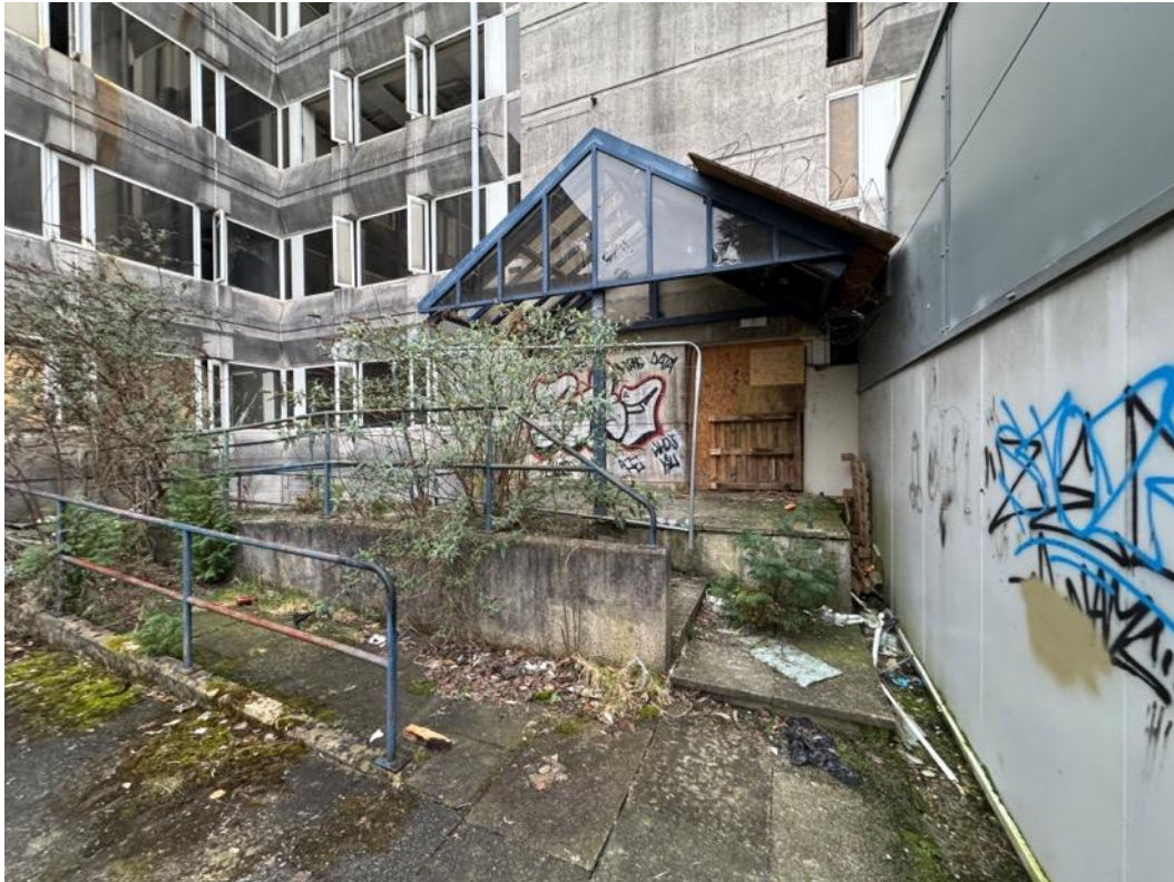
Image 28 – Closer view of entrance to west elevation, with ramped and stepped access.
