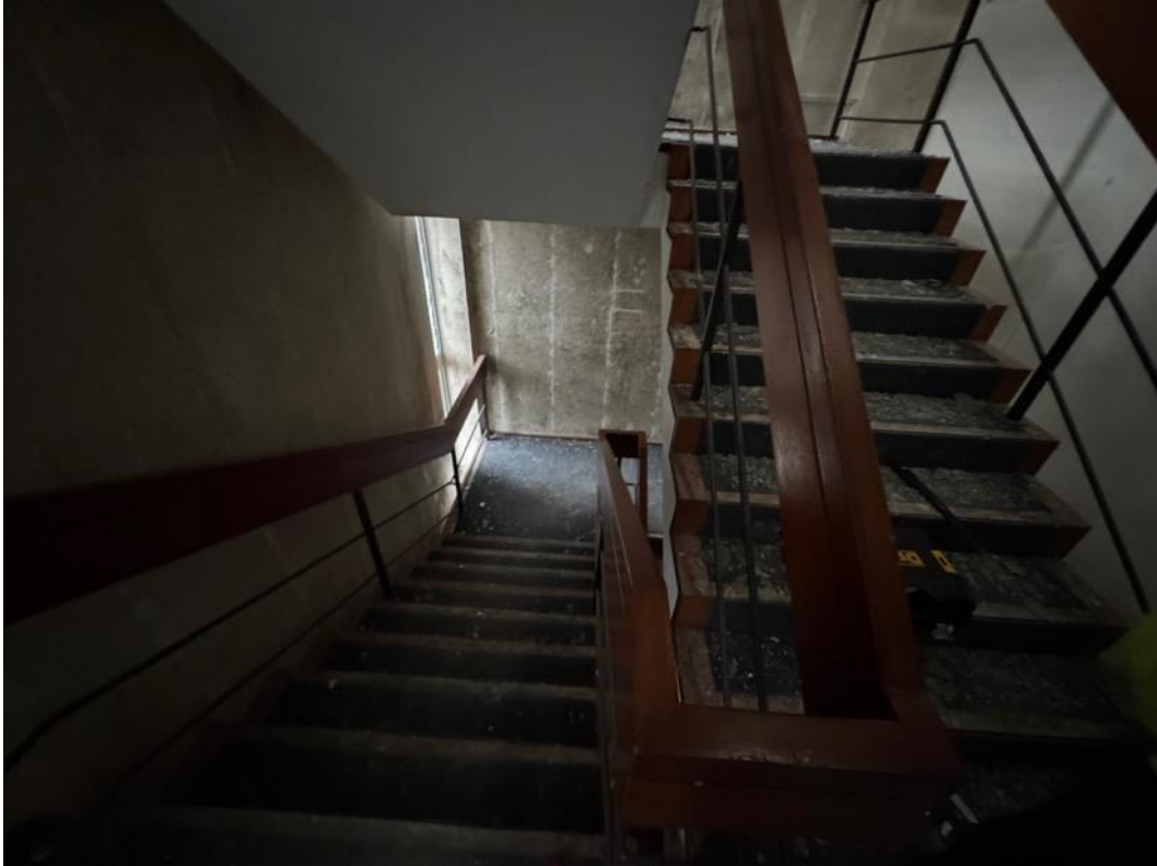
Image 78 – Second floor view into northern stairwell.
