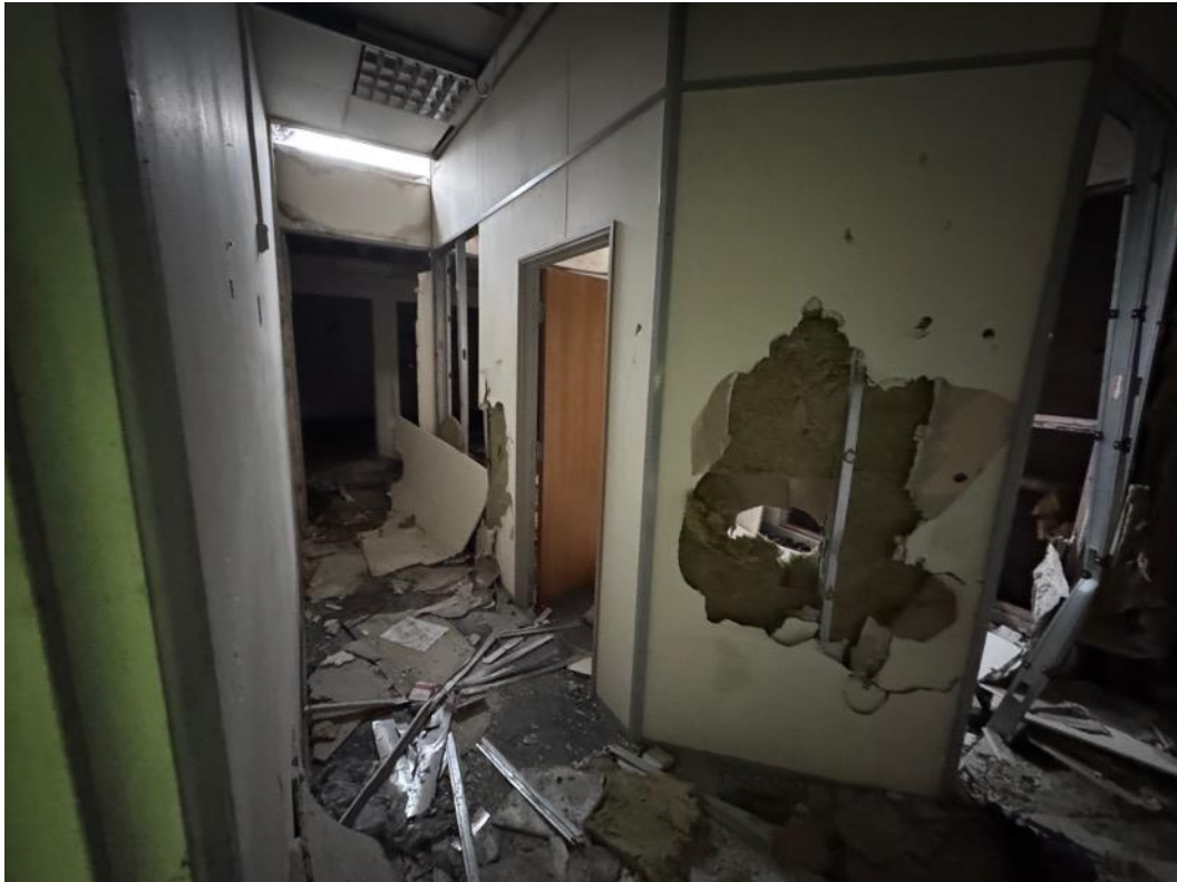
Image 46 – View of corridor area to west extension.
