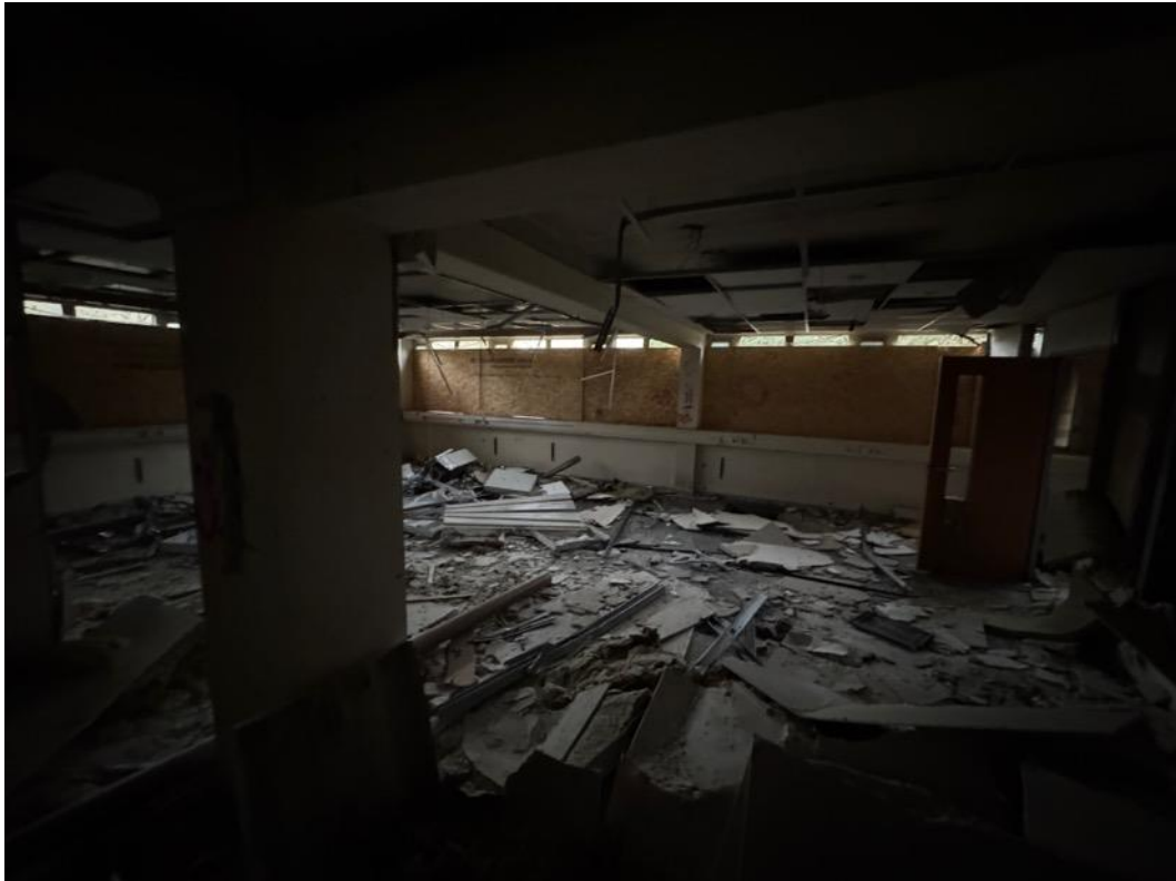
Image 54 – Internal view of northeast corner of ground floor.
