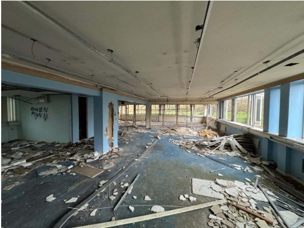
Image 72 – First floor internal view looking north.
