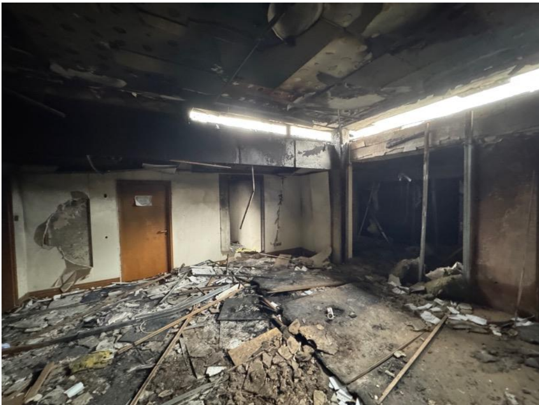
Image 43 – Internal view looking southwest. Clerestory windows above a notable feature.
