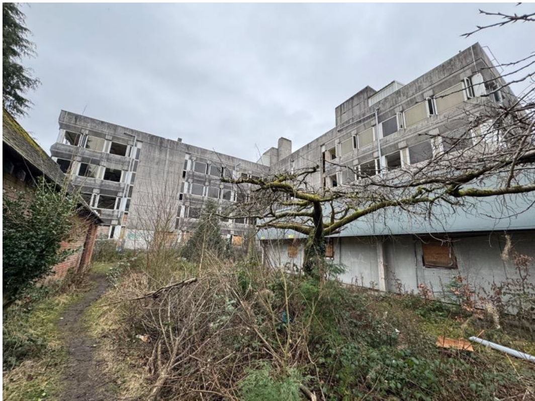
Image 31 – View of inner corner of south and west elevations.
