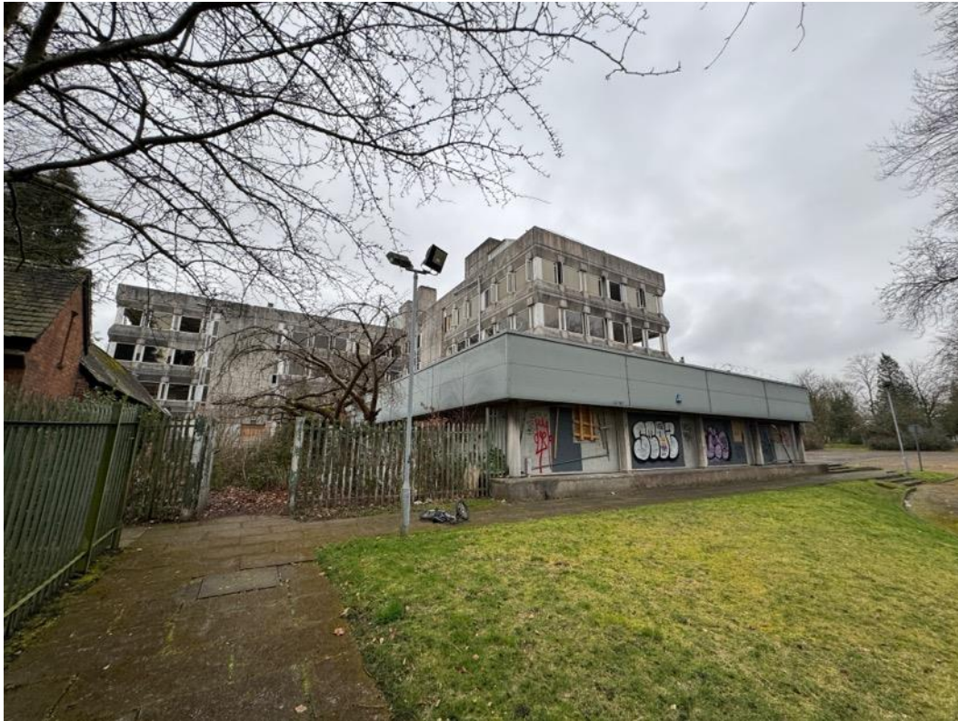
Image 4 – Closer view of southern approach from pedestrian walkway.
