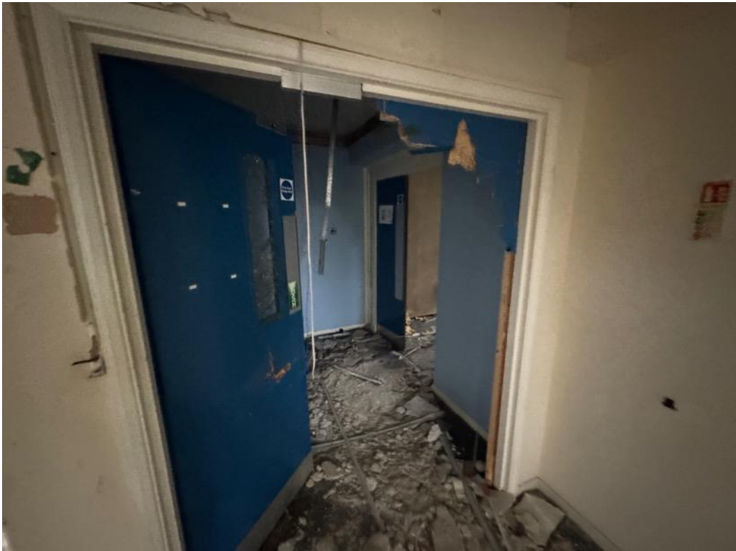
Image 63 – Lobby area to first floor stairwell, northern side.
