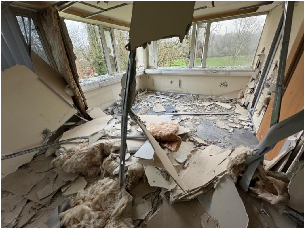
Image 84 – View of second floor office looking at northwest corner.
