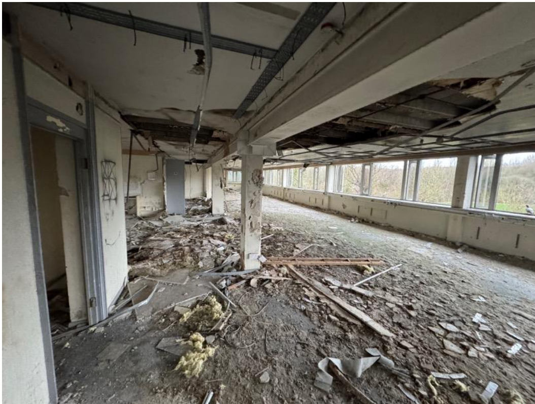
Image 105 – Third floor northeast corner looking west.
