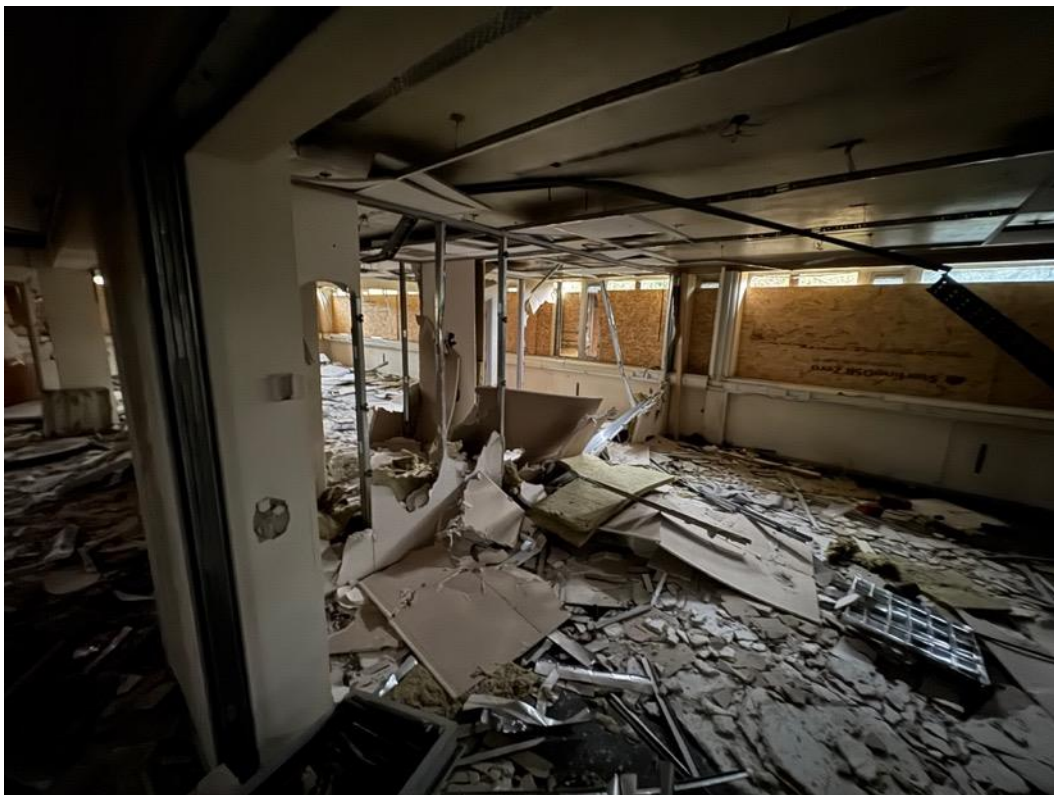
Image 51 – View of internal office spaces to eastern side ground floor.
