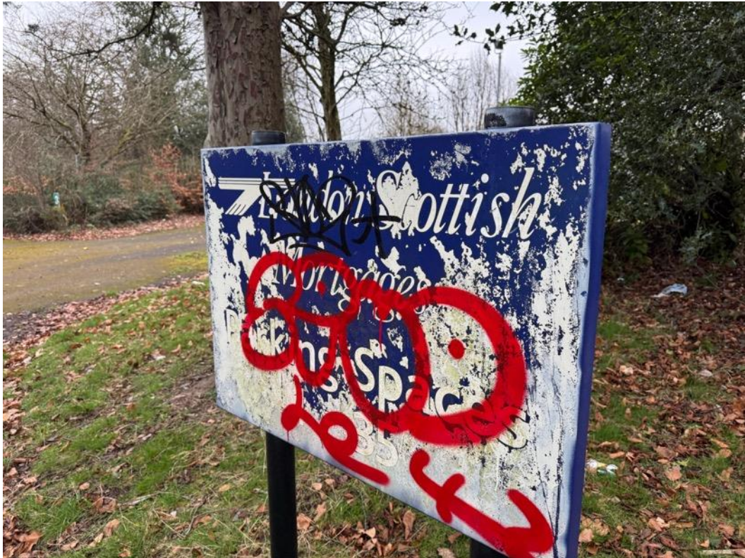
Image 12 – Sign on entrance to east gate, reads “London Scottish Mortgages Parking Spaces – 35” highlighting a former occupier to part of the building.
