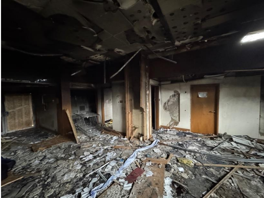
Image 42 – Internal view of entrance hall looking south toward toilet block.
