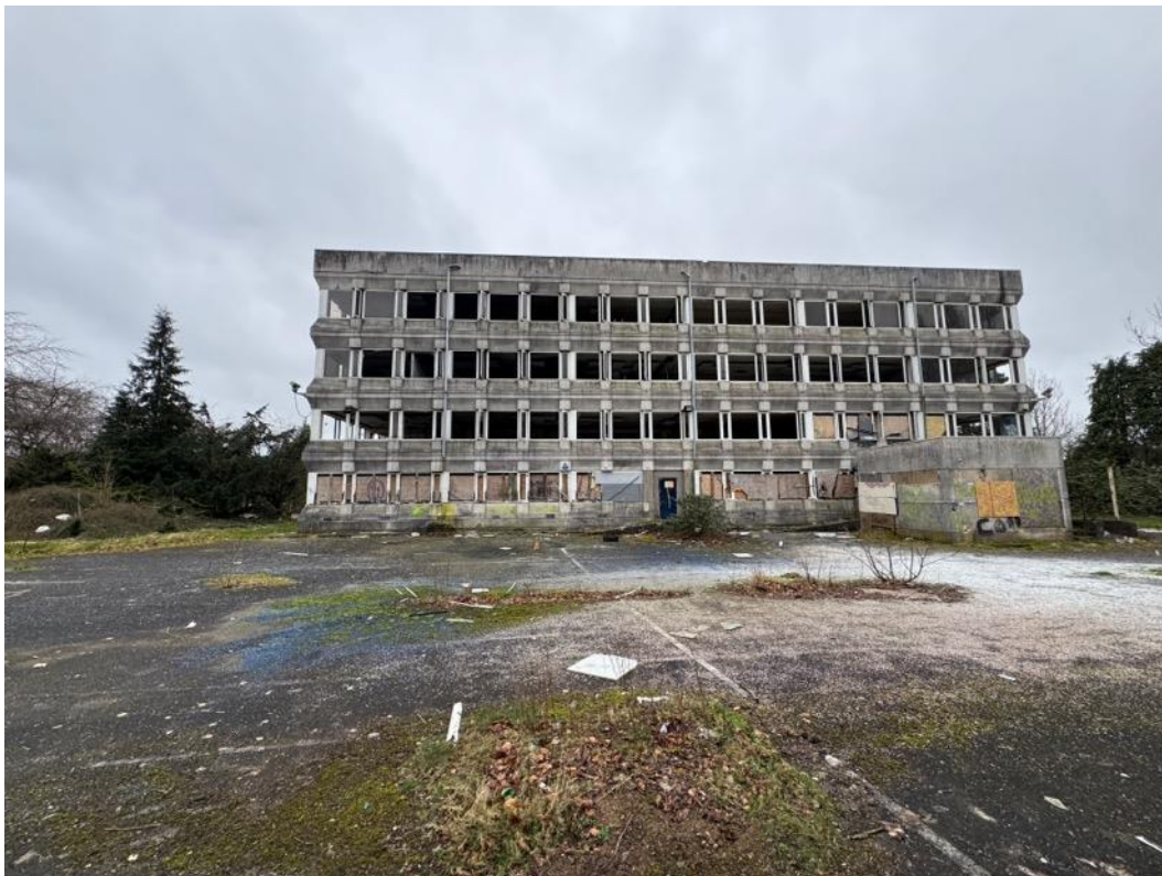
Image 17 – Overall view of north elevation.
