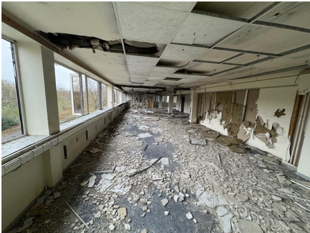
Image 83 – Long view of second floor looking east.
