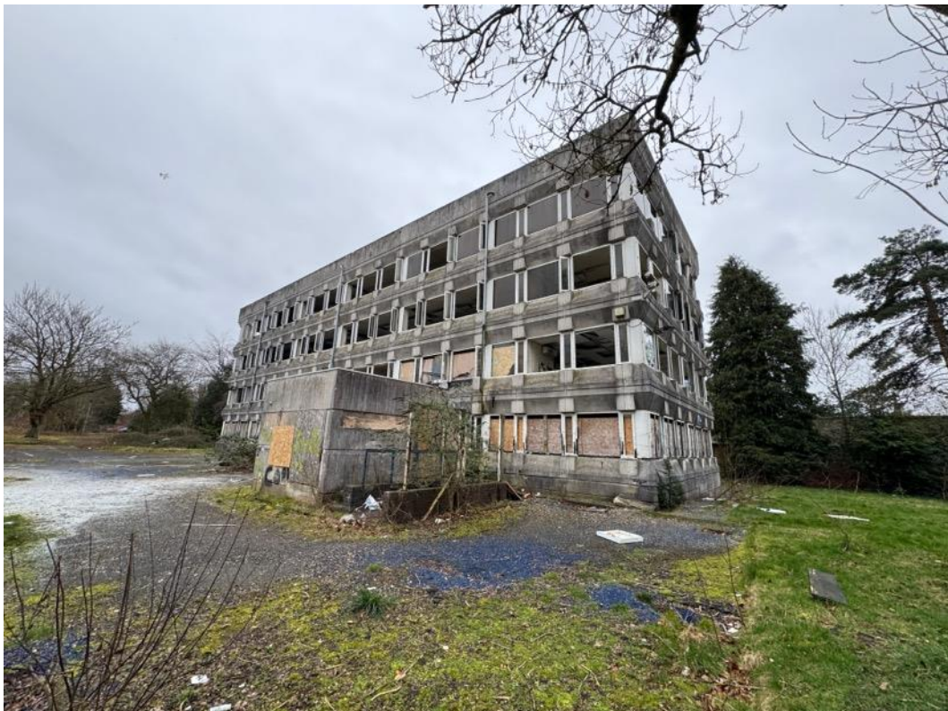
Image 19 – View of northwest corner. Ground floor extension believed to be a plant room or substation.
