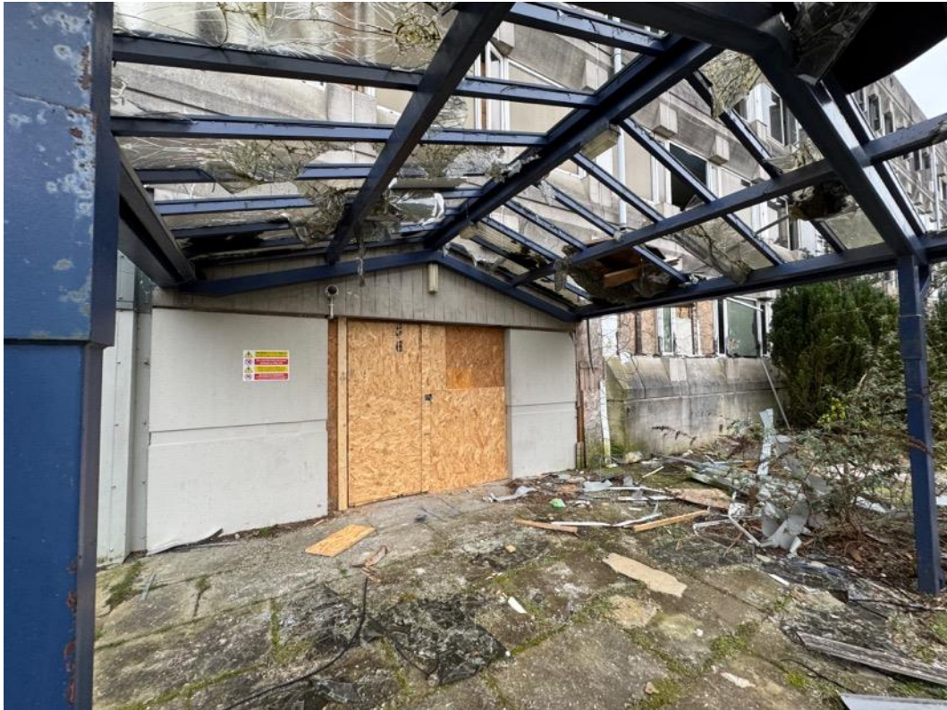
Image 40 – View of main entrance area, with doors boarded to prevent entry.
