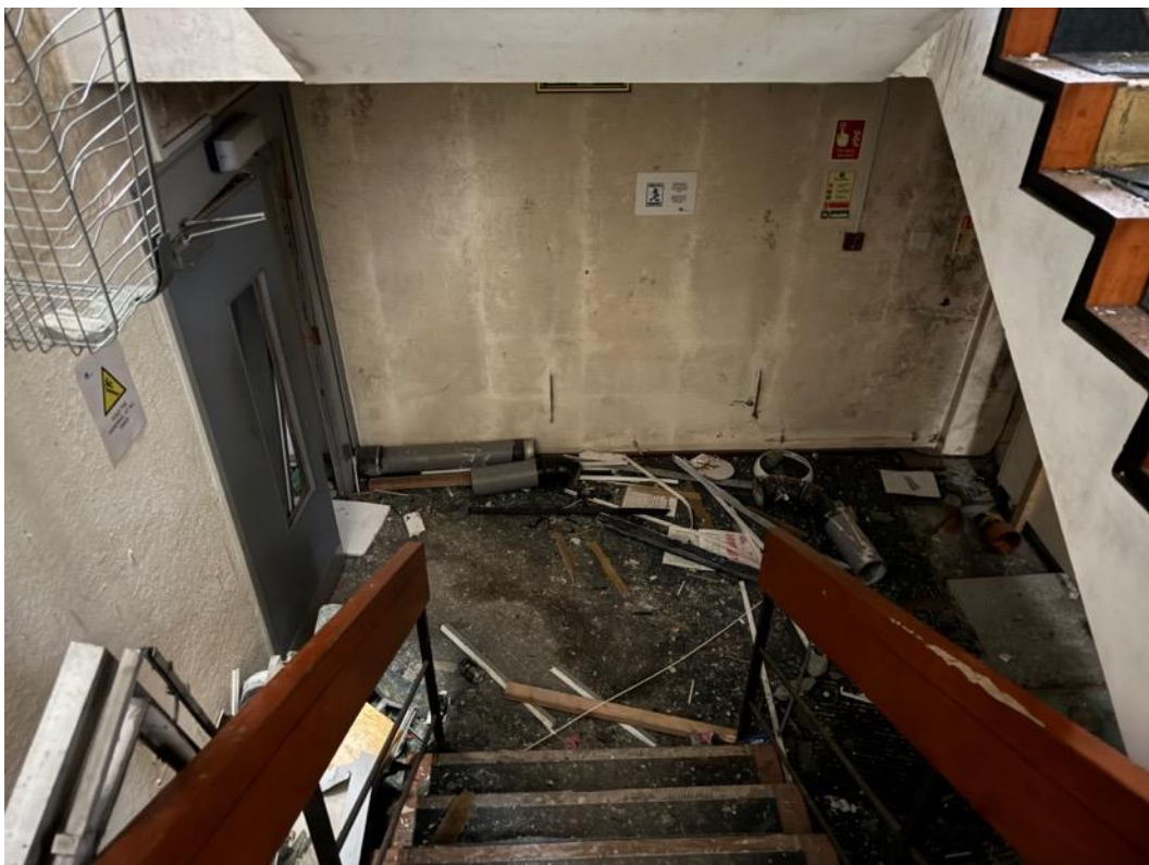
Image 61 – View from half landing down to ground floor from northwest stairwell.
