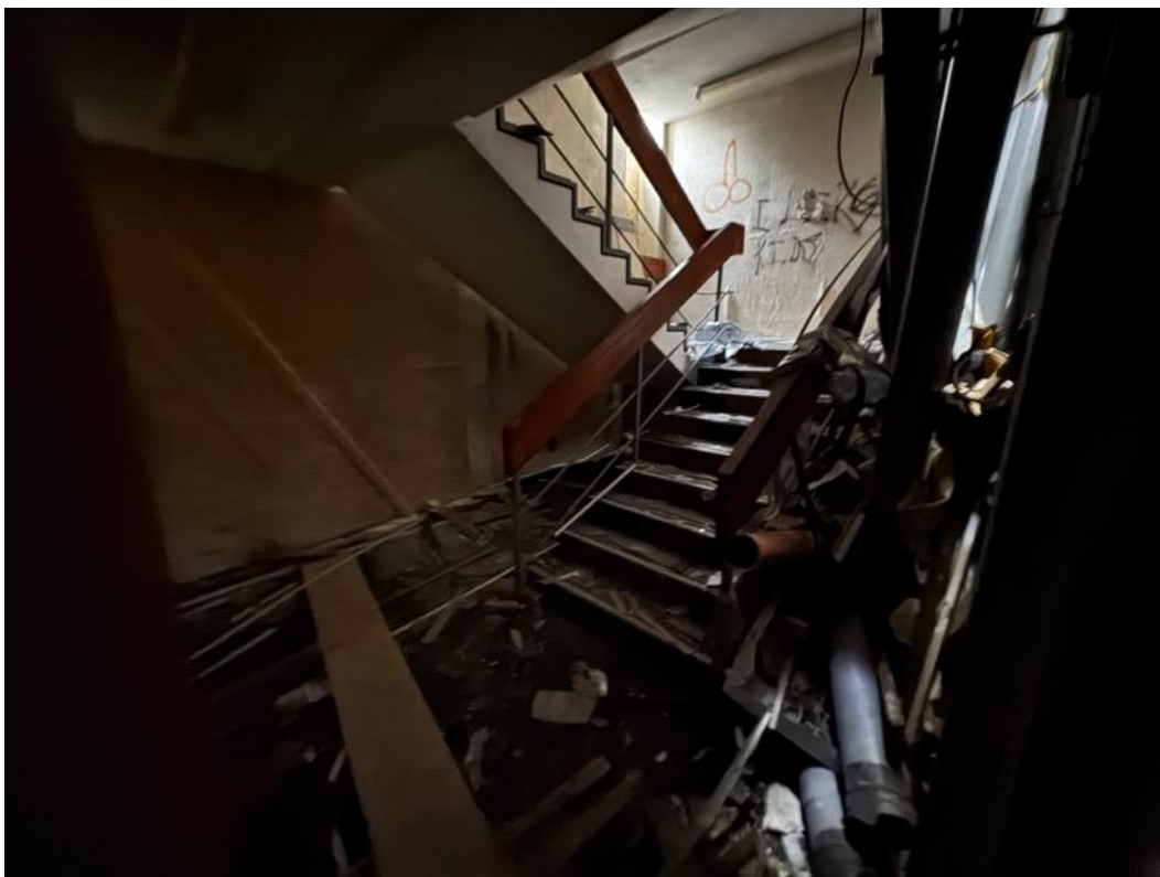
Image 49 – View of stairwell to west elevation. External door boarded to left side.
