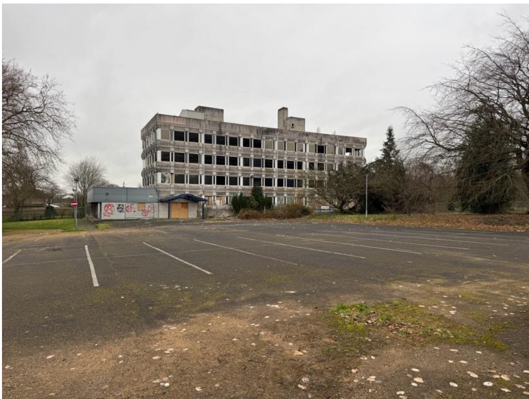
Image 9 – Wider overall view of east elevation from car park.
