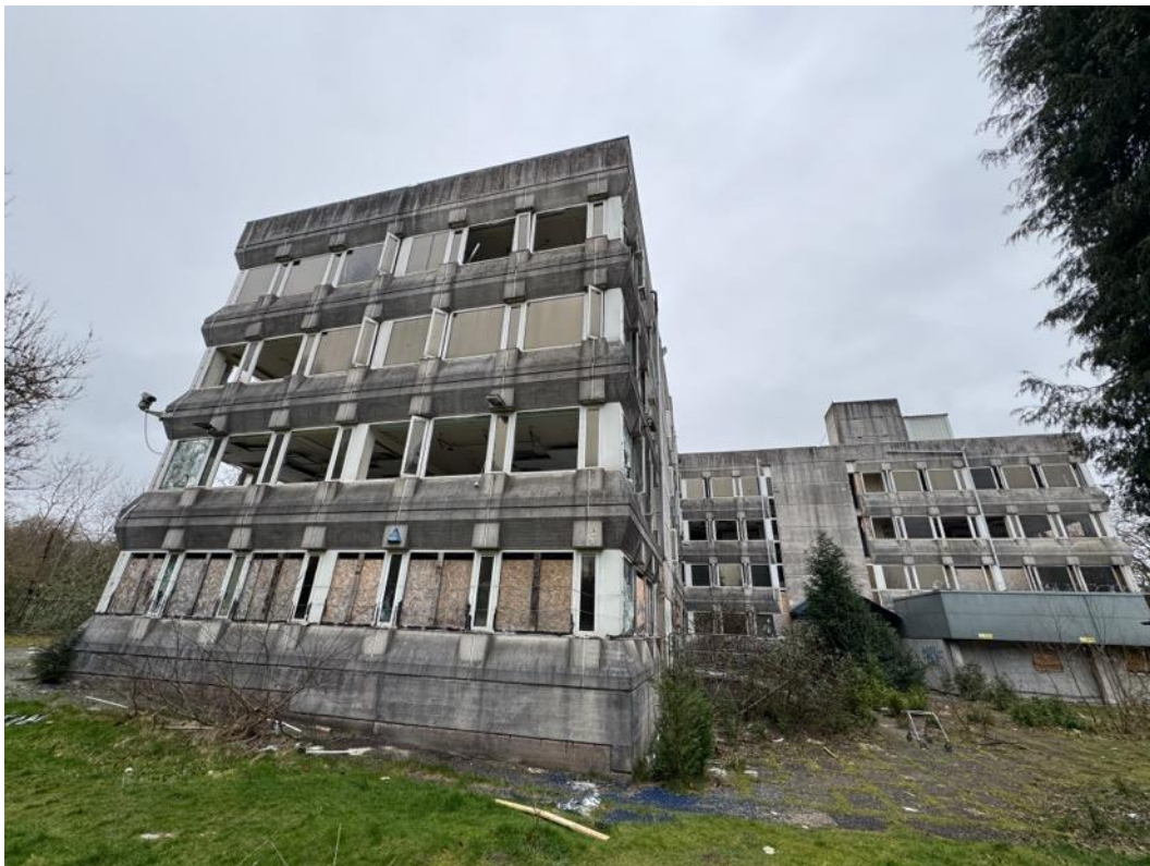
Image 21 – Overall view of west elevation, access restricted by mature trees and site boundary.
