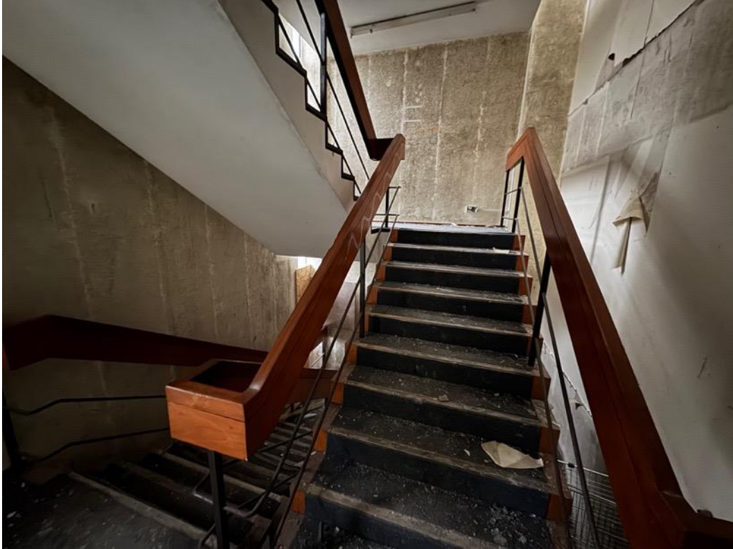
Image 62 – Northwest stairwell, first floor level.
