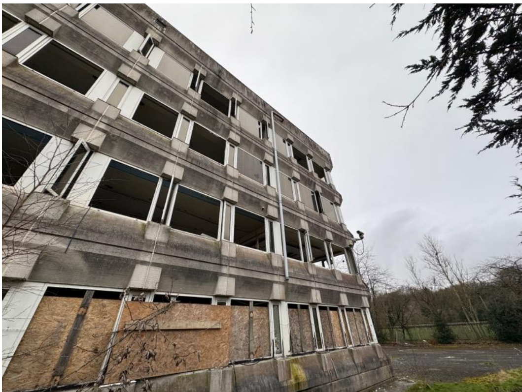
Image 15 – Closer view of northeast corner, access restricted by extensive vegetation.
