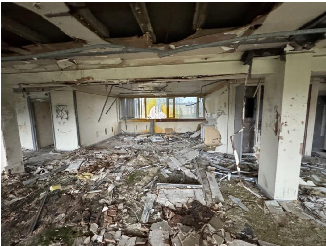
Image 103 – Third floor centre of western end, looking south.
