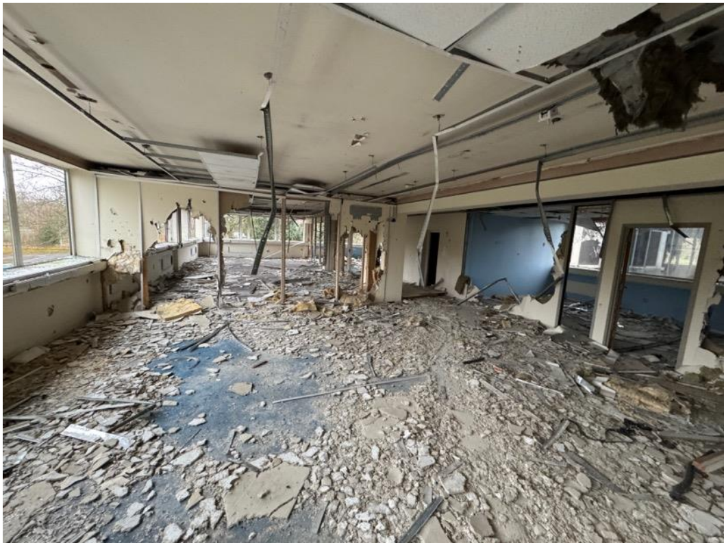
Image 67 – View to centre of north side of first floor.
