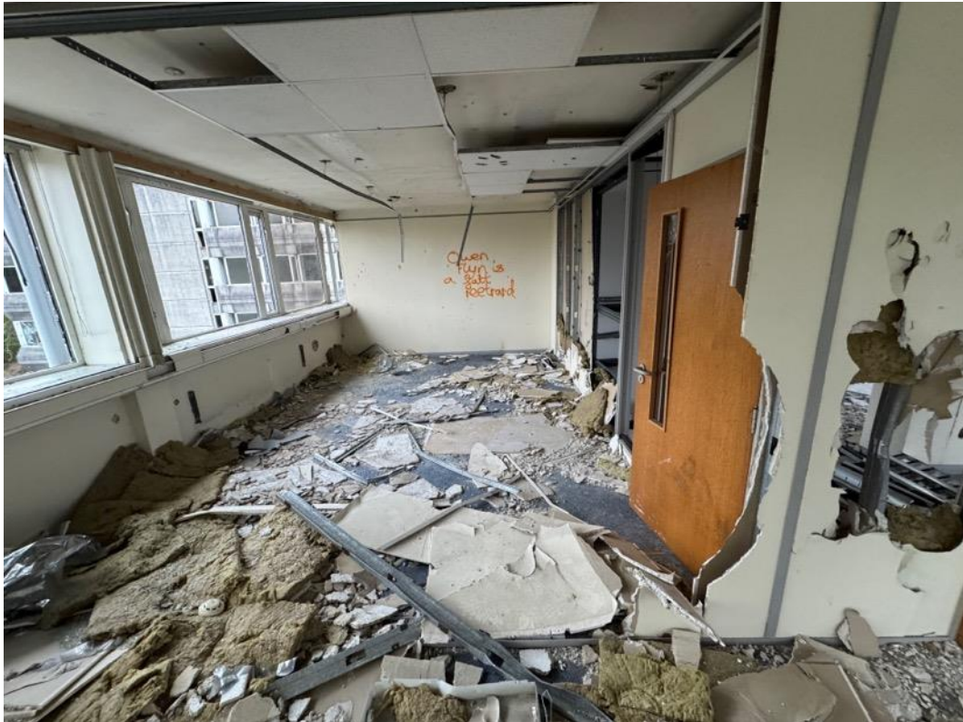
Image 96 – Sub-divided offices, second floor southern end, looking north.
