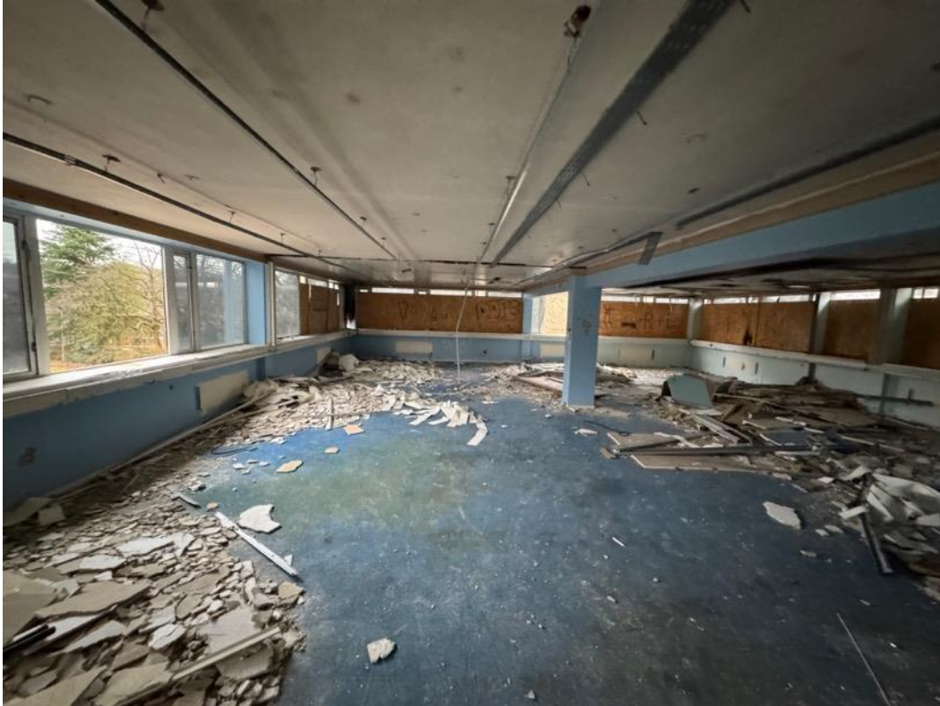
Image 76 - First floor view of southeast corner.
