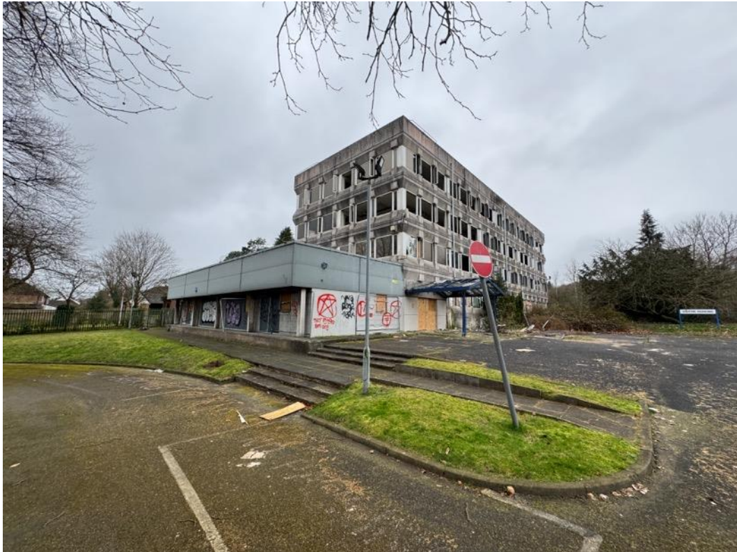
Image 6 – Overall view of southeast corner from driveway approach.
