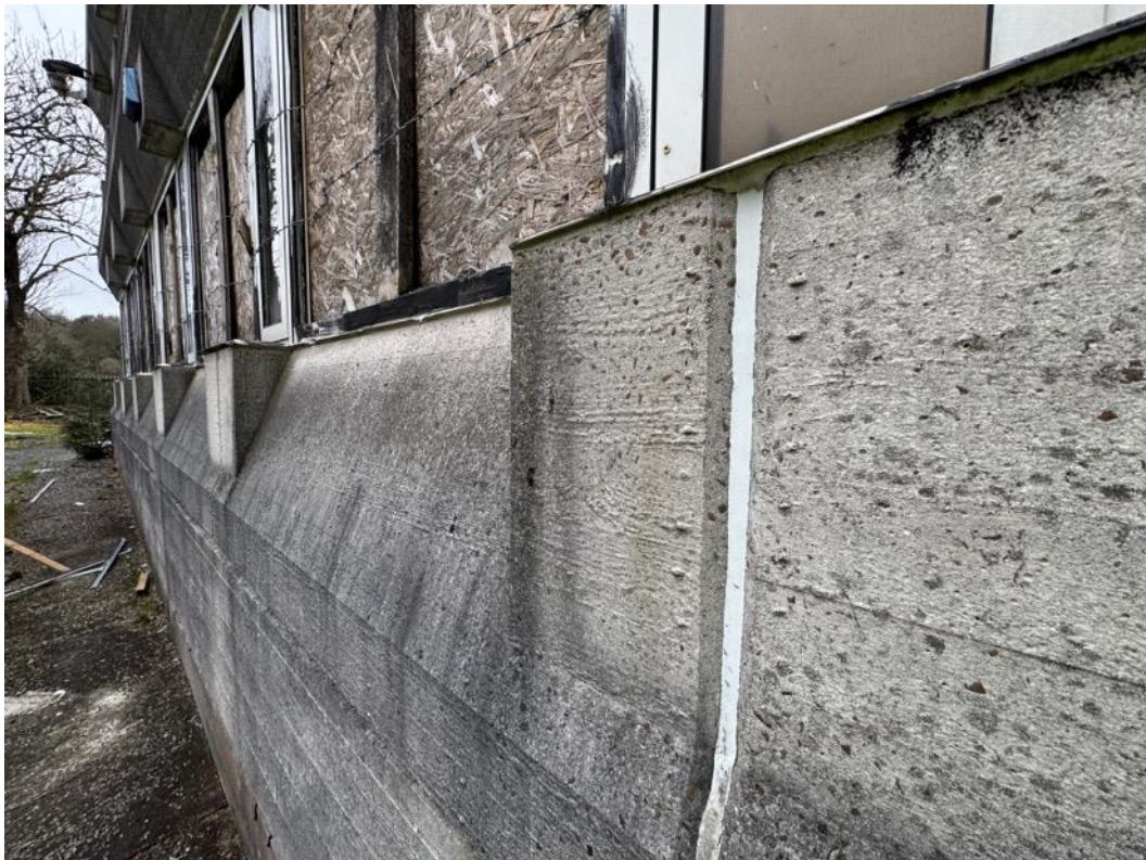
Image 23 – Close-up view of wood grain detail to pre-cast concrete panels, a design feature of the original Brutalist style.
