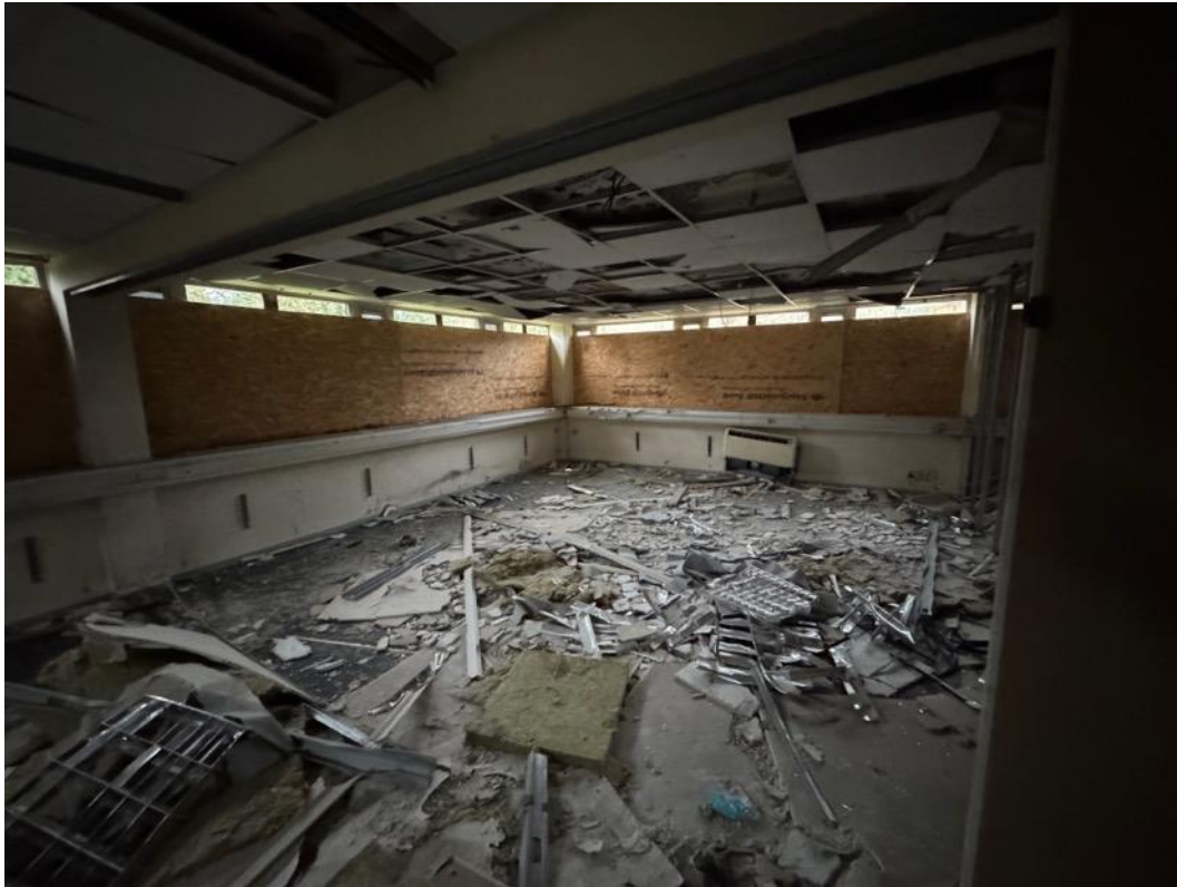
Image 56 – Internal view of northeast corner, ground floor.
