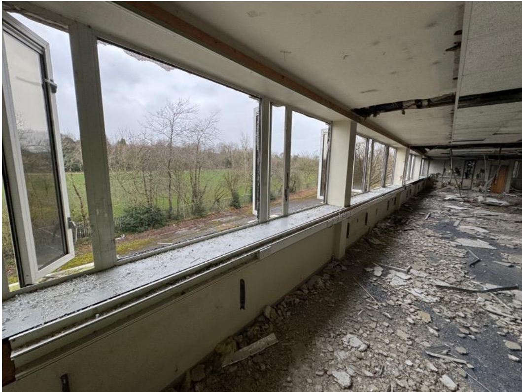
Image 82 – Second floor view of windows to north elevation.
