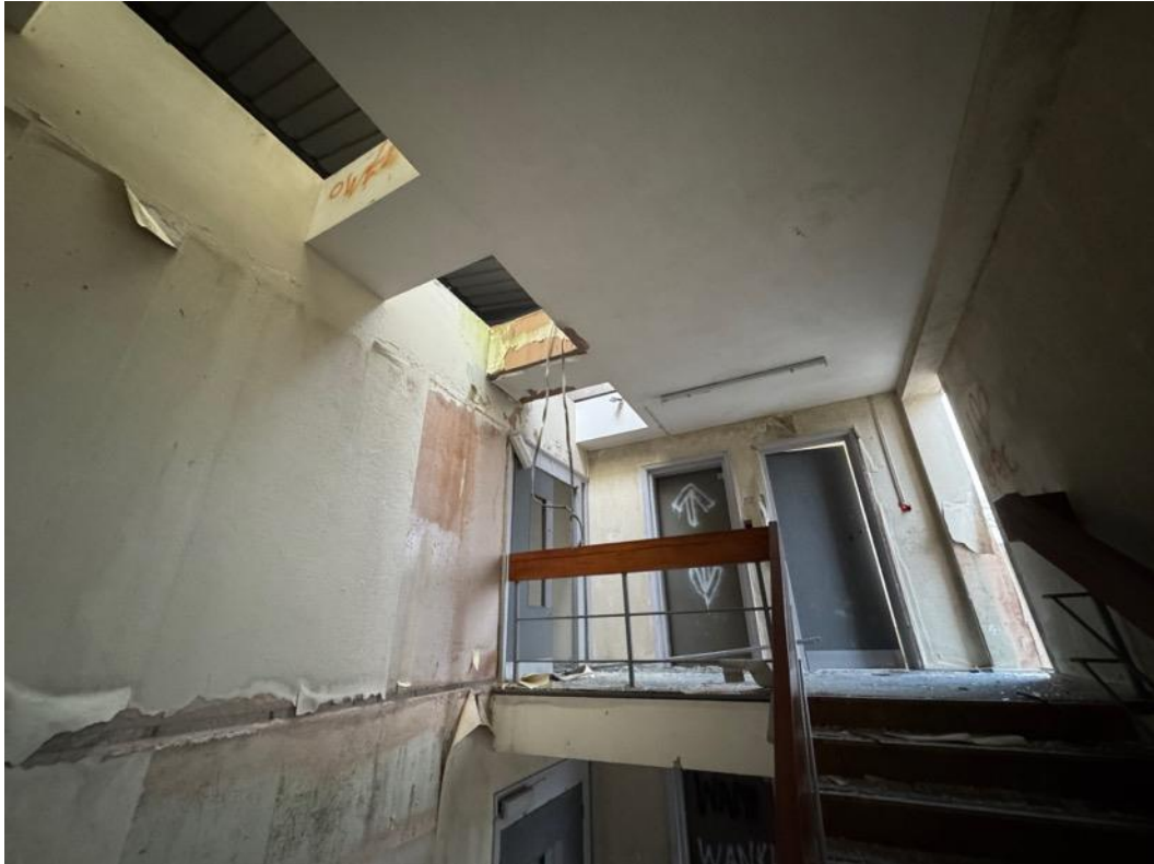
Image 100 – Southern stairwell third floor level, showing skylights and lift doors. Door to right is for a small store cupboard.
