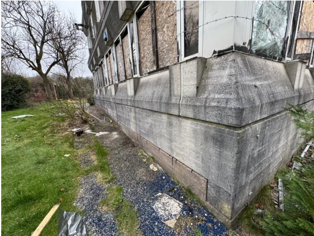
Image 22 – Closer view of west elevation, with some wood grain imprints to pre-cast concrete panels.
