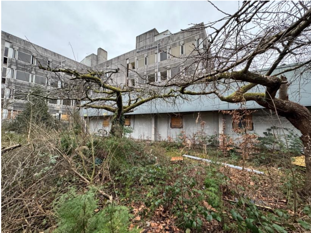
Image 30 – View of west elevation of ground floor extension. Courtyard garden area now heavily overgrown. Original glazing to length of extension has been removed and overclad.
