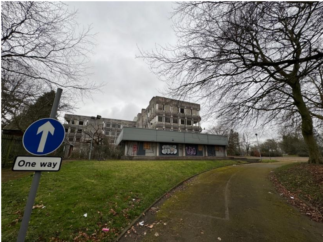
Image 5 – Overall view of southern side, from driveway approach.
