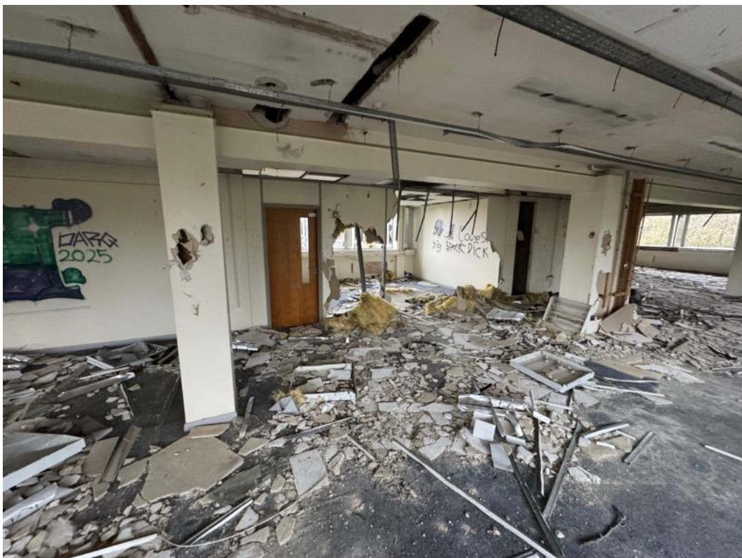
Image 91 – View of office to west side of southern section.
