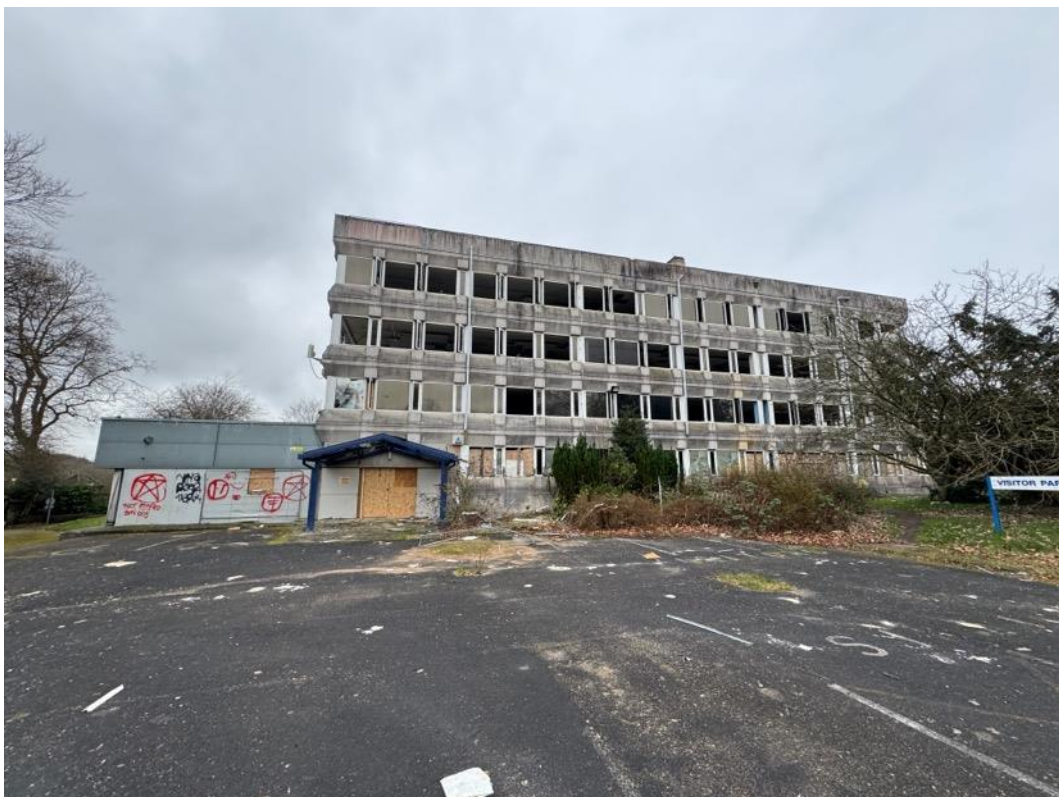
Image 7 – Overall view of east elevation from car park.
