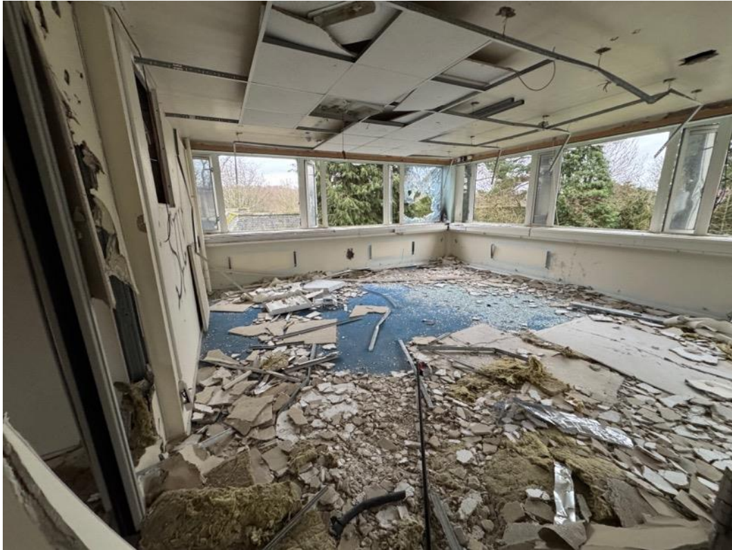
Image 64 – View of west end of first floor. Suspended tile ceiling remains in part.
