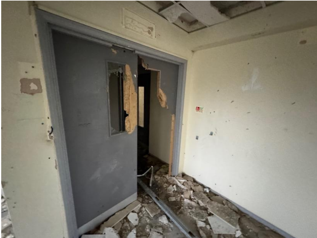
Image 60 – View of doors to stairwell to northwest.
