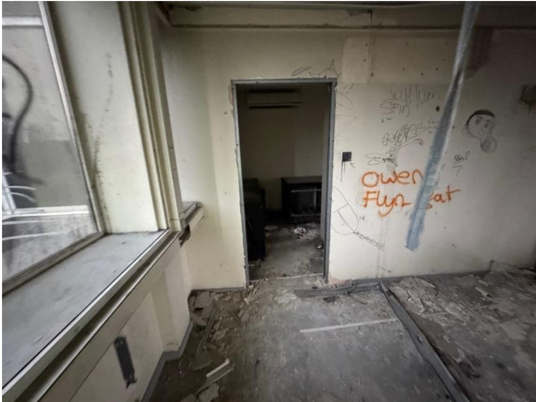
Image 106 – Former server room to centre of third floor looking north.
