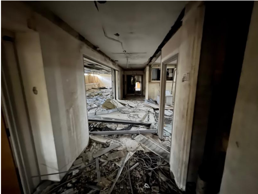
Image 50 – View down length of ground floor corridor.
