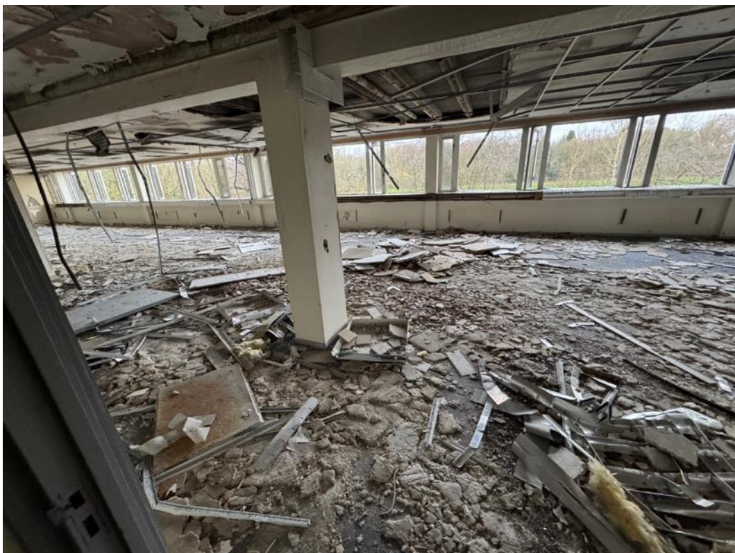
Image 89 – Second floor view looking north.
