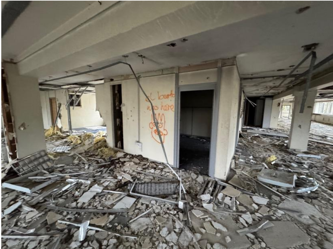
Image 98 – Rooms to centre of second floor, presumably storerooms due to lack of windows.
