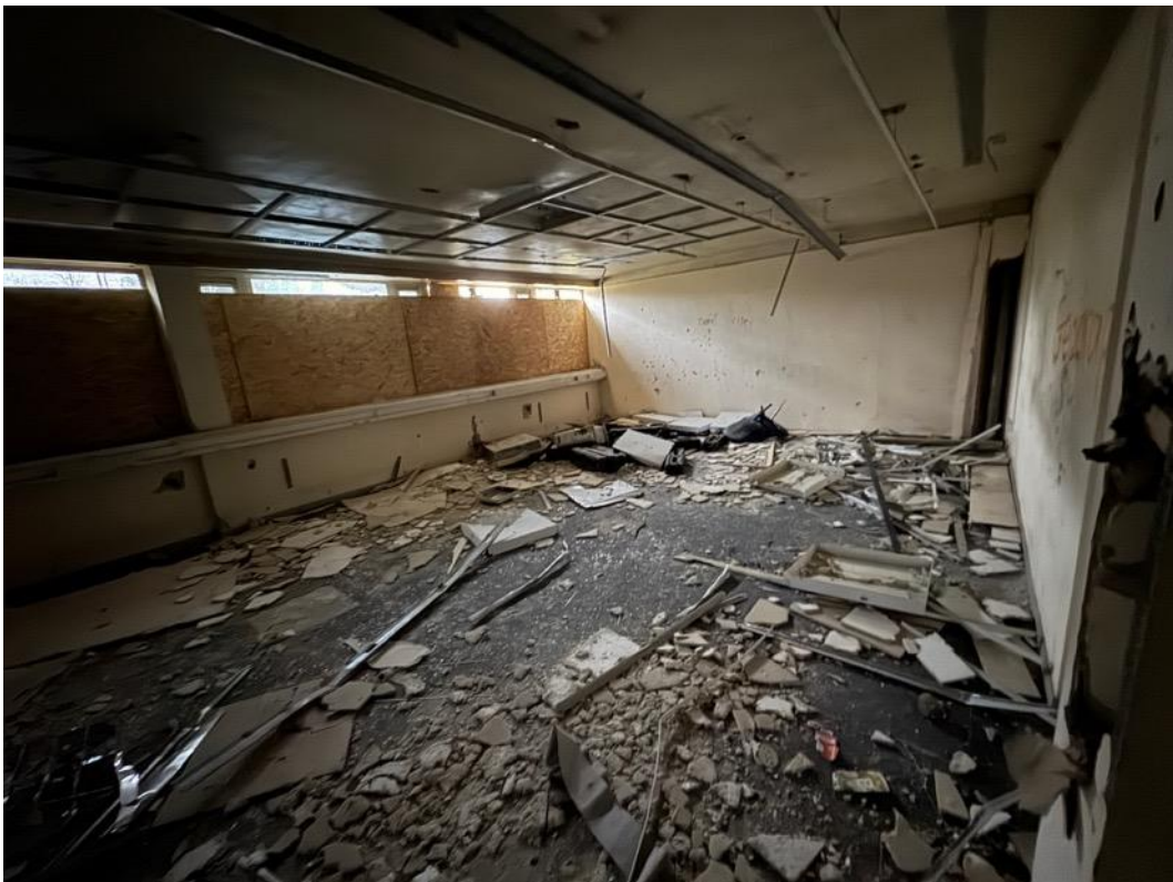
Image 53 – Office space to ground floor from central corridor.
