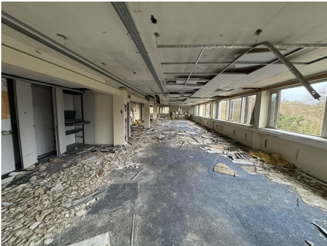
Image 97 – Overall internal view looking toward the north, second floor.
