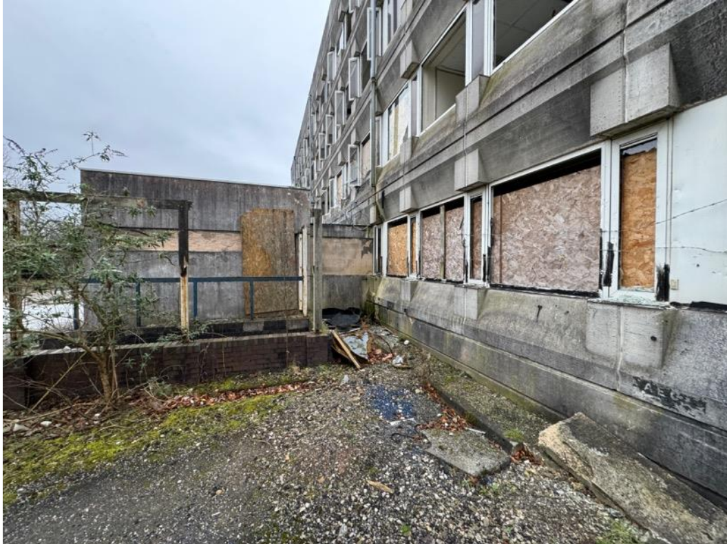
Image 20 – Closer view of northwest corner, showing connection of extension to main building.
