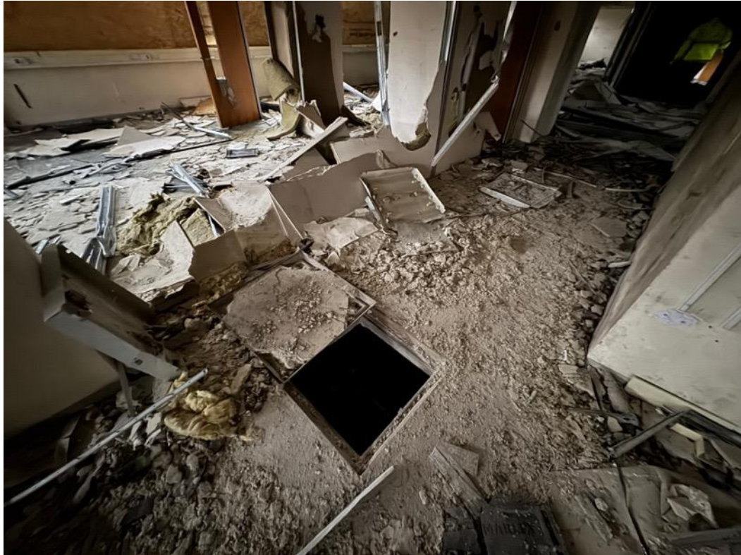
Image 59 – Access point to service duct in floor.
