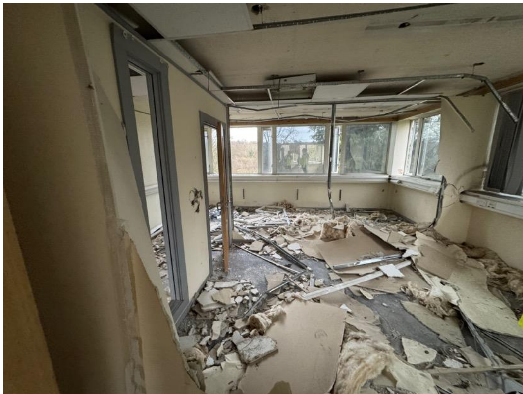
Image 85 – View of second floor offices at western end, looking south.
