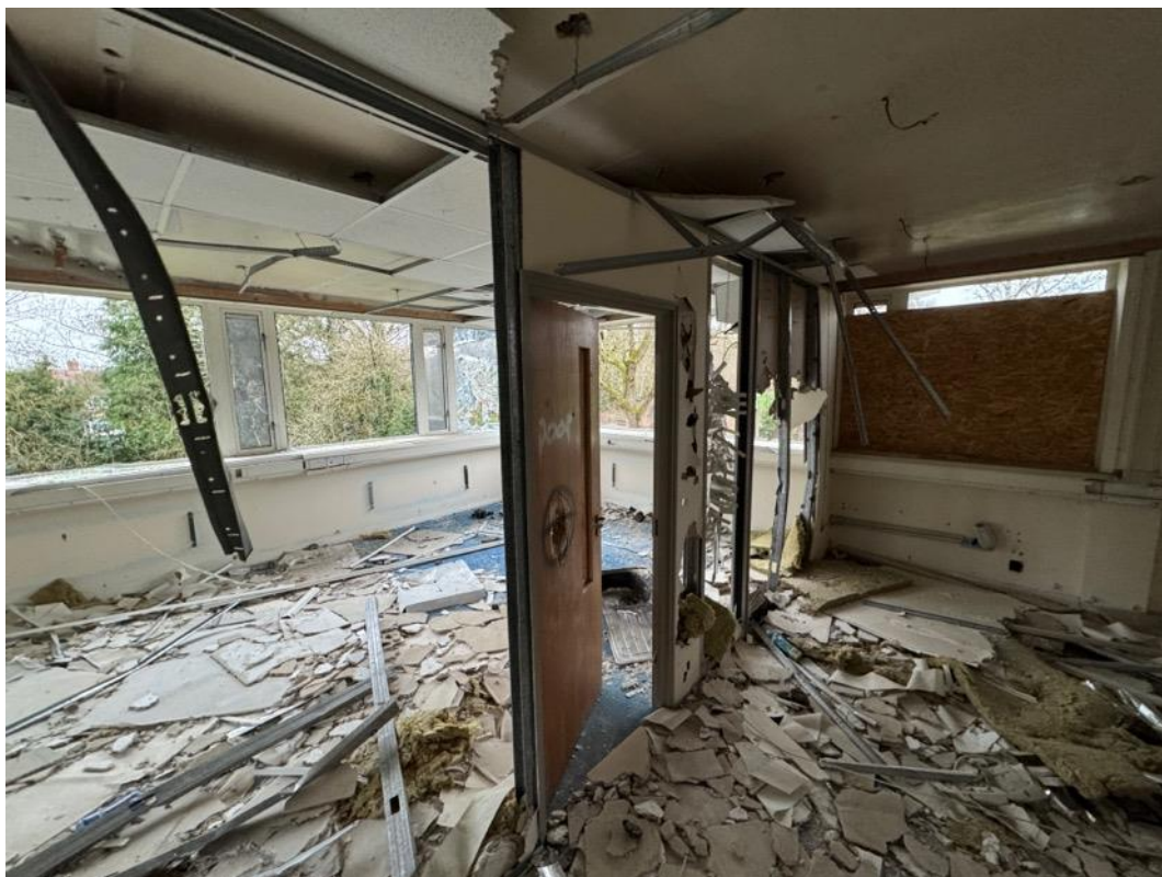
Image 65 – Internal view, first floor looking to northwest.
