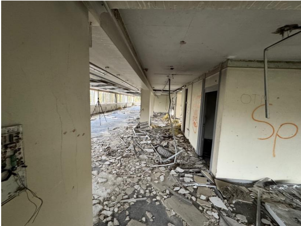
Image 90 – View looking south from the central inner corner.
