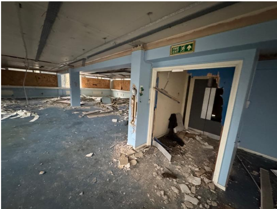
Image 77 – View into southern stairwell doors, sealed shut at time of survey.
