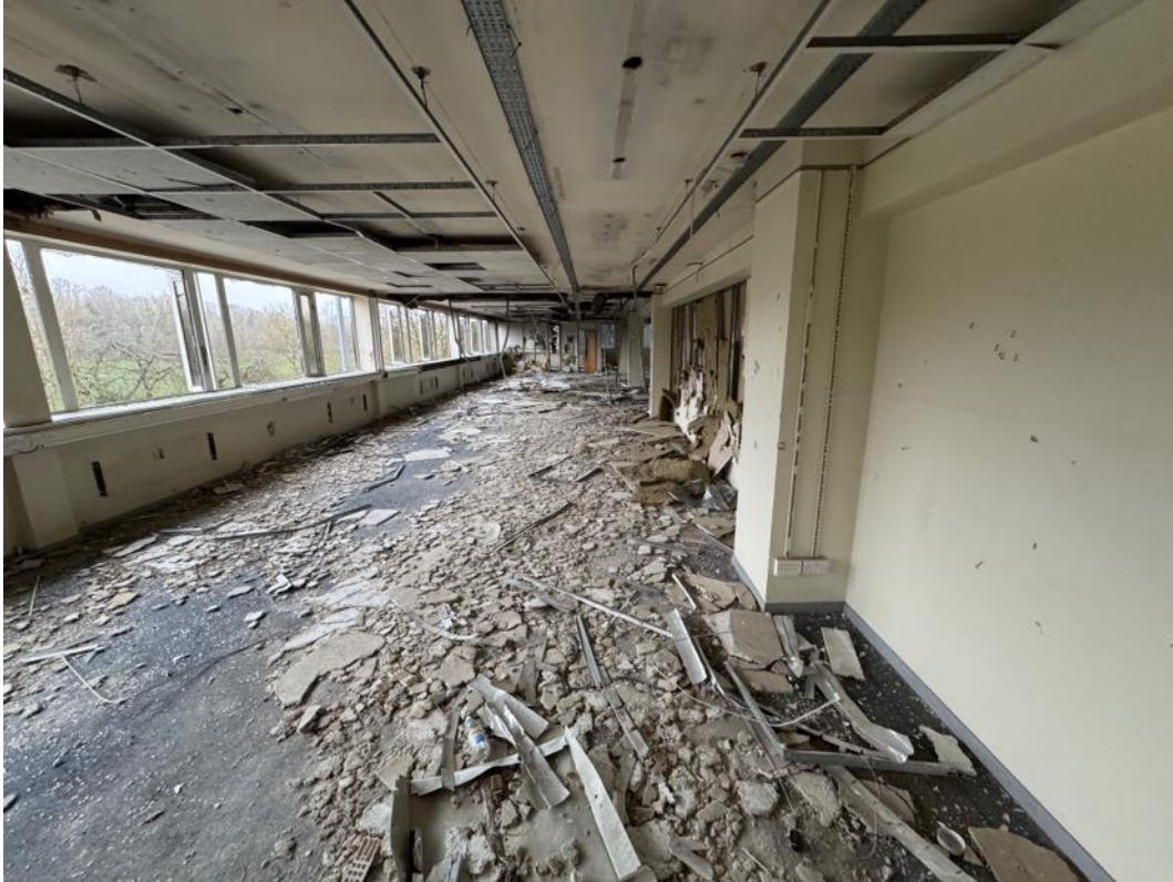
Image 86 – Second floor view looking east.
