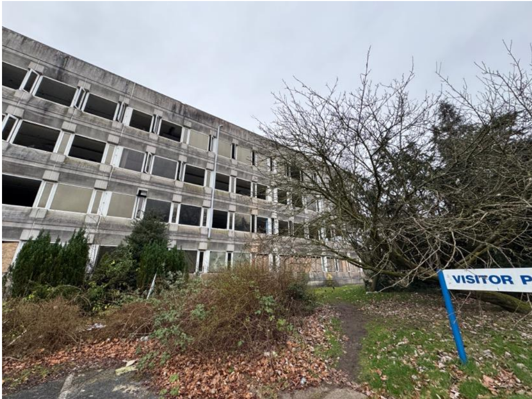
Image 14 – Closer view of east elevation, some vegetation obscures a full view.
