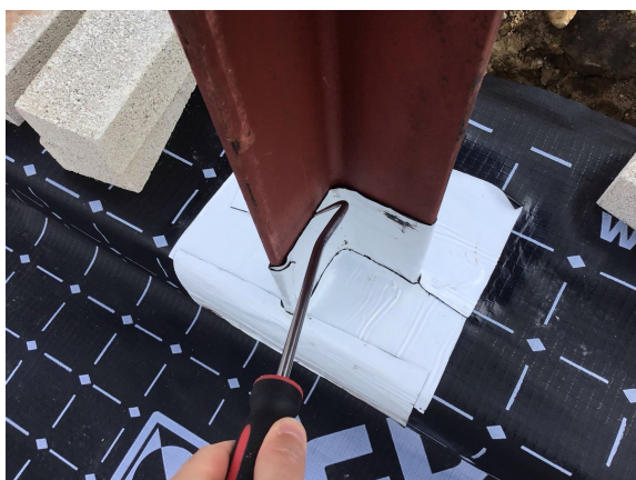
Testing the windpost detailing
