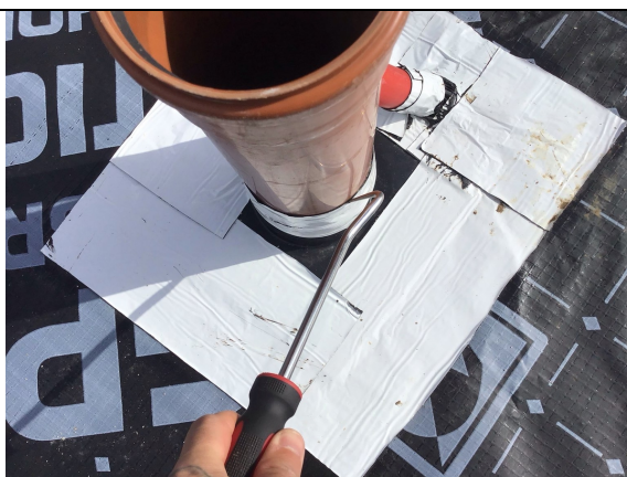
Testing the pipe detailing
