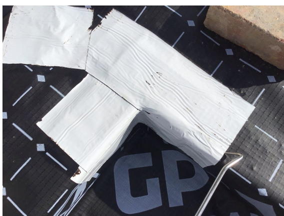
Testing the corner detailing
