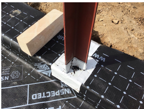
Windpost detailing
