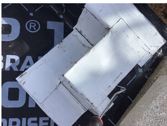
Testing the threshold detailing
