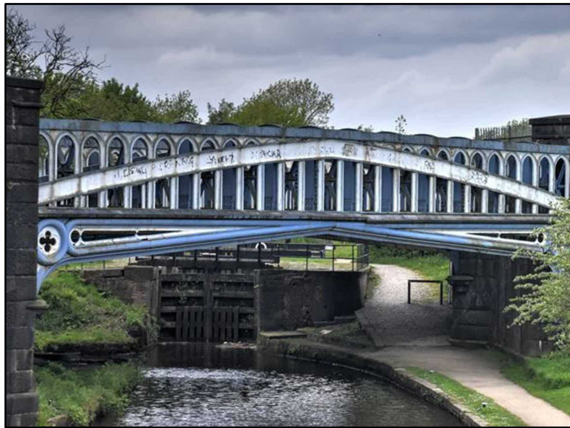
IMAGE SHOWING EAST ELEVATION OF BRIDGE PRIOR REMOVAL OF DECORATIVE SPANDRELS
