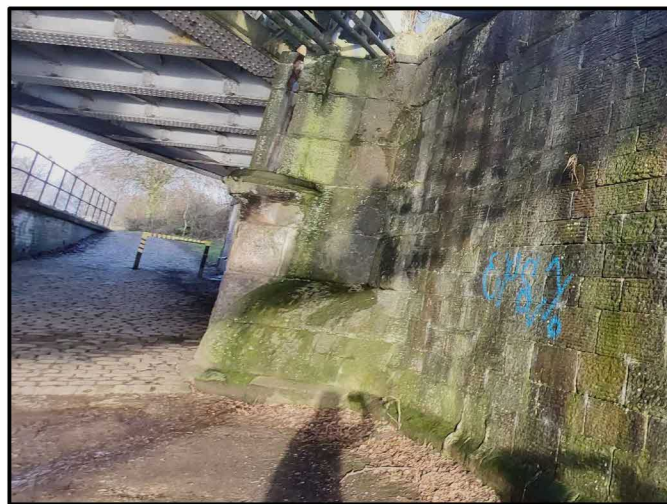
PHOTO 3 - STONE CORBEL AT WEST END OF NORTH ABUTMENT
