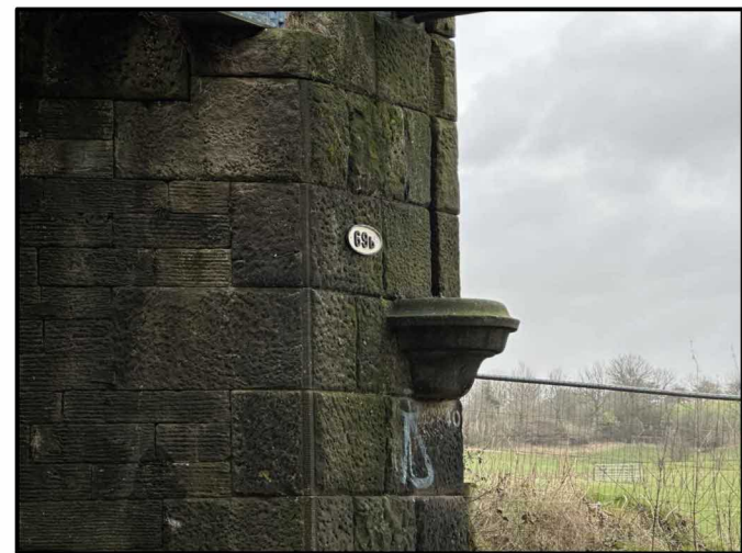
PHOTO 1 - STONE CORBEL AT EAST END OF NORTH ABUTMENT
