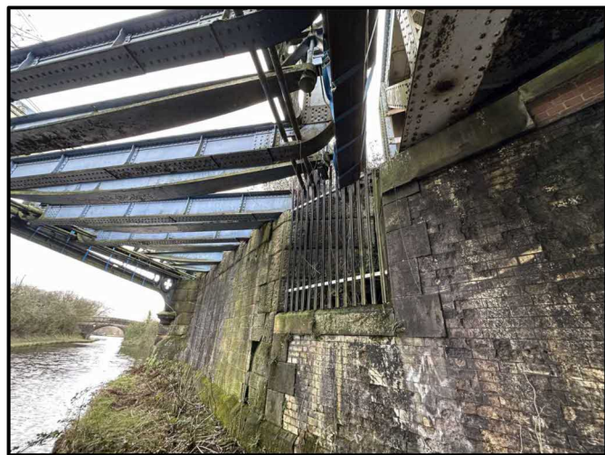
PHOTO 4 - PALISADE FENCING OBSCURING CORBEL AT WEST END OF SOUTH ABUTMENT
