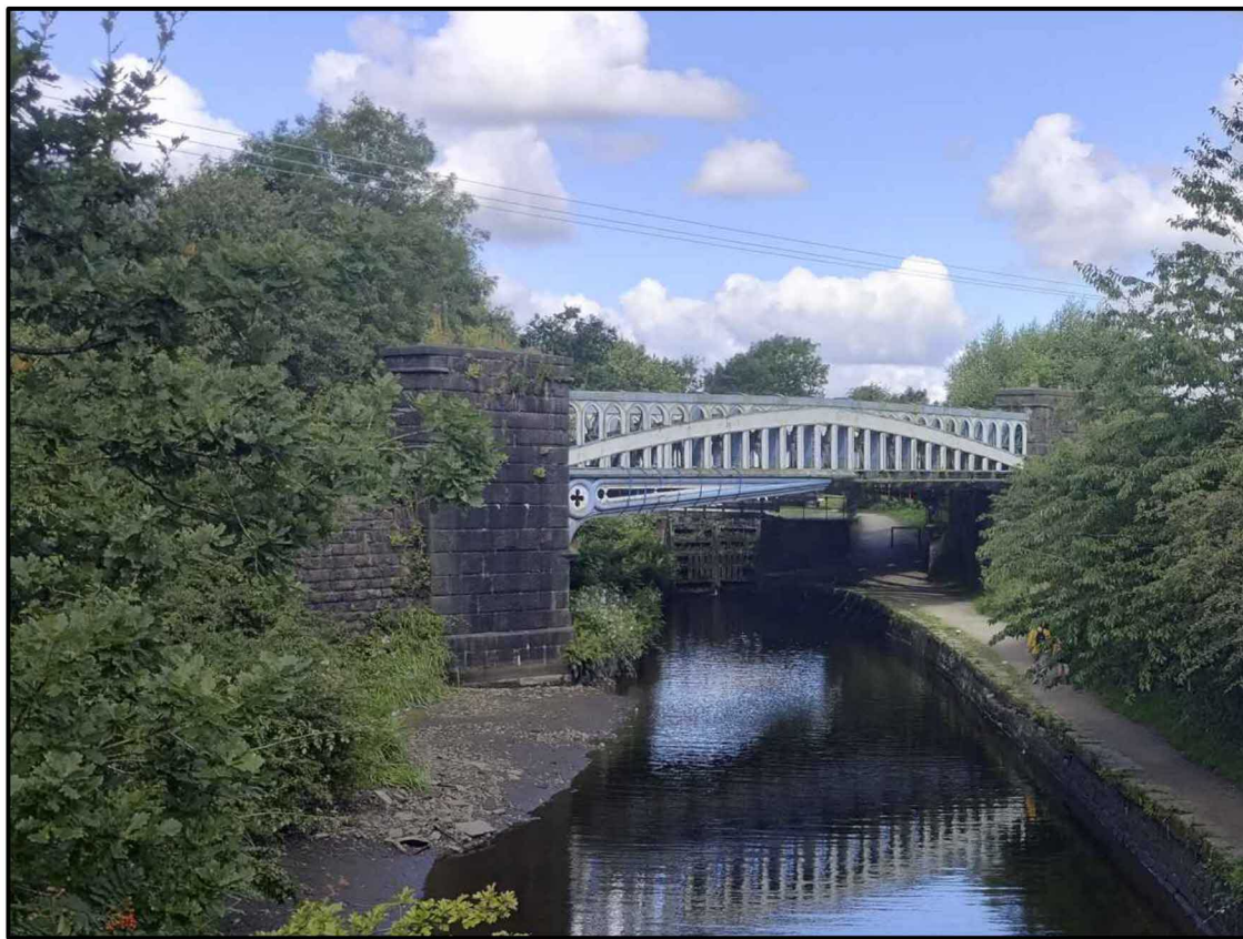
IMAGE SHOWING EAST ELEVATION OF BRIDGE FOLLOWING THE REMOVAL OF 1No. DECORATIVE SPANDREL (23/07/2024)
