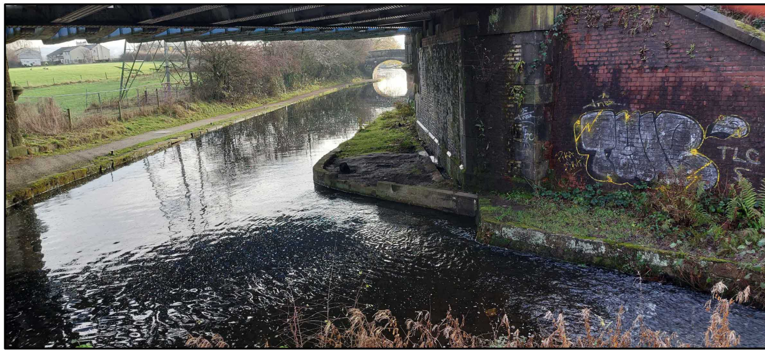
PHOTO 4 - LOW MILEAGE ABUTMENT & WING WALL (12/03/2025)
