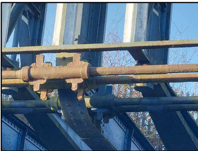
PHOTO 6 - WROUGHT IRON TENSION RODS
