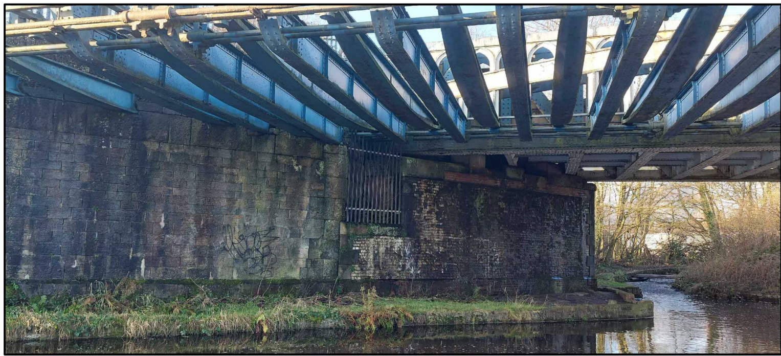
PHOTO 3 - DISUED DECK AND LOW MILEAGE (SOUTH) ABUTMENT (12/03/2025)
