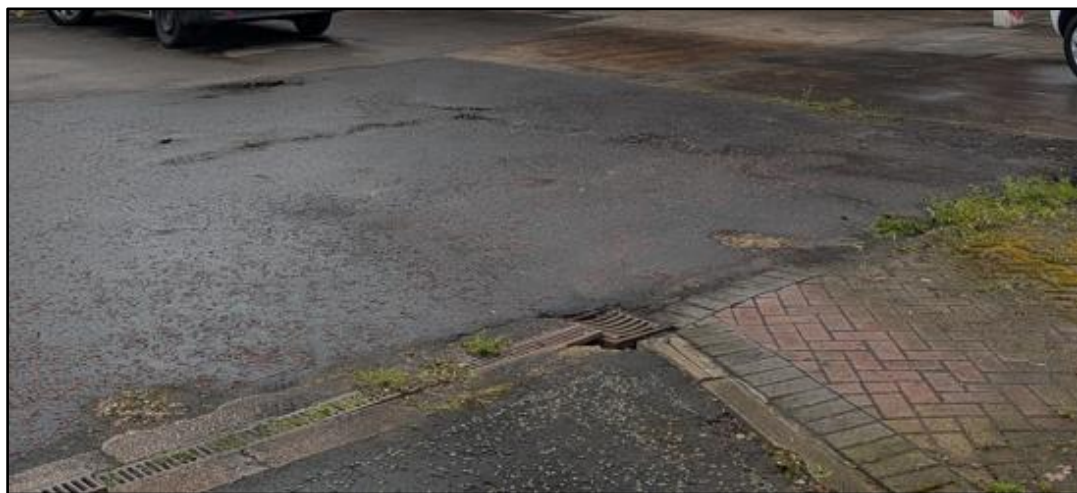
Photograph 6 – Hardstanding entrance to the site (P4)
