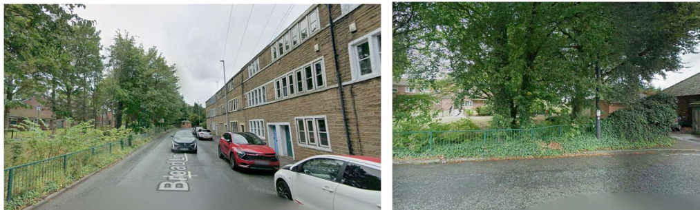
Above left – view along Broad Lane with listed buildings to right and planting screen to left
