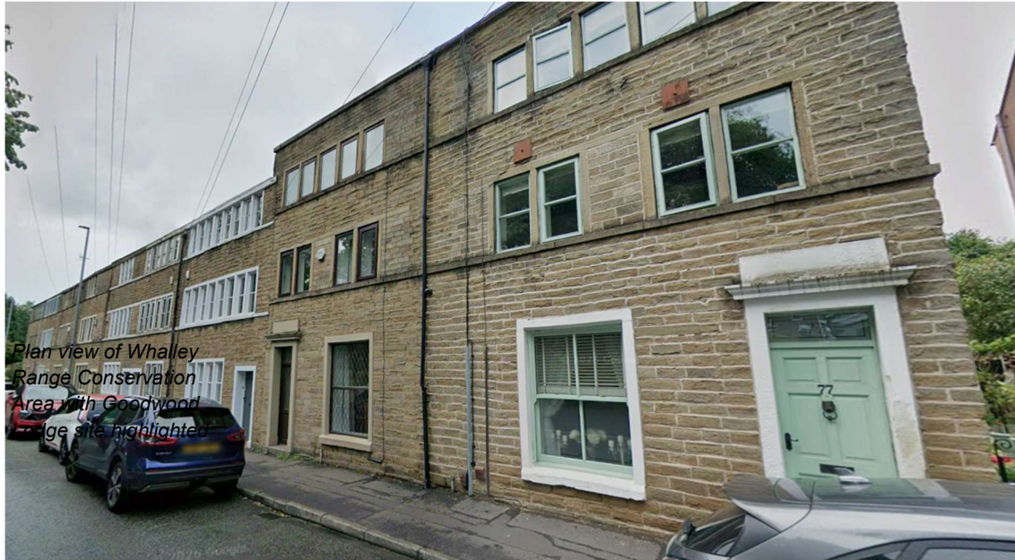
Above – view of listed properties located on Broad Lane (image Google Maps)
