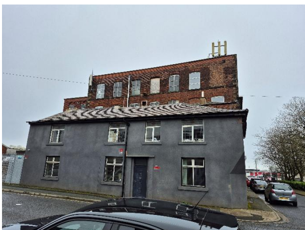
Photo 5: West face of B2.
