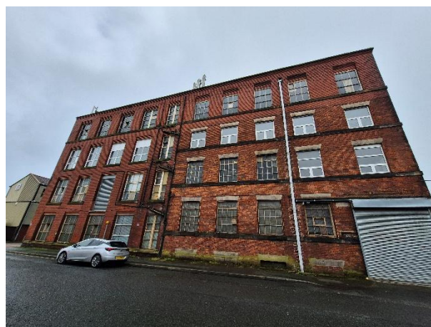
Photo 6: North face of B1.
