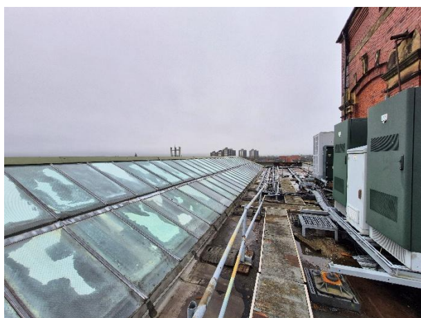
Photo 9: Hipped glass area on roof of B1.
