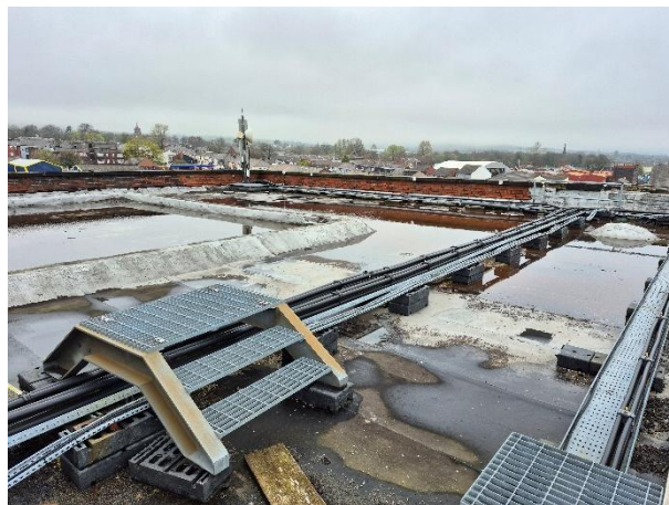
Photo 8: Roof of B1.
