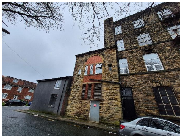
Photo 4: Southwest corner of B1 and south face of B2.
