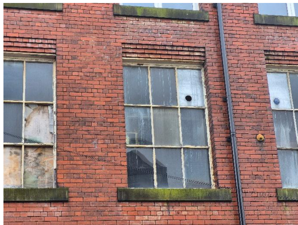
Photo 14: Vent hole on B1 second storey.
