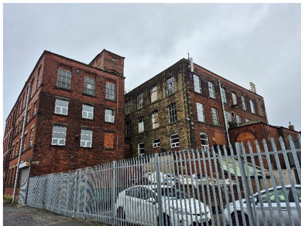
Photo 7: Northwest area of B1.
