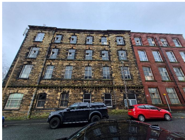
Photo 2: East face of B1.
