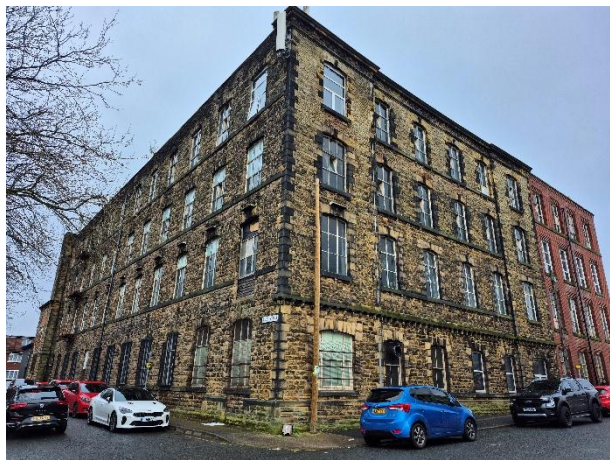
Photo 1: Southeast corner of B1.
