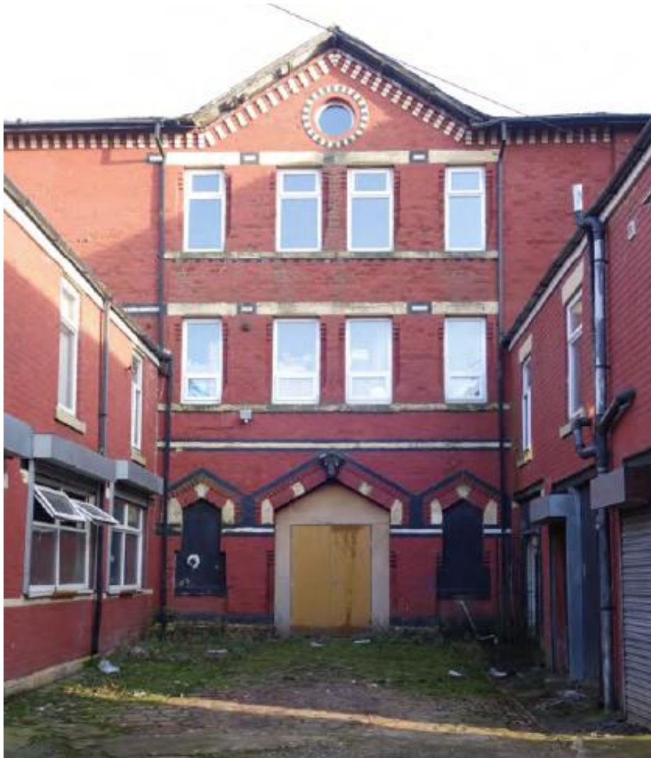
3.7 Above: Courtyard area looking towards front portion of building, new windows and doors to be installed to ground floor
