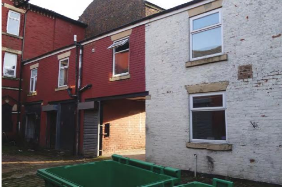
3.9 Above: South eastern elevation from courtyard area showing undercroft access.
