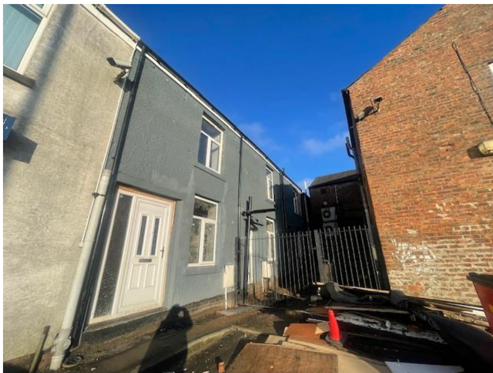
Photo 1: Photo of southern/front elevation of application site at 2, 4 and 6 Sutcliffe Place. Source: Case Officer Site Visit Photos.
