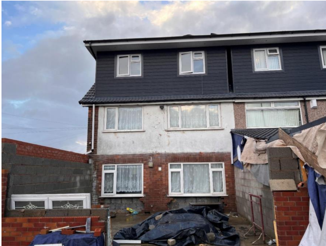
Figure 1 - Site Photo of Application Property on 24.11.25 (Source: Author)
