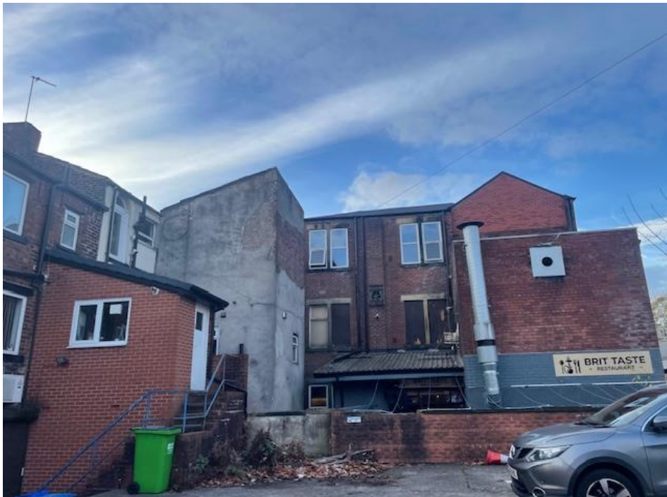
Photograph 1: Site visit photo from western elevation of the building, showing the existing flue and extractor fan on the rear of the property. Source: Case Officer
