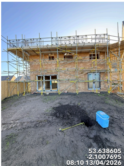
Plot 47 520mm imported topsoil over an orange marker layer - Vistry agreed to top up this plot and send confirmatory photographs
