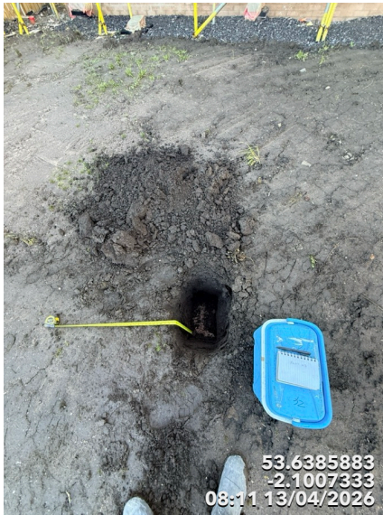
Plot 47 520mm imported topsoil over an orange marker layer
