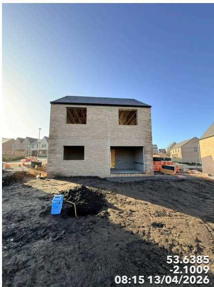
Plot 49 660mm imported topsoil over an orange marker layer
