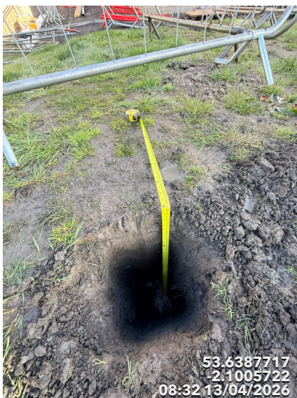
Plot 43 760mm imported topsoil over an orange marker layer
