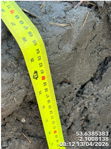
Plot 48 650mm imported topsoil over an orange marker layer
