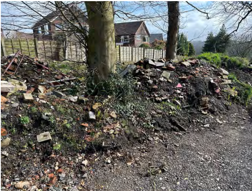
Photographic plate showing the build-up of construction waste and suspected change in ground levels surrounding trees T1 and T5 (ROAVR, 2026).
