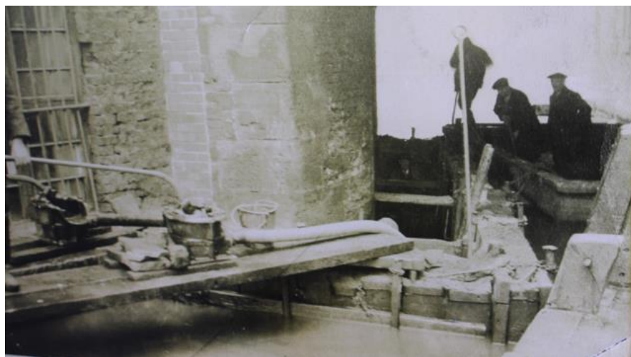
Plate 20 - Men working on pontoon on Rochdale Canal (date and author unknown) The Canal and River Trust Archives.
