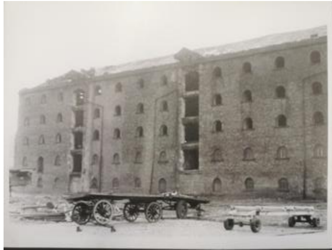
Plate 16 - Eastern elevation of central warehouse- Rochdale Local Studies
