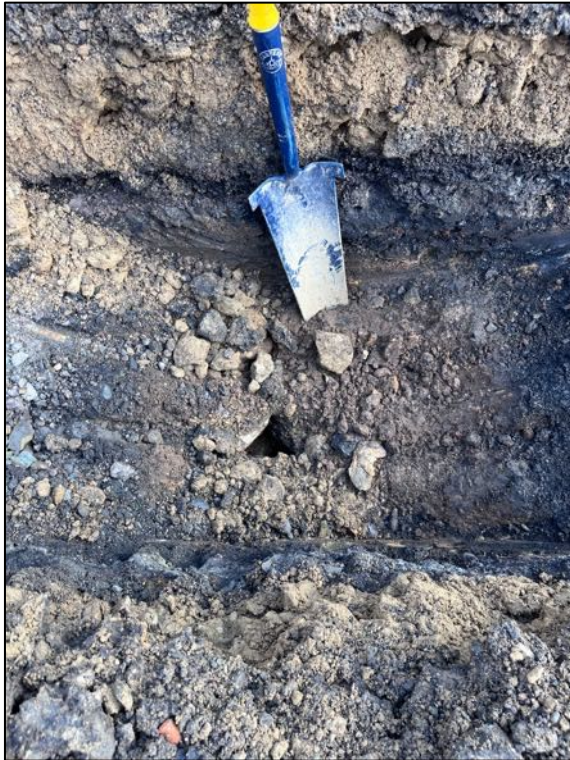
TP4 old land drain exposed
