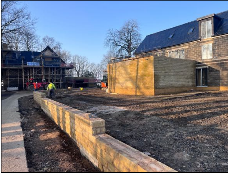
General view looking south west from site entrance at Crimble Lane
