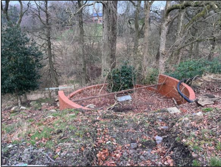
View to the west of a disused drainage structure land immediately west of the site – attempting to highlight ground level falling steeply on adjacent land
