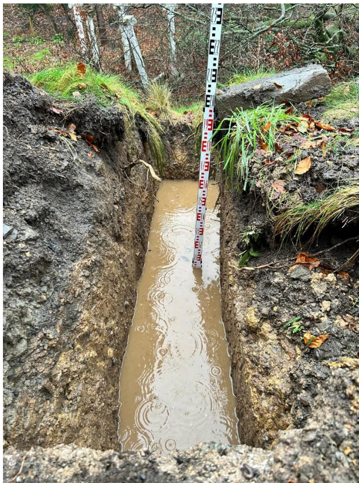
Figure 4: Failed Infiltration Testing 18/11/25
