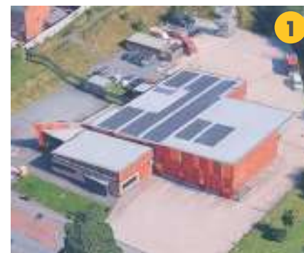
Rochdale Community Fire Station
