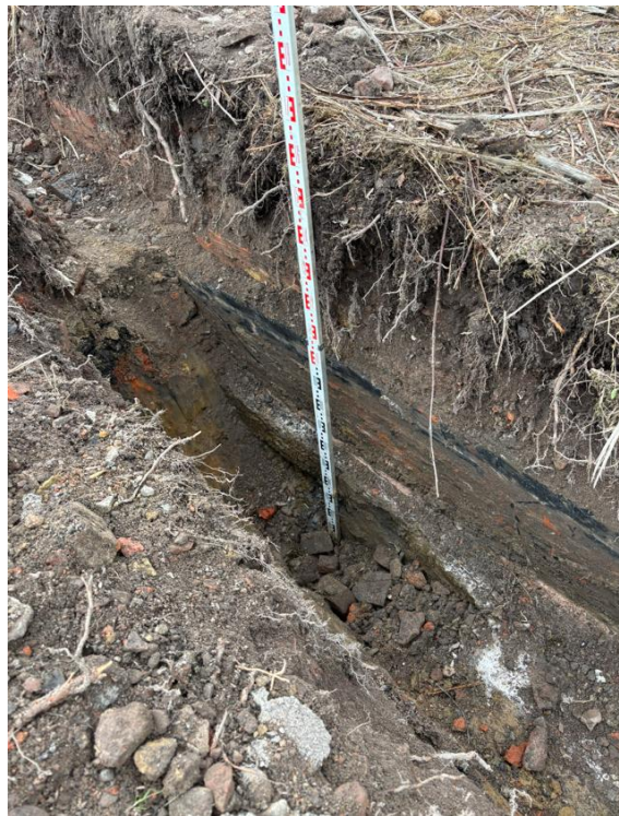
TT01 East - Brick wall and footings
