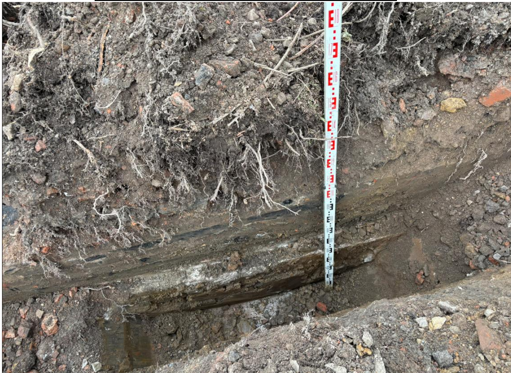
TT01 East - Brick wall and footings
