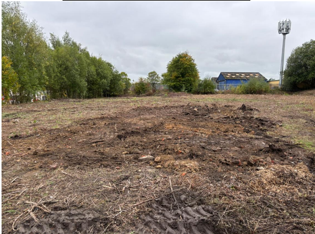
Trial trench area reinstated
