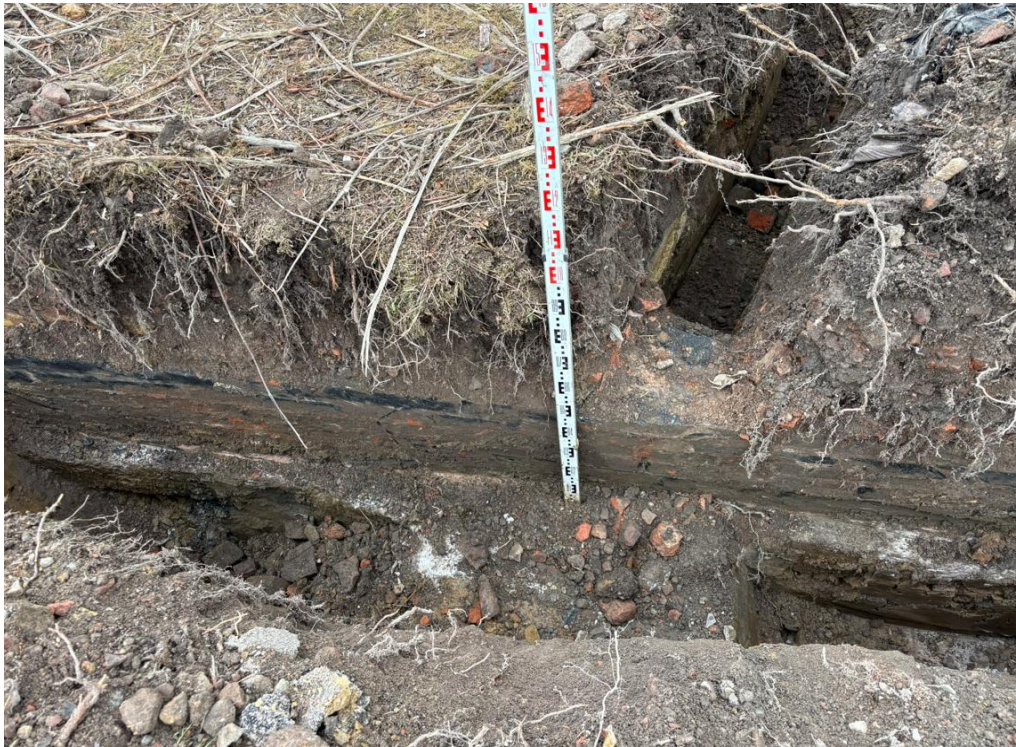
TT01 East - Brick wall and footings
