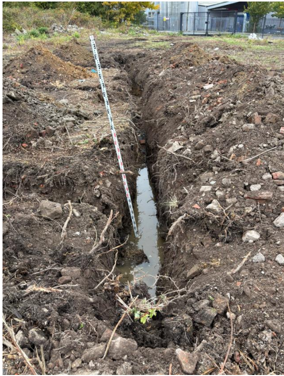
TT01 West - looking east
