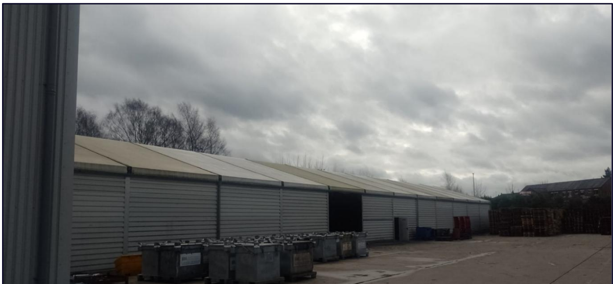
Figure 2: Image of the building in situ
