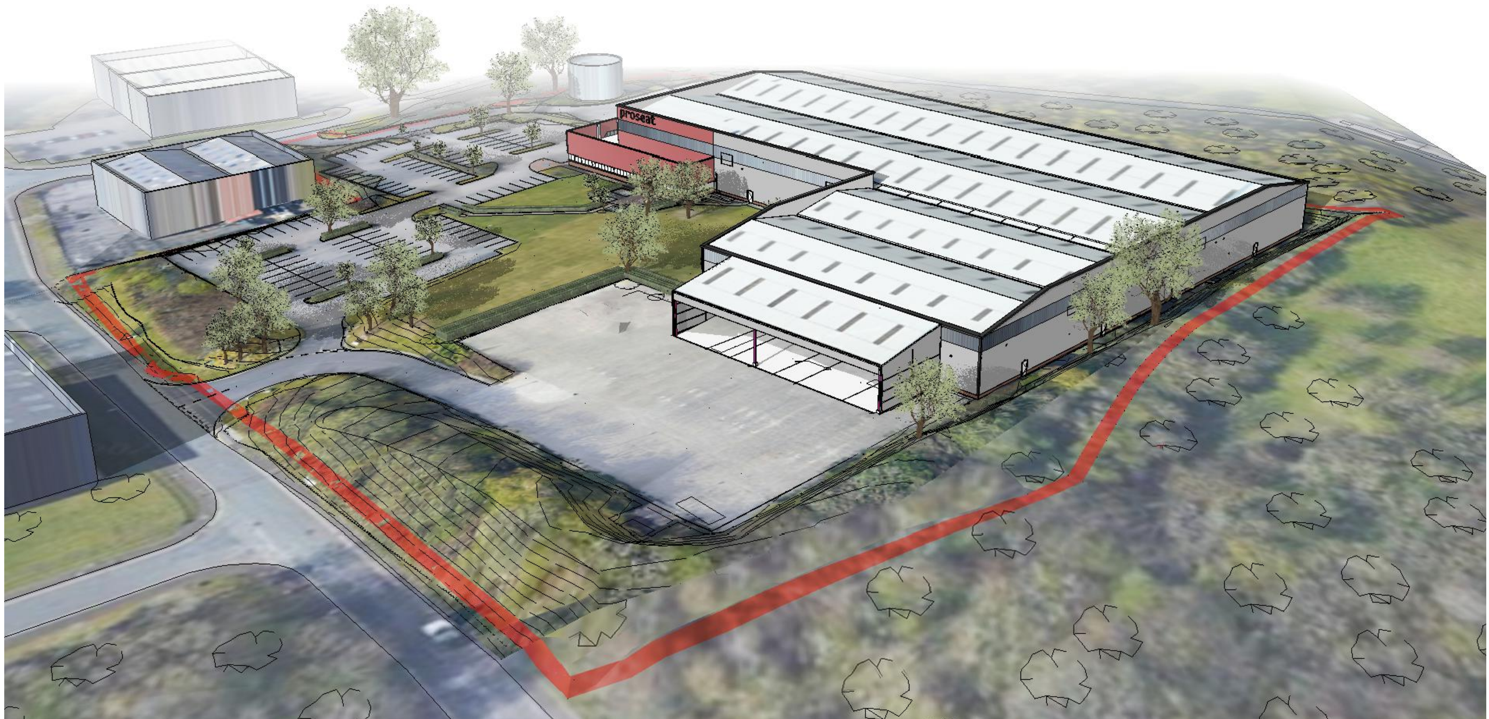
EXISTING AERIAL VIEWS AERIAL IMAGE - C_VIEW OF SERVICE YARD A
