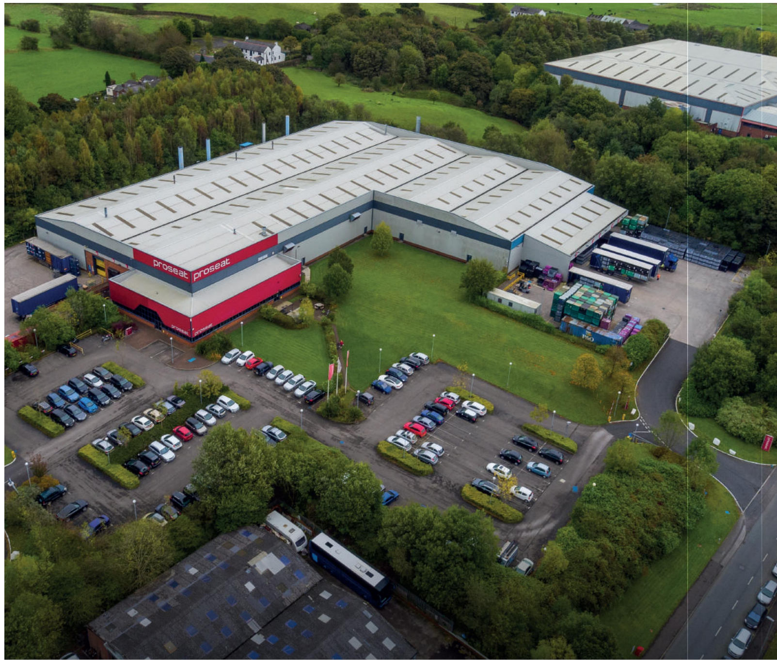
AERIAL PHOTOGRAPH - A_EXISTING ENTRANCE
