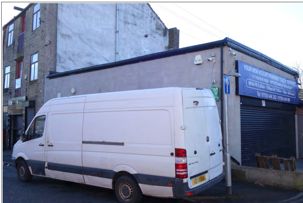
Existing pharmacy building
