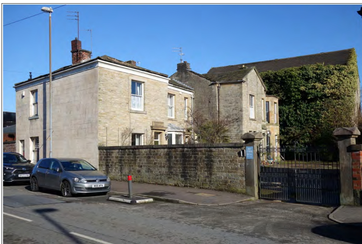
Heybrook House/Flats, with mill to right, from Entwisle Road
