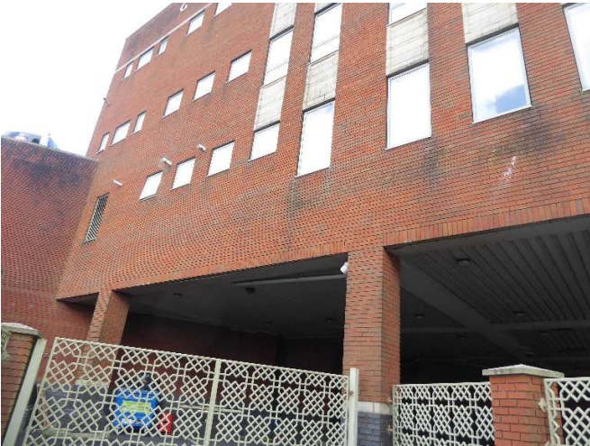
Car port and steel panel underside roof.
