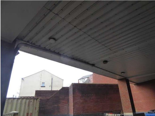
Car port and steel panel underside roof.
