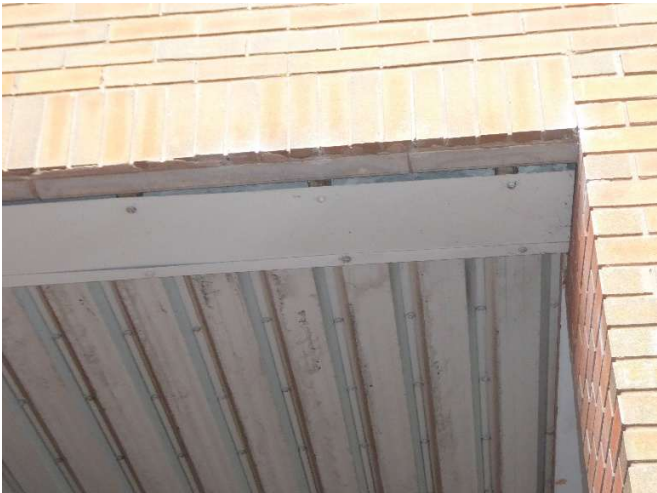
Car port and steel panel underside roof.
