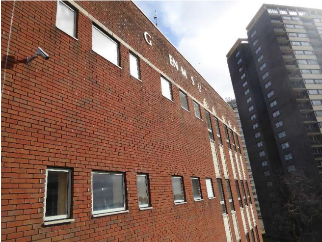
South west elevation location of proposed extension. All brickwork and windows are tightly sealed with no potential points for bat ingress.
