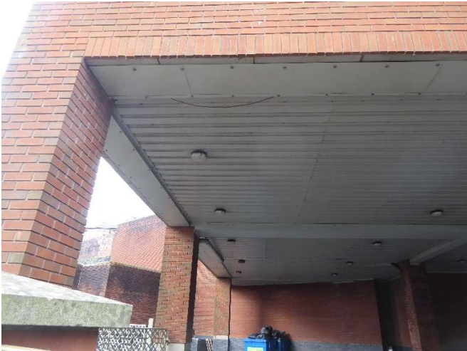
Underside of car port area showing steel panel roof with no suitable points of ingress for bats.
