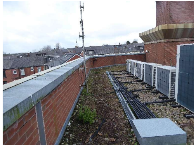
Flat green roof, showing steel panel protective panels over the wall plate.
