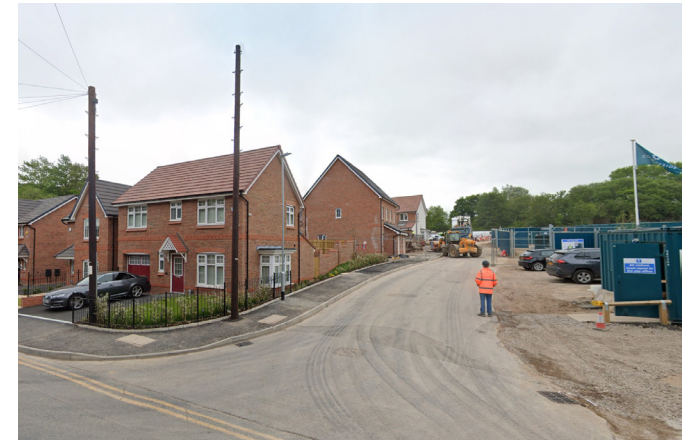
View No. 4 - This is a view further down Royle Road showing the ongoing development of houses.
