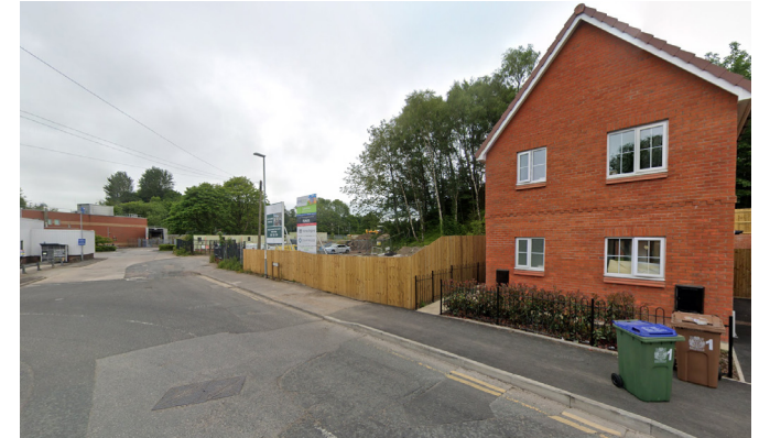
View No. 2 - This is a view from Royle Road towards the site entrance and the proposed extension of Royle Road to create the new access road.
