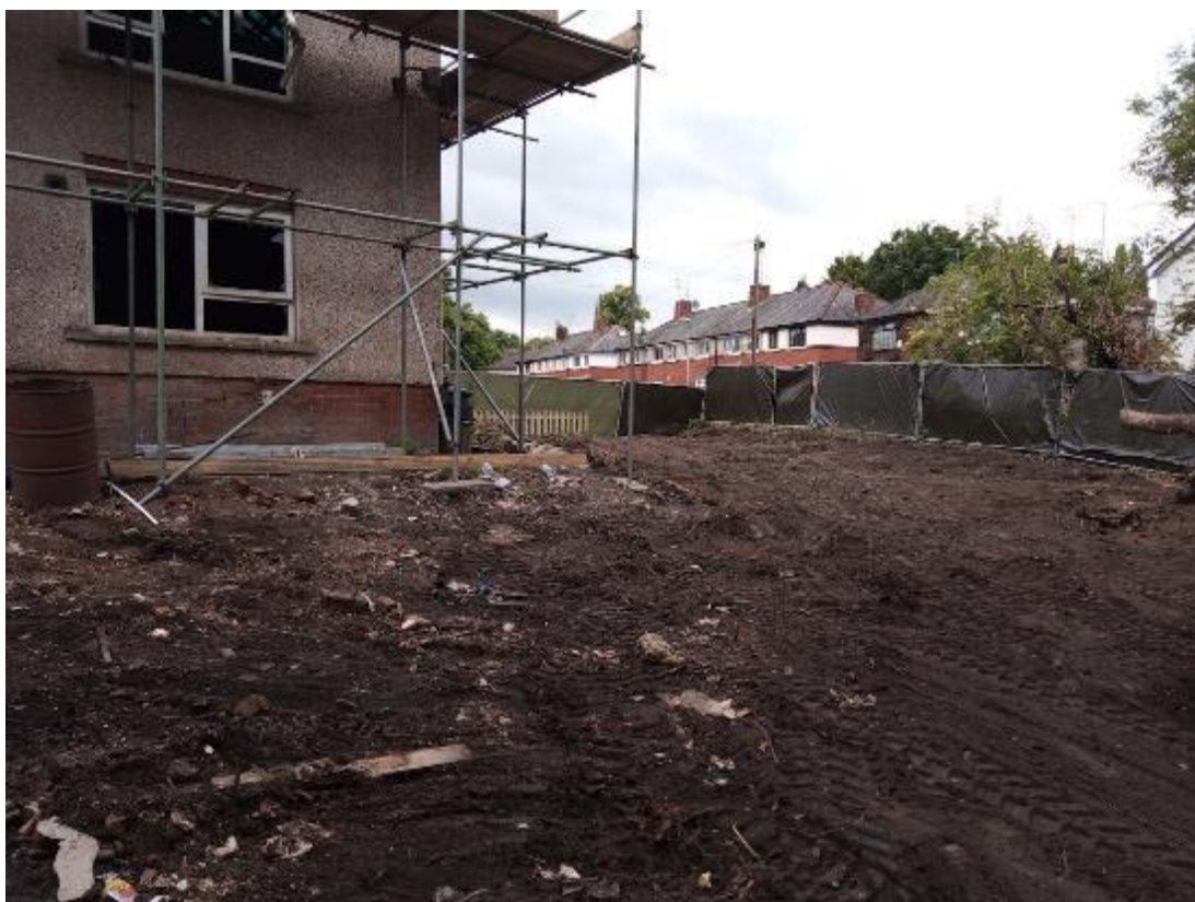
The site (above) after clearance and removal of 3 trees
