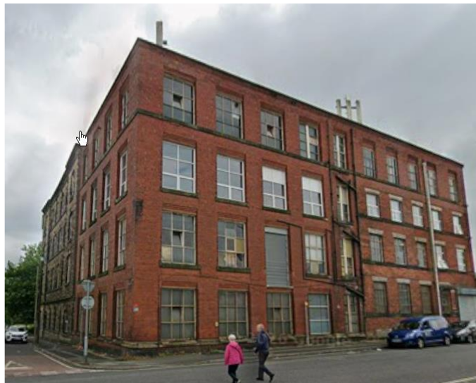
Figure 1 Street view of site
