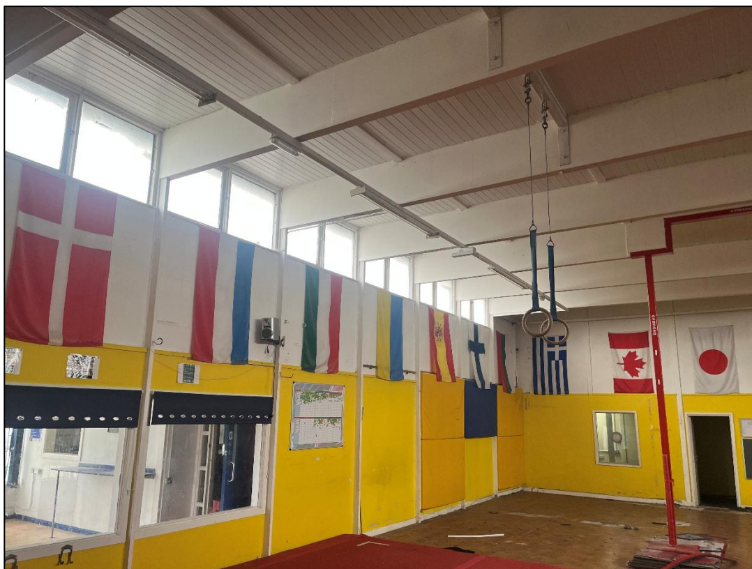
Plate 4 – Internal character of main section of building
