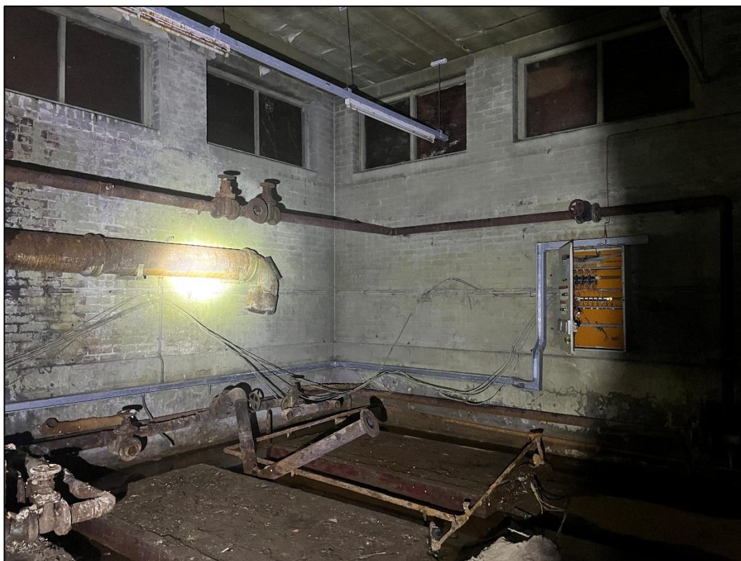
Plate 6 – Internal character of plant room
