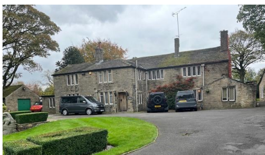
Fig 2.2 North elevation of House (front)
