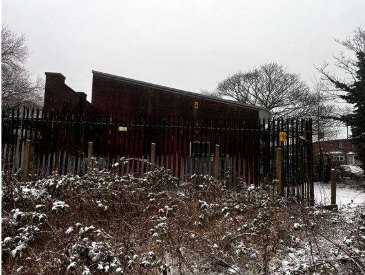
View to the east of the Electrical Substation on adjacent land
