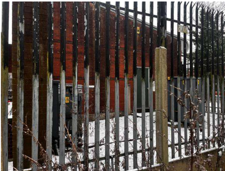
View to the east of the Electrical Substation on adjacent land
