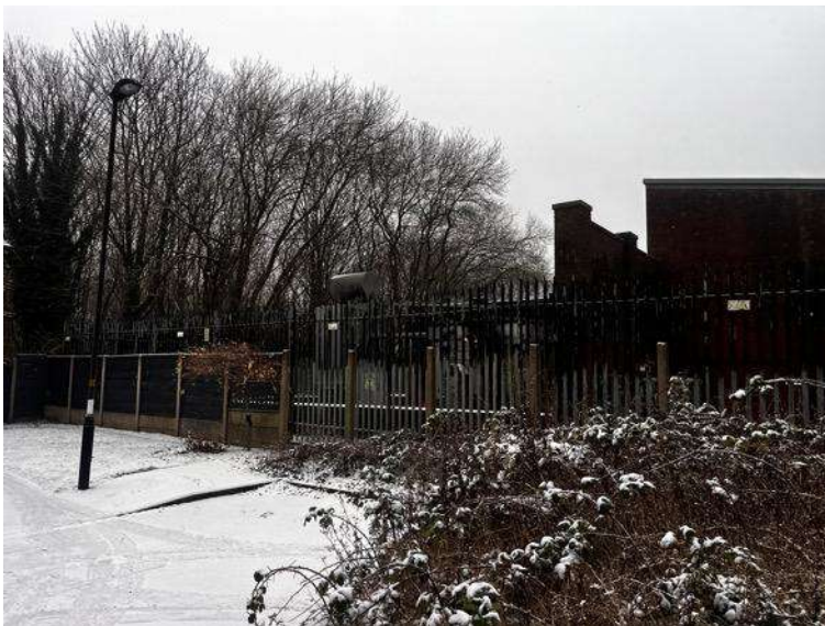
General view to the east showing the Electrical Substation and associated infrastructure immediately adjacent to the site
