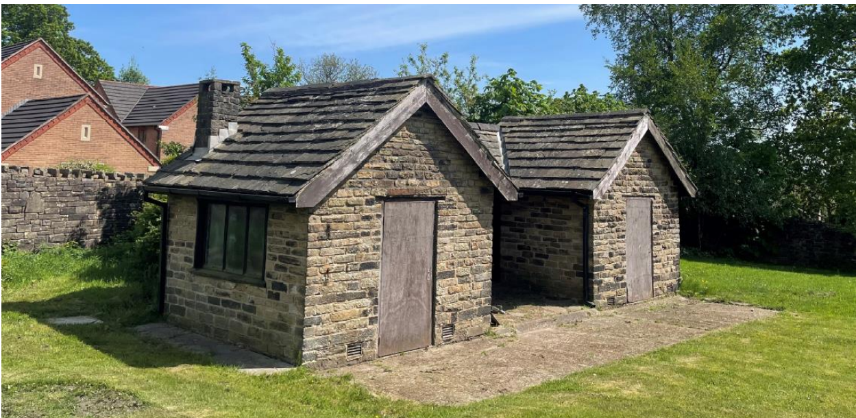
Figure 4: Existing stone Outbuilding and boundary wall
