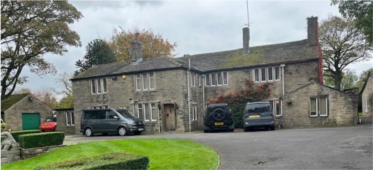
Figure 2: North elevation of Standrings House (front), image courtesy of Heritage Statement document
