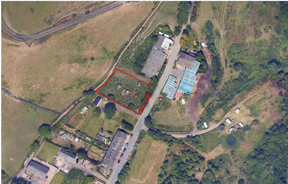
Figure 1.1: Location of Salley Street ( https://earth.google.com/ historical imagery 2023)
