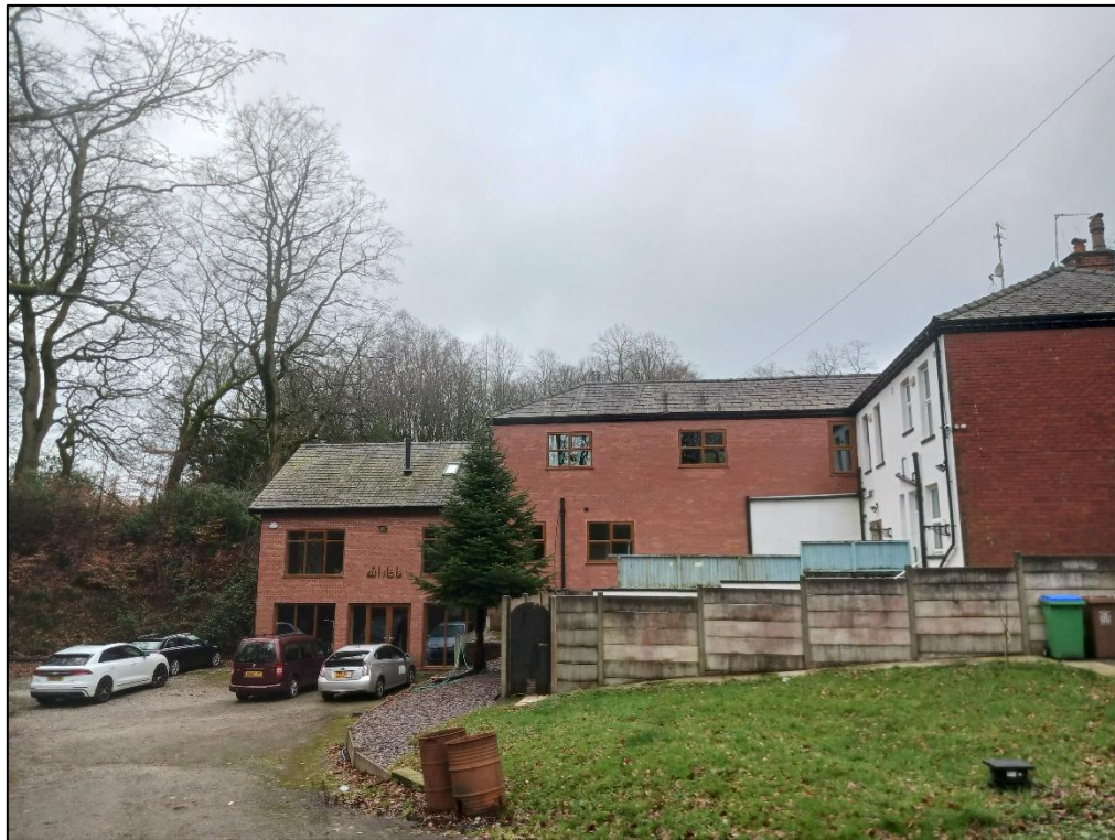
Figure 2.5: View along the driveway towards parking area and Plumpton Cottage extension beyond (note: the rear element has a lower ground floor level).
