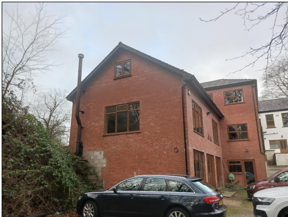
Figure 2.6: View of the rear elevation of Plumpton Cottage.
