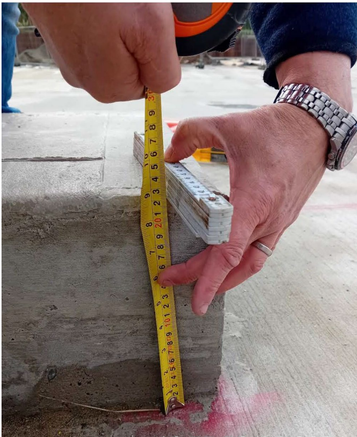
Photograph No.8: Concrete plinth of depth 230mm
