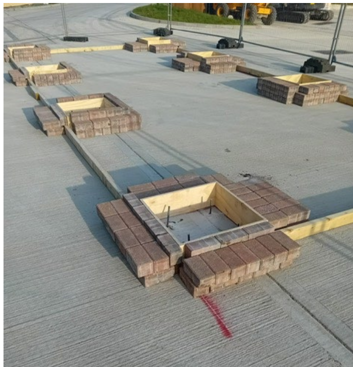
Photograph No.3: Demonstrable thicknesses of concrete pads (c. 2no. brick depths in foreground, 3no. bricks in background) and ground anchors installed.
