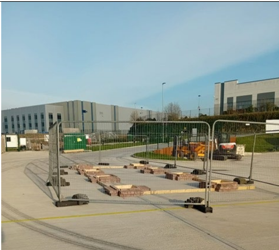
Photograph No.2: Setting out of the 8no. pad foundation locations on existing concrete slab
