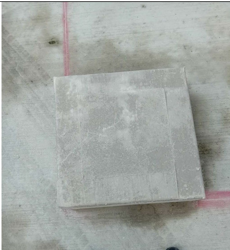
Photograph No.10: Completed concrete pad foundation (plan view)
