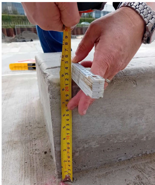
Photograph No.9: Concrete plinth of depth 220mm
