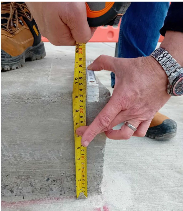
Photograph No.6: Concrete plinth of depth 250mm
