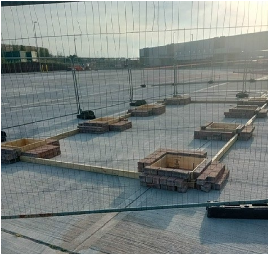
Photograph No.1: Setting out of the 8no. pad foundation locations on existing concrete slab
