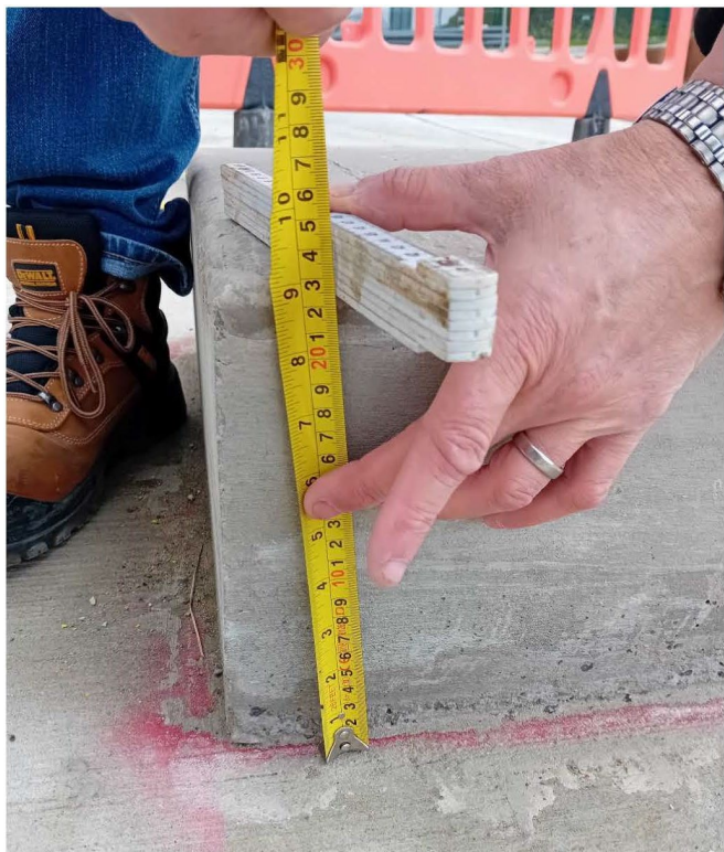
Photograph No.7: Concrete plinth of depth 225mm
