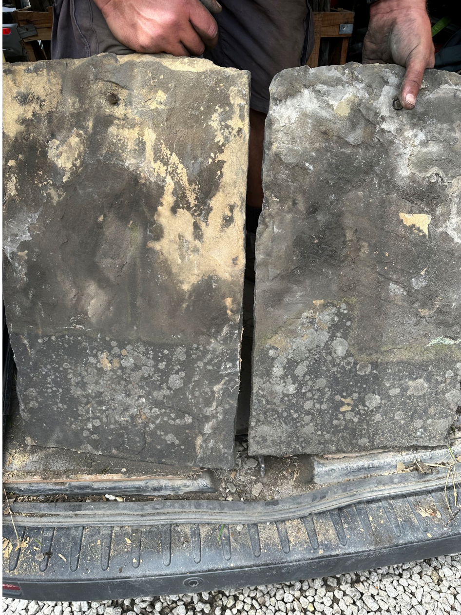
Fig. 1: Reclaimed Riven Sandstone Slate (left) and Existing Sandstone Slate (right).
