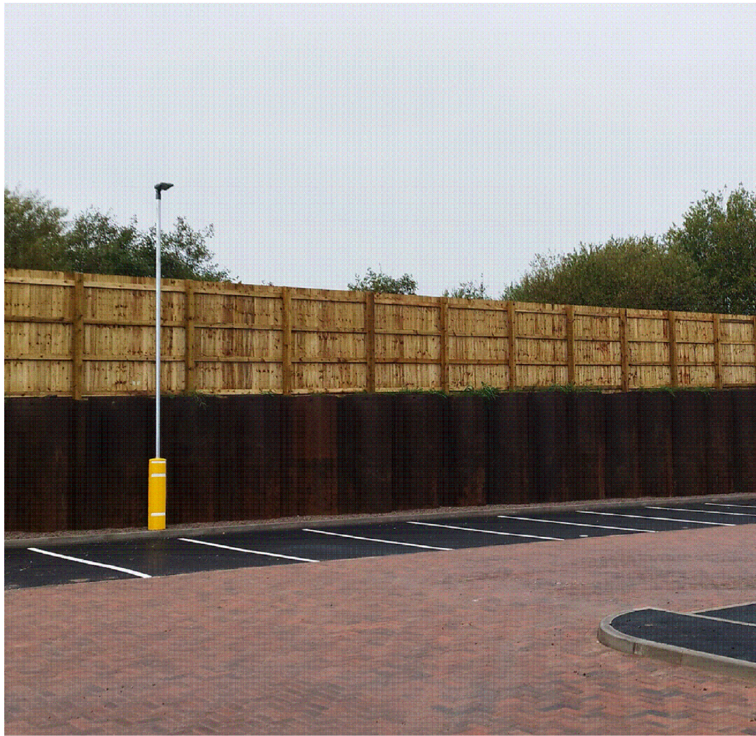
Typical metal sheet plied wall image
