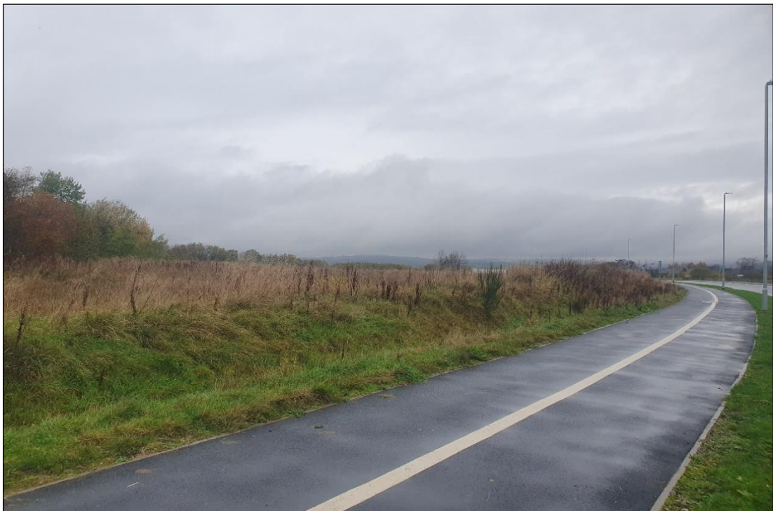
Photograph 2: View Along Pedestrian Path which Runs Alongside North Boundary
