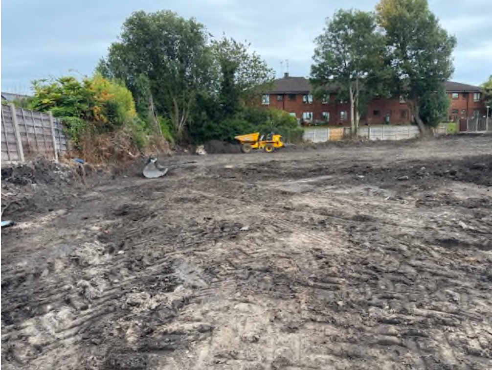
Plot 5s - 8 Gardens: Contaminated topsoil removed, natural subsoil exposed
