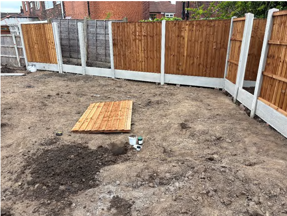
Plot 6 Garden: imported green field topsoil placed in garden
