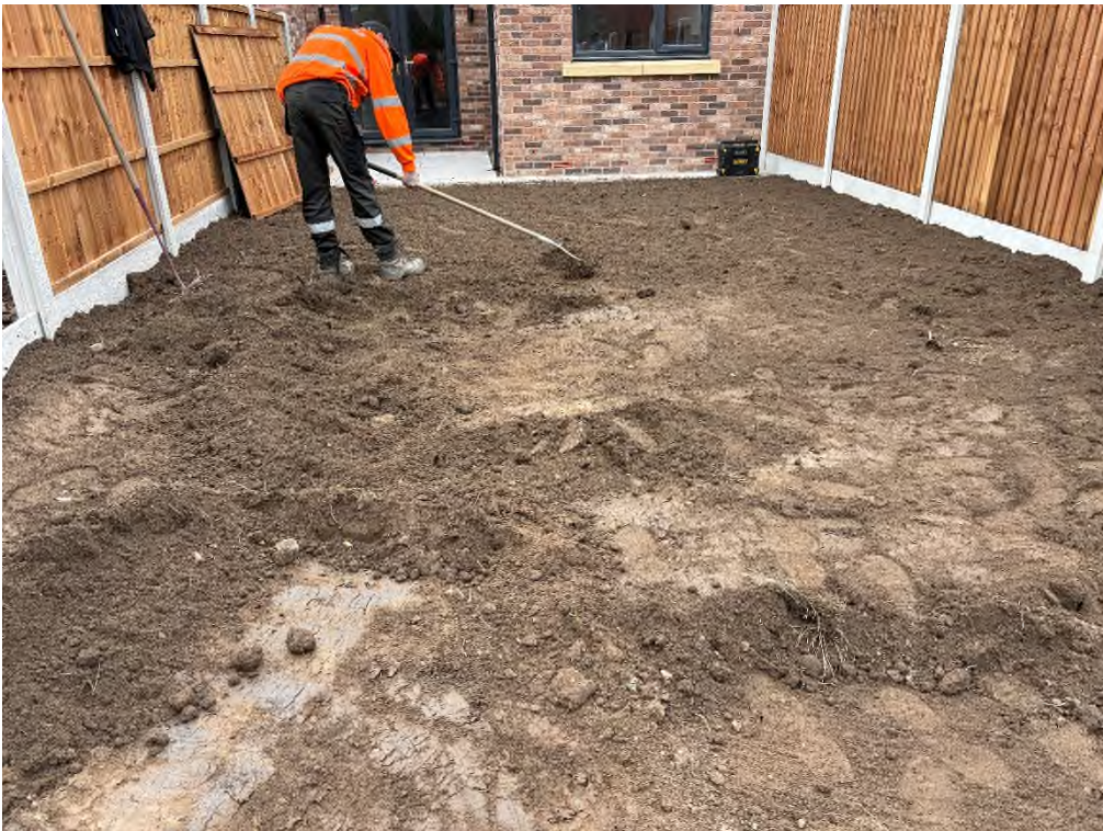
Plot 7 Garden: imported green field topsoil placed in garden
